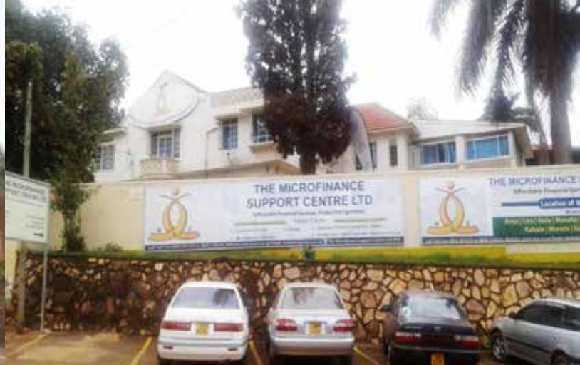
Former MSC Offices on plot 46 Windsor Crescent in Kololo
