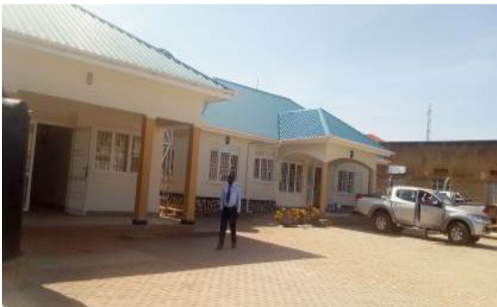
DDA office buildings for Northern region were completed in Gulu District
