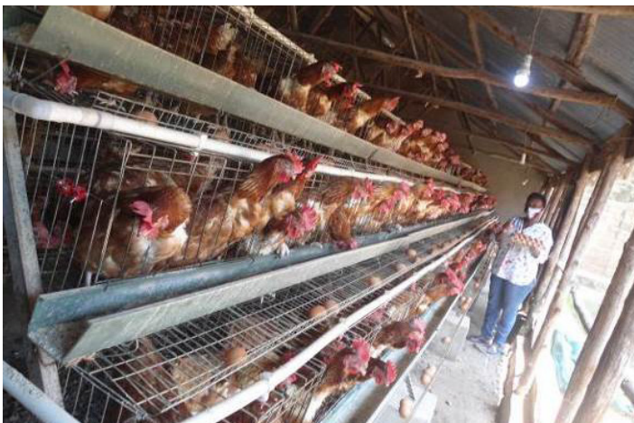
Poultry structure and cages established with ACF at Peri Farmers Limited premises in Kampala District
