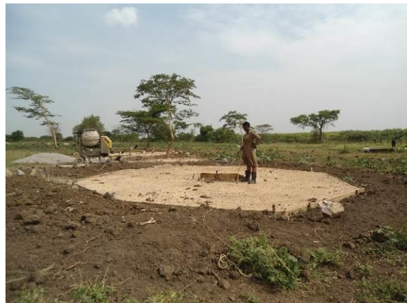
Foundation of water trough constructed at Maruzi Ranch in Apac District
