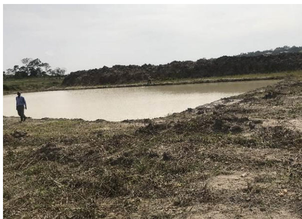
MAAIF excavated community dam with unlevelled soil piles in Buikwe District (left), and valley dam without means of drawing water and troughs in Kaganja village Nakasongola District (right)
