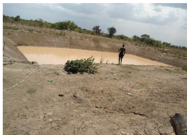
MAAIF excavated community dam with unlevelled soil piles in Buikwe District (left), and valley dam without means of drawing water and troughs in Kaganja village Nakasongola District (right)
