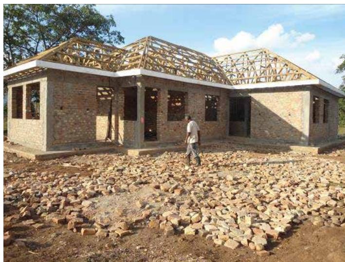
Administration offices under construction at Rubona Stock Farm in Bunyangabo District
