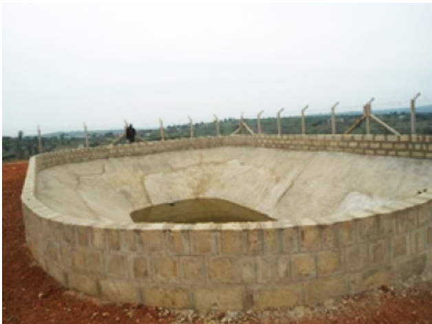
A well cemented water reservoir by MAAIF in Rwamabala village, Lyantonde District
