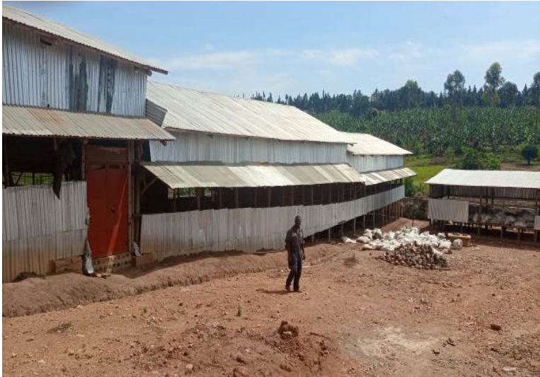
ACF financed poultry house that was constructed at Sako Fish Ltd Farm in Mukono District
