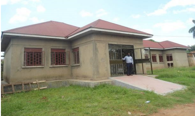
Laboratory constructed including internal walls, ceiling, and flooring, internal and external doors at Jinja District Production Office
