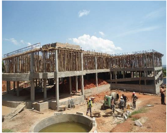
NAGRC&DB Headquarter structures under construction in Entebbe Municipal Council Wakiso District
