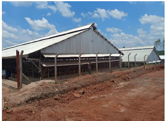
ACF financed poultry houses at Mr. Wambedde's farm in Mukono District
