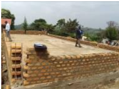
A classroom block under construction at Kibiito S.S.
