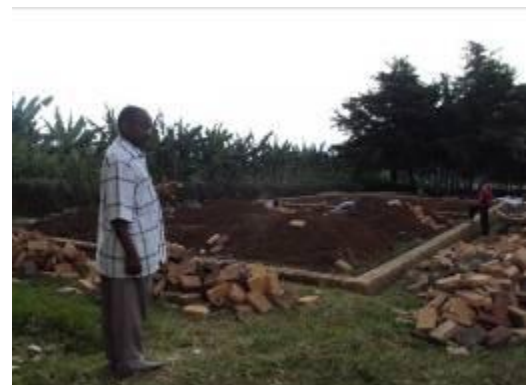
Science Lab. at substructure
