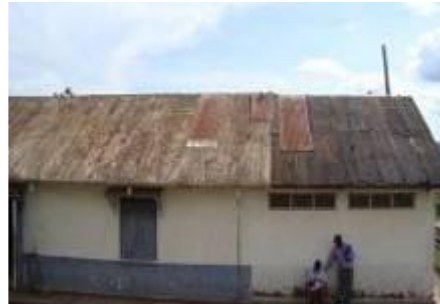
Drug store before rehabilitation
