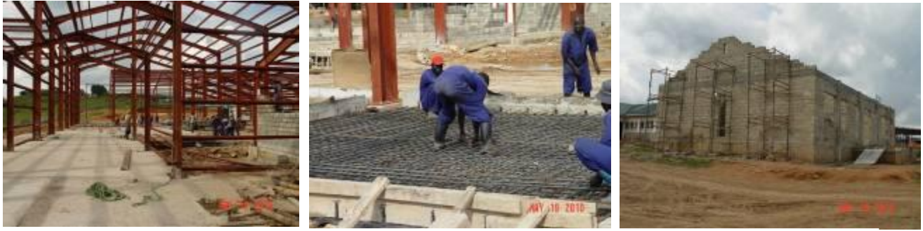
Ongoing Stell works at the main processing plant and administration block
