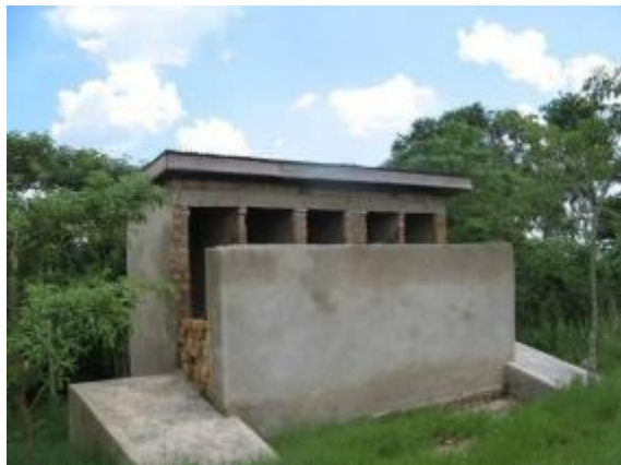
Construction of an ECOSAN facility at Bukalango Prayer Palace in Wakiso district next to a water borne toilet
