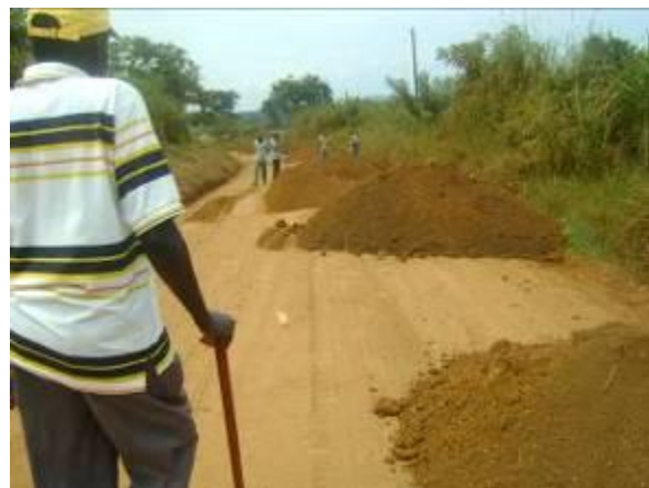
Kiziranjumbi – Kagadi road: a long stretch graveled with less than 50mm thickness as opposed to the 150mm instructed (left) and the wide spacing of gravel heaps placed on a dusty road. Shoddy works evident.
