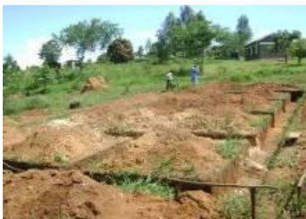
Staff house at Loinya HCII
