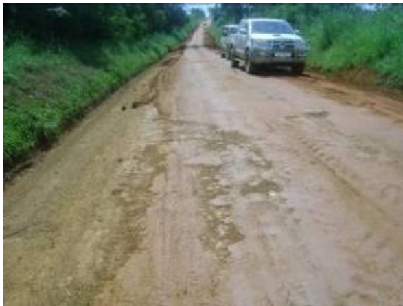
Kiziranjumbi – Kagadi road: a long stretch graveled with less than 50mm thickness as opposed to the 150mm instructed (left) and the wide spacing of gravel heaps placed on a dusty road. Shoddy works evident.
