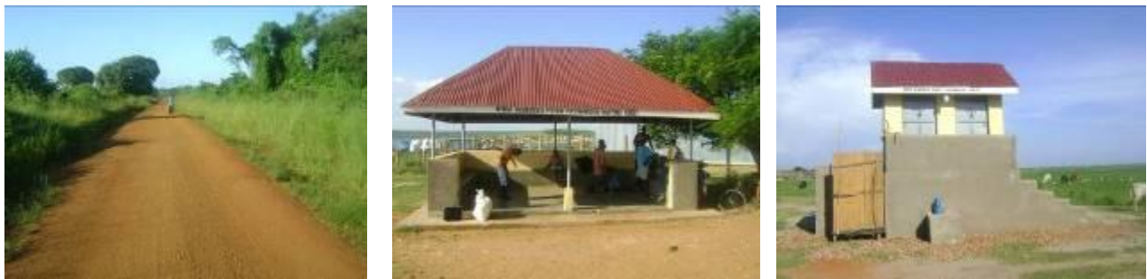
Works done by force account: a section of Rwenkunya – Masindi Port road, still in good condition (Left); Passenger shade and latrine at Wanseko landing site (center and right)
