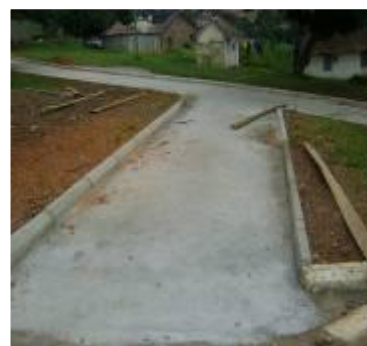
Paved access roads
