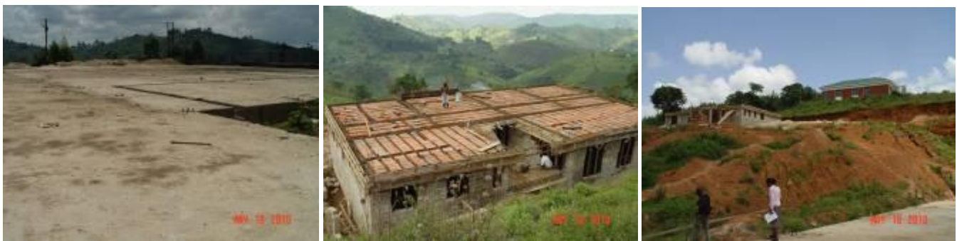
Main plant slab, administration block and kitchen house at Burere-Buhweju
