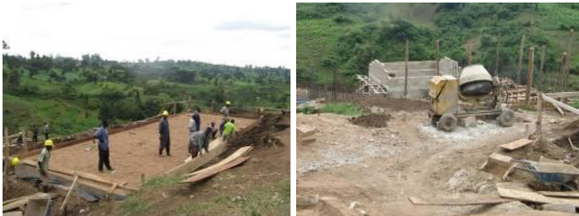
Works ongoing at Tororo - Manafwa gravity flow scheme
