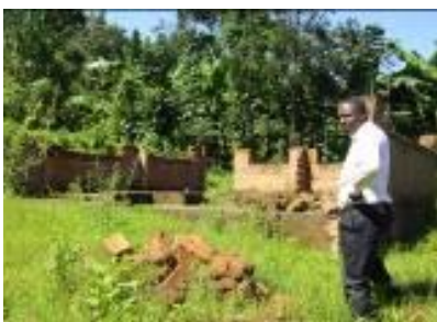
The H/M showing the team the Teachers' house that was left incomplete by the contractor
