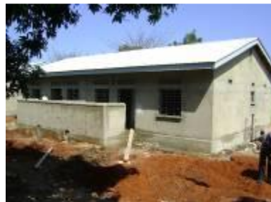
Staff house under construction
