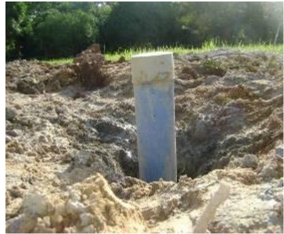
Drilling complete at Nakasongola Prison but pumps need to be installed
