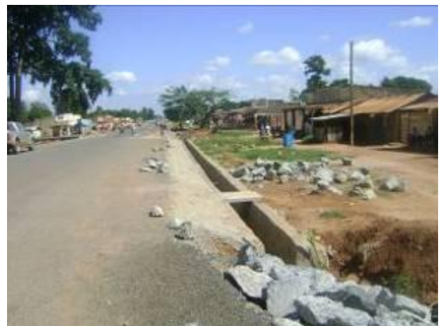
Dokolo – Lira road: Works in progress - 2 nd layer of bituminous surface dressing (left) and stone lining of open drains in Dokolo town (right)
