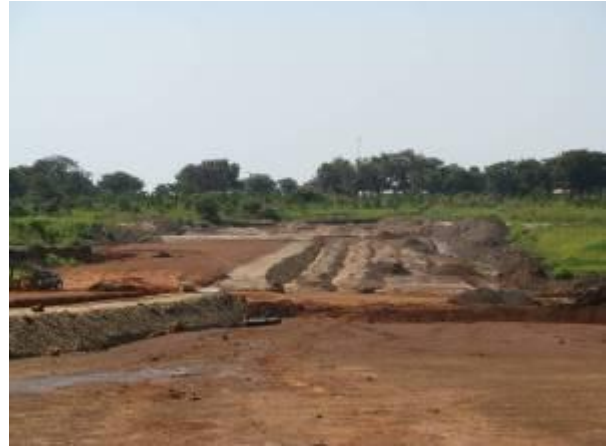
Works ongoing on Akwera dam, Otuke district
