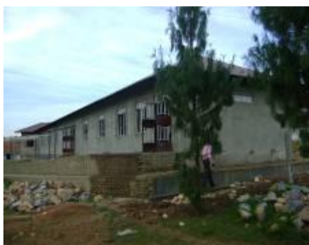
Male TB ward under renovation&
