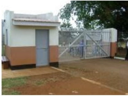
New gate and security house
