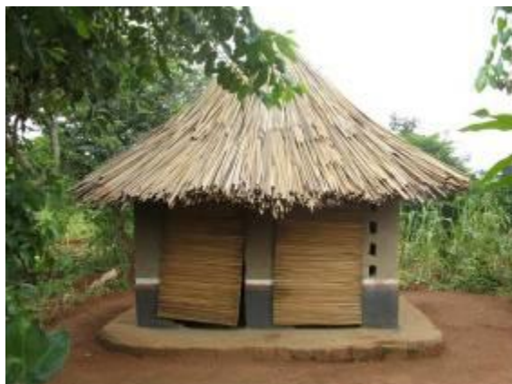
Construction of a pit latrine
