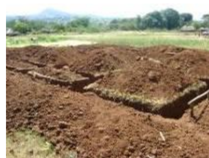
Staff house at Pagwata HCII
