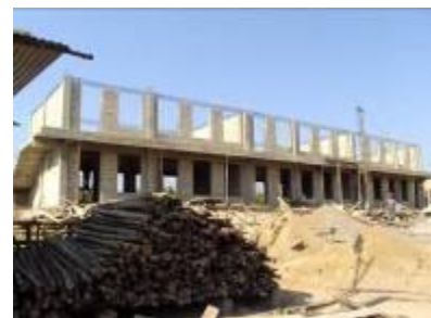
Six classroom storied block
