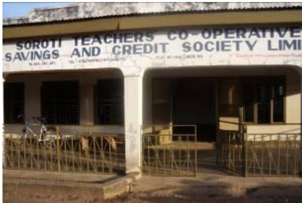
Office premises of Soroti teachers SACCO
