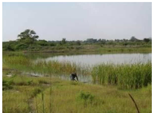
Olamia valley tank in Apac constructed at a unit cost of US$ 34,000 per m 3 . Site is one year delayed and still incomplete; a beneficiary is accessing water directly – a public health risk
