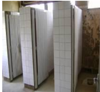
Partially rehabilitated toilets
