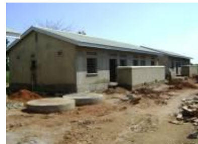
Staff houses under construction
