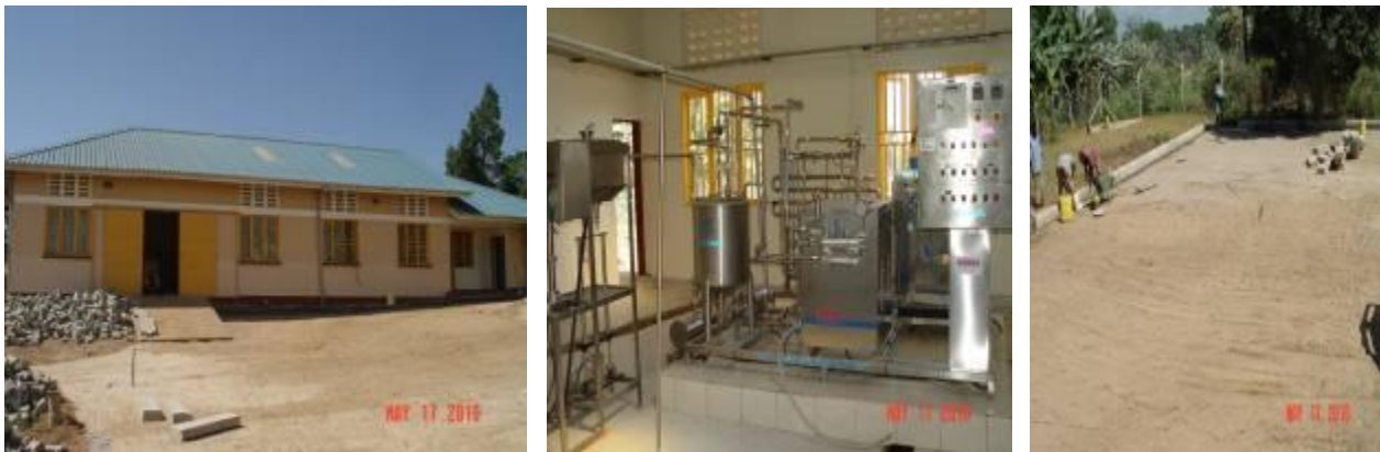
Front view of Nabusanke Fruit Factory plant, installed equipment and ongoing paving
