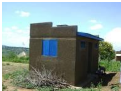
Kitchen at Abong HCII
