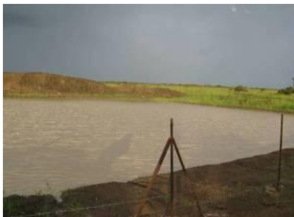
Valley tank constructed in Katakwi at a unit cost of US$ 3,300 per m 3
