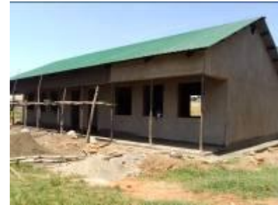
Two classroom block at Palisa
