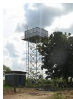
New reservoir complete as planned, Gulu Youth Centre. Gulu district
