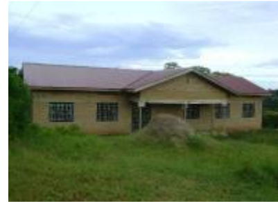
Stalled General ward, Kiganda HCIV
