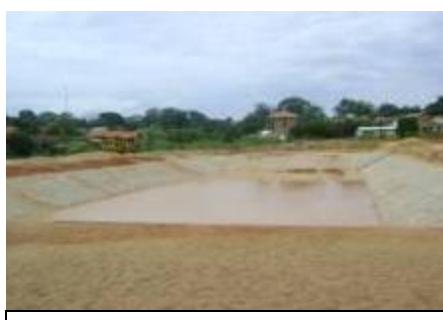
Lagoon under construction
