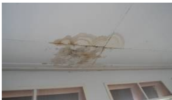
Left: Ceiling works at Pallisa Hospital
