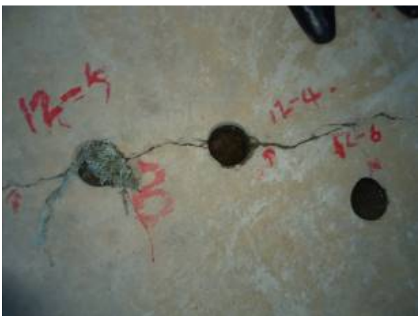
L-R: Some of the observed cracks at the Spillway section and Civil works at Karuma HPP
