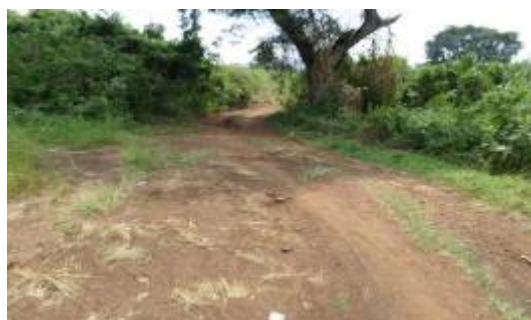
Part of Munteme–Kajoga-Bubogo road along which only bush clearing was done
