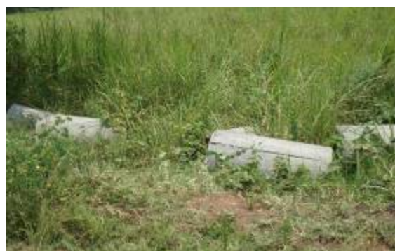
Culverts along Namunkanga–Nabutaka road yet to be installed
