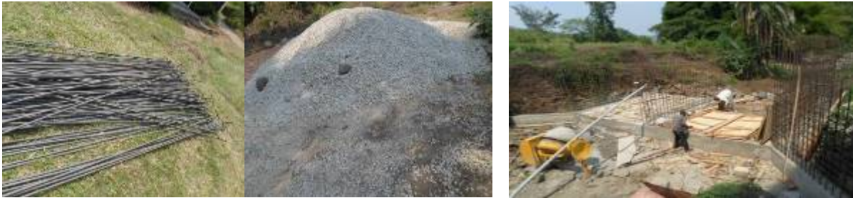
Some of the materials mobilised for the construction works
