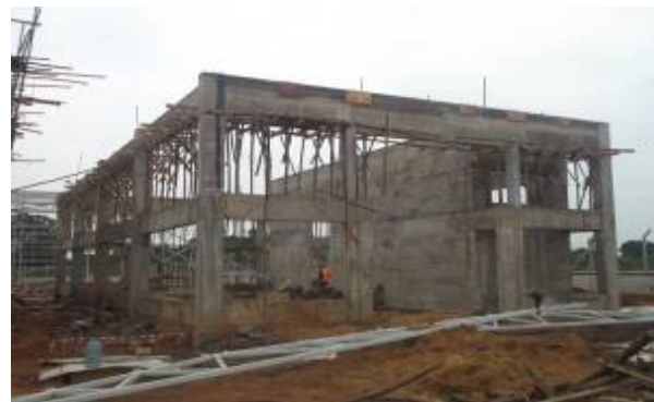
L-R: Ongoing casting of the slab on the two underground water harvesting tanks and a completed super structure of the power house at the UCDO seed dressing station in Pader district
