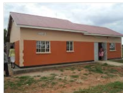
Completed Omatenga Health Centre II in Kumi District
