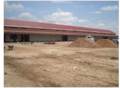
Left: Completed stores in Namalu Prisons, Nakapiripit District
