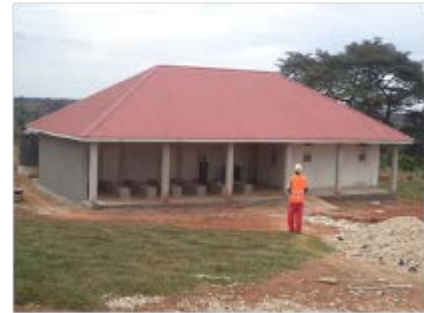
Incomplete Nalutuntu Health centre in Mubende District
