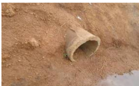
Installed culvert line along Kiraka-Katuugo with no end structures A well graded section along Kiraka-Katuugo road
