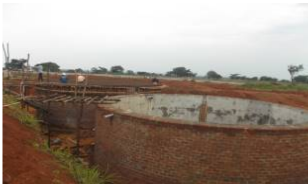
L-R: Ongoing casting of the slab on the two underground water harvesting tanks and a completed super structure of the power house at the UCDO seed dressing station in Pader district
