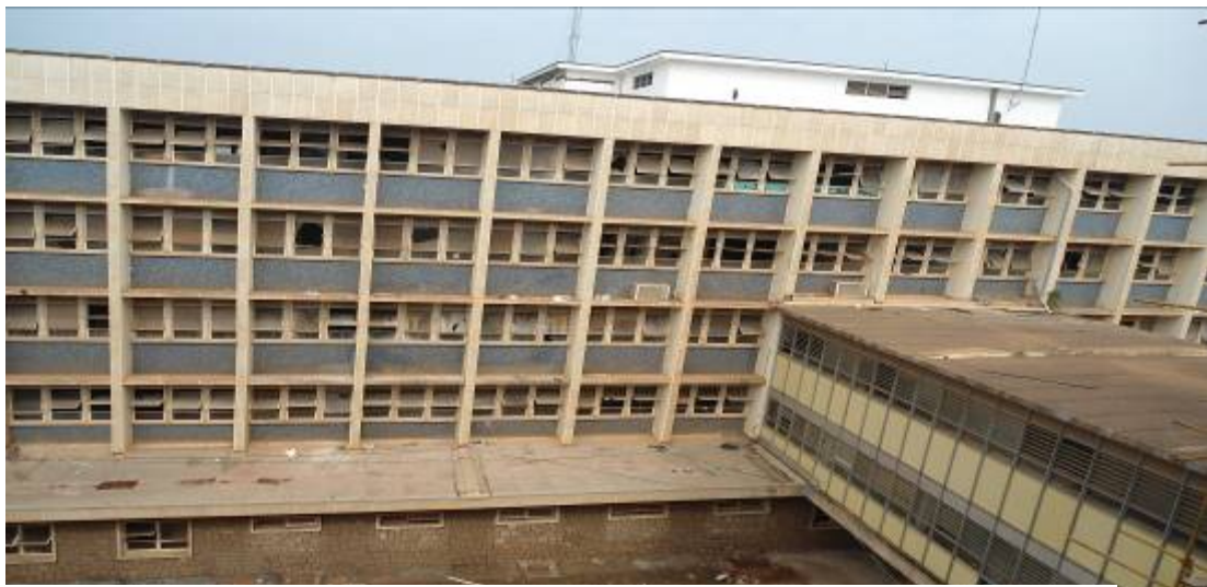
Some of the incomplete works at Mulago National Referral Hospital
