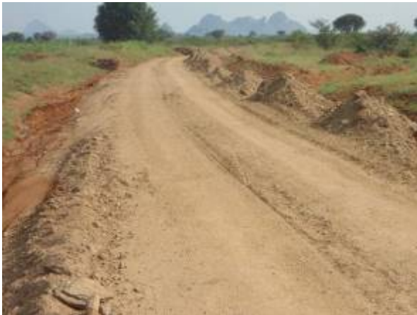
Dumped dead rock for graveling at km 9+500 from Kopoth along Kopoth-Kabong road Graded section along Kanawat-Kopoth road
