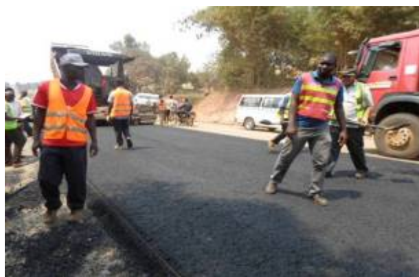
Laying Asphalt along Nansana–Busunju road in progress
