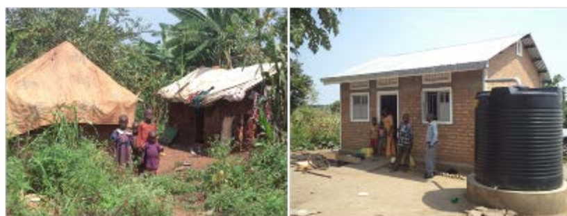
Left: Previous house of Beneficiary Hatiya John; Right: Newly completed house for Widow Bukosera Margaret handed over by Habitat for Humanity in Zone B2, Panyadoli, and Kiryandongo District
