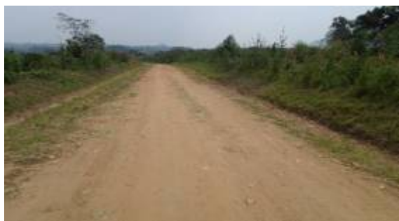
Graded section along Kyomera–Ihindiroyabukumba road
