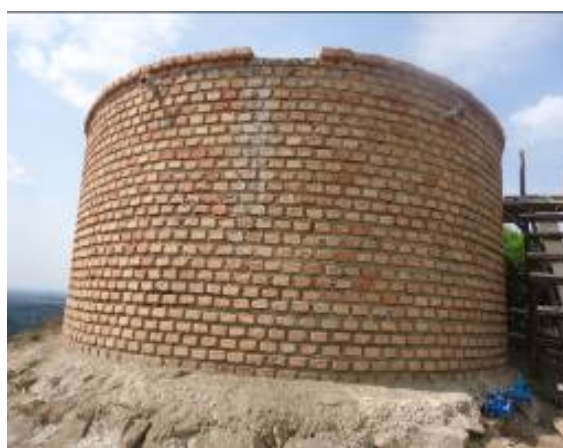
L-R: A spring in Nwoya district and 75m 3 reservoir tank at Kabingo GFS, Ibanda district
