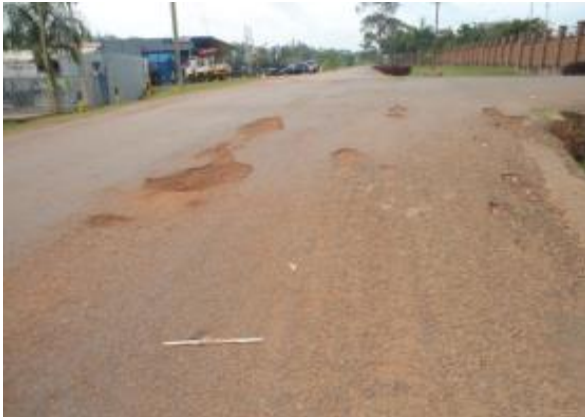
Potholed surface dressed roads in Luzira and Bweyogerere Industrial Parks
