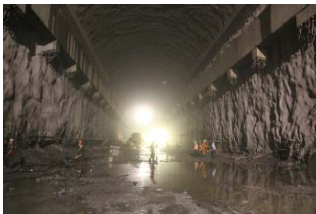
L-R: Civil works at bench III of Power House
