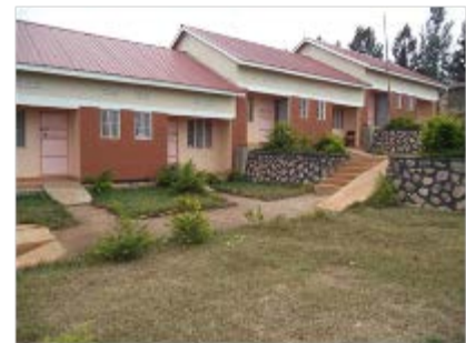
Ruhiira Medical staff quarters constructed in Isingiro district
