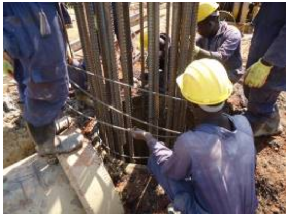
L-R: Excavations and steelworks of special tower (Pile) foundations in swampy sections of Buwama in Mpigi district of the Kawanda–Masaka Transmission Line
