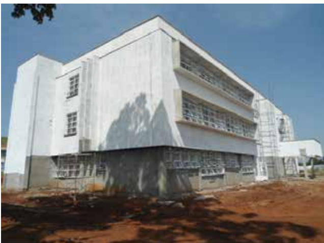
The library at 85% progress at Busitema University by June 2017
