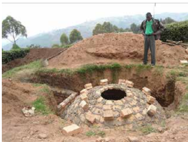
Biogas plant still under construction at Kachwekano ZARDI, Rubanda district
