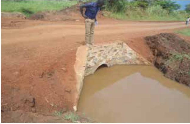
A culvert installed at Km 33+400 along Muyembe- Namalu Road
