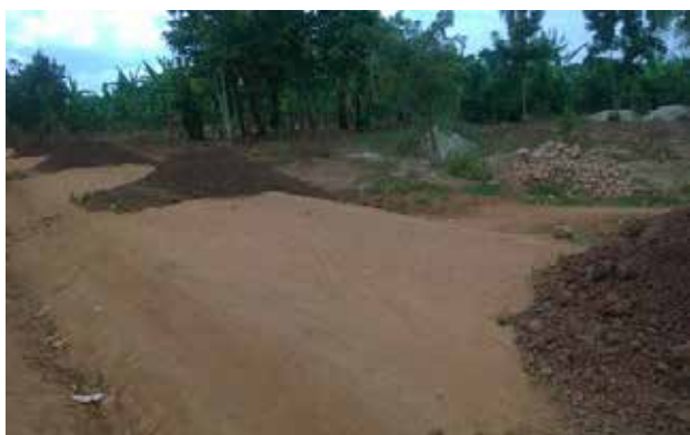
Dumping of gravel ongoing along Banda - Buzibazi Road – Mityana District
