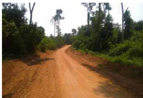
Graded section of Kalandazi – Buwungu Road – Mpigi District
