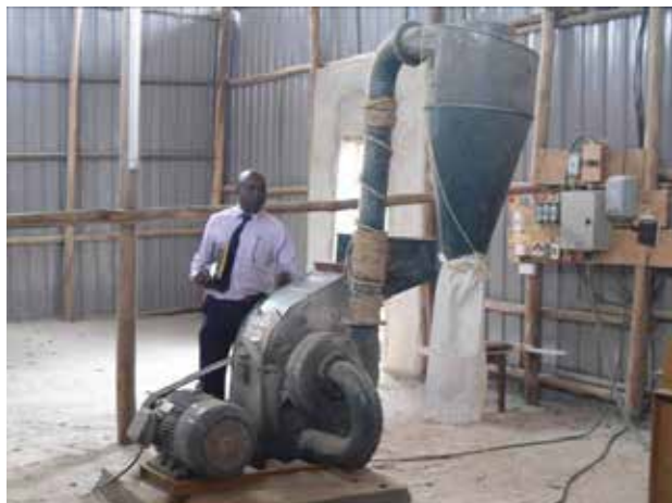
Project feed milling machine installed at Mbarara ZARDI, Mbarara district
