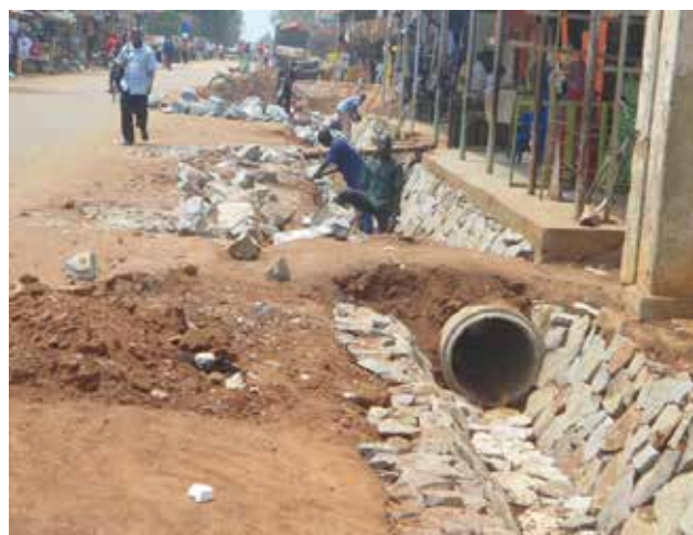
Ongoing stone pitching at Old market Street Road
