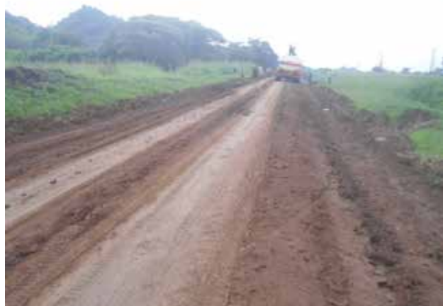
On-going works along Angatun Chosan Road under Term maintenance
