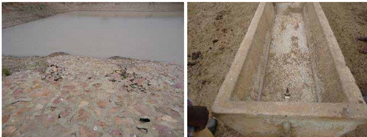
L-R: Butugo Valley Tank; Watering Troughs at Lutunku valley tank, Lutunku A village, Lugusulu sub-county, Sembabule District
