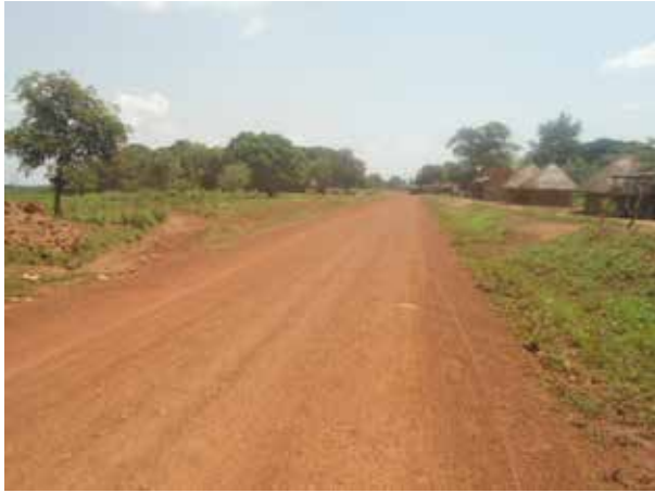
A gravelled section along Arapai-Lira Junction Road
