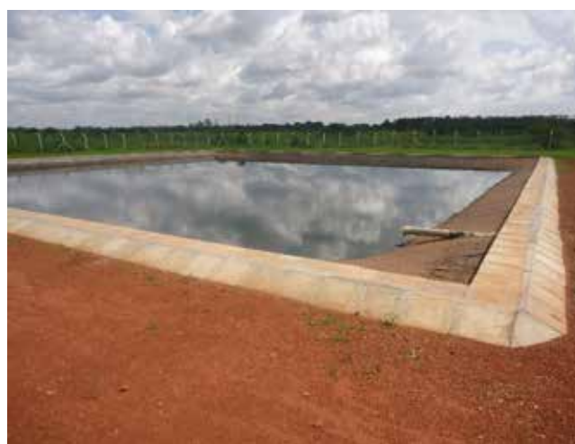
L-R: Fecal sludge receiving chamber and maturation pond in Kayunga District
