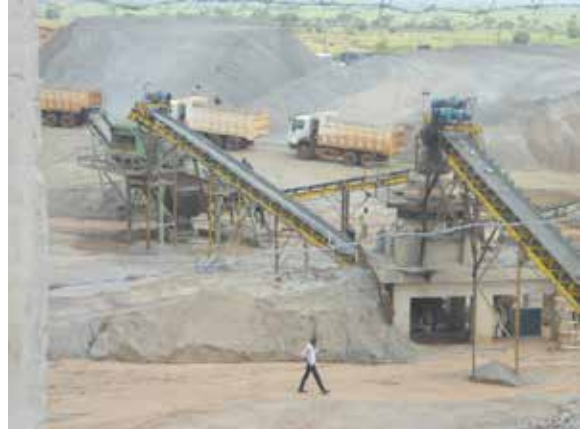
Stock pile crushed stone at the quarry for Akisim-Moroto road project
