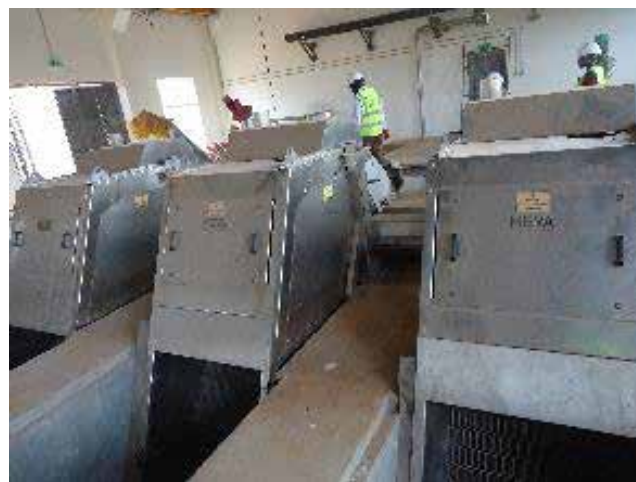
L-R: Anaerobic sludge digester; and Coarse screens at NWWTP Bugolobi, Kampala
