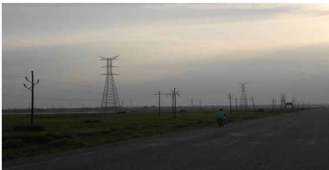
L-R: Completed towers at Awoja swamp on the Lira-Opuyo-Tororo Transmission line
