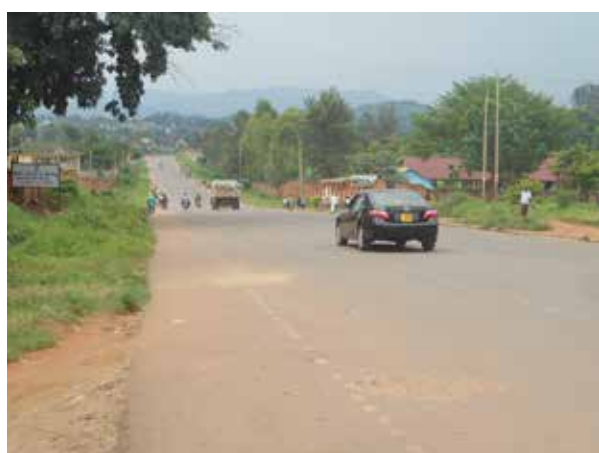
A section of Nabuyonga Rise intervened using the USMID project funds
