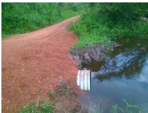
Incomplete Installed culverts along Mugereka – Bumbiri Road- Kyankwanzi District
