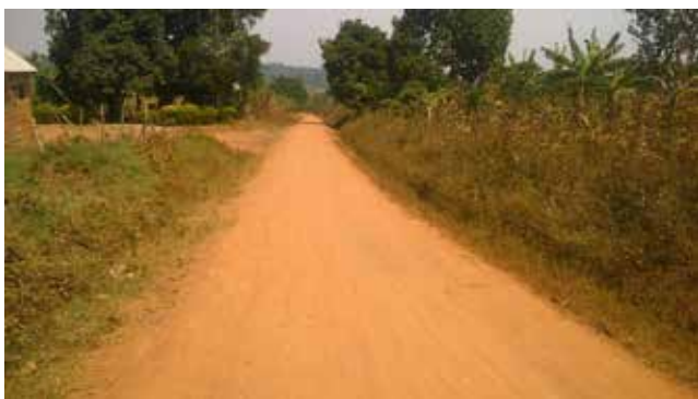
Completed Bukaana–Ntete Road in Sembabule District
