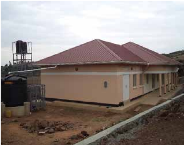
Newly constructed Kihiki HC II in Isingiro District
