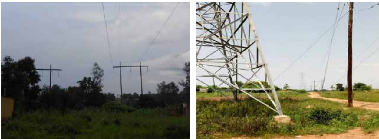
L-R: Section of Lira-Opuyo transmission line at Angwet Angwet, 3km from Lira substation where the old line is being relocated to make way for the new line due to failure to obtain RoW; Towers near Soroti Flying School that have to be dismantled due to objection by CAA because of safety concerns
