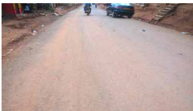
Kabumba Road where single seal surface dressing was applied
