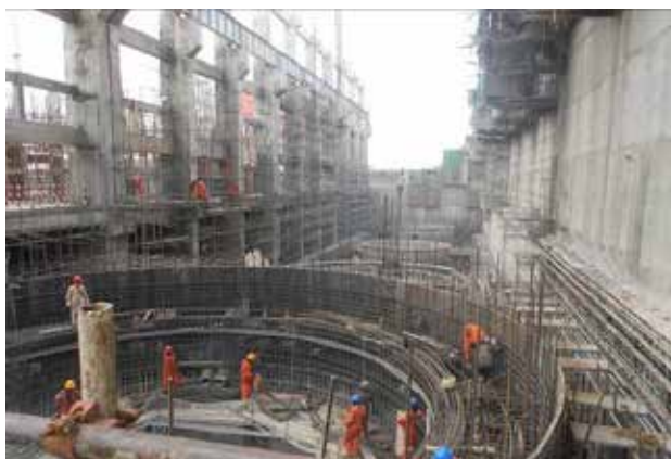
L-R: Installation of rebar in the generator foundations in the power house of Isimba HPP; civil works at the spillway of Isimba HPP
