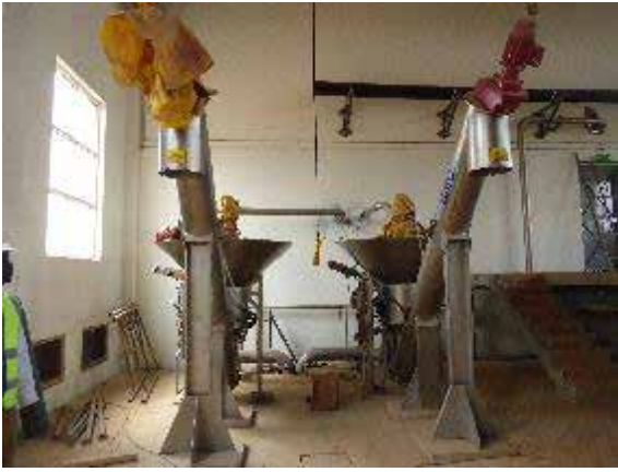
L-R: Grit washer; Sludge thickening and watering building at the NWWTP in Bugolobi, Kampala district
