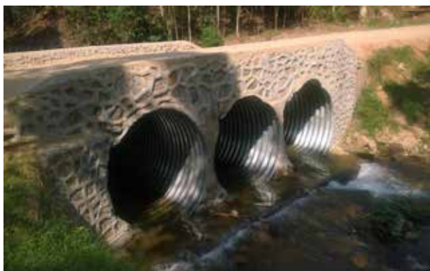
Three cell Amrco culvert bridge implemented using force account – Kasese station
