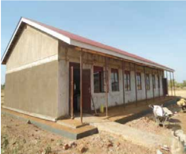
A science block completed at Patong S.S
