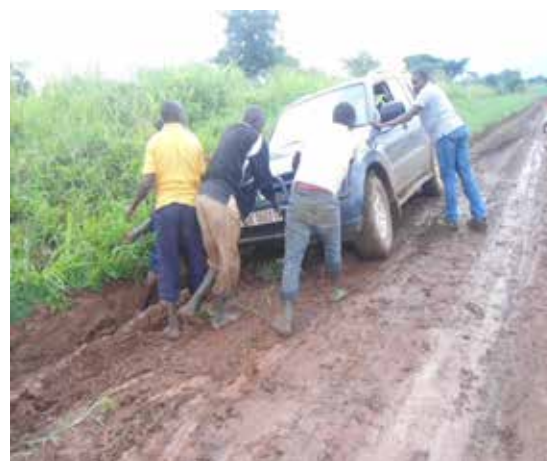
Slippery section along Minakulu-Zambia Road
