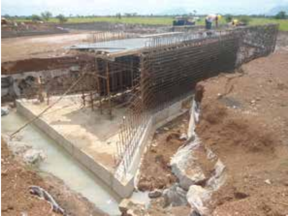
Box culvert works ongoing along Soroti-Akisim road
