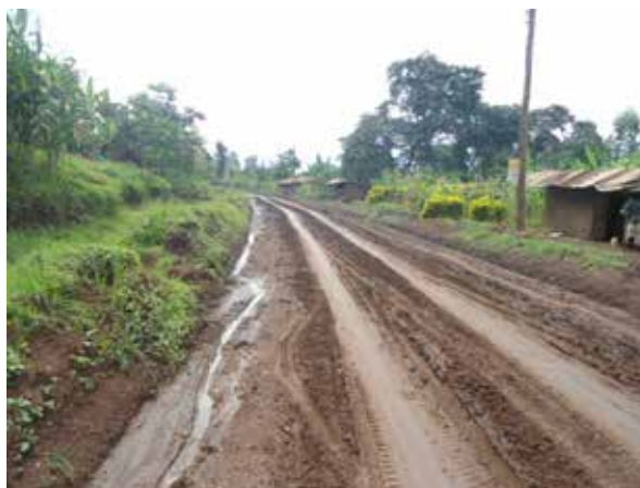
A section of Namagumba Budadiri Road at Km 6+900
