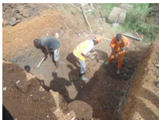
Excavation works for culvert installation at km 11+100 along Amuria-Acowa-Usuk Road
