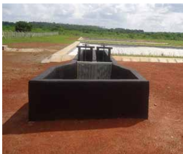
L-R: Fecal sludge receiving chamber and maturation pond in Kayunga District
