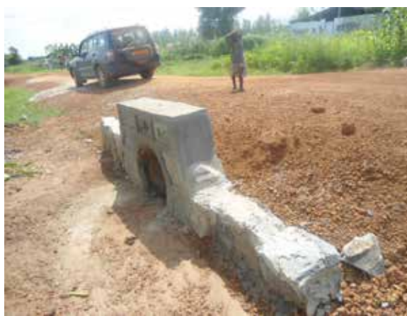
A culvert installed along Teso Road
