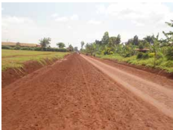
A widened section of Budadiri –Nalugugu Road
