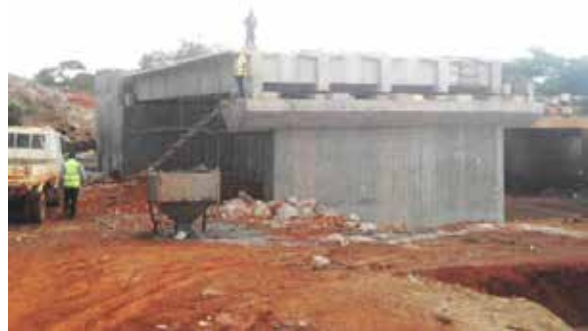
Ongoing deck works for the bridge along Gulu-Acholibur road at Km 127+900
