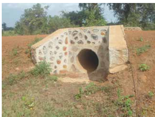
A culvert installed at Km 9+400 along Amuria-Acowa-Usuk Road
