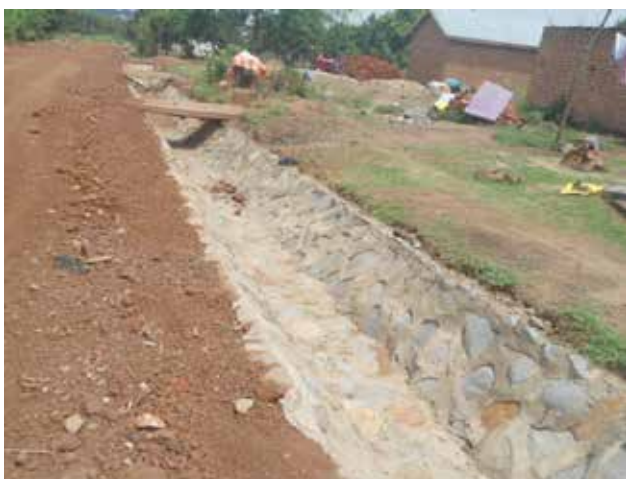
A stone pitched side drain along Barak Road
