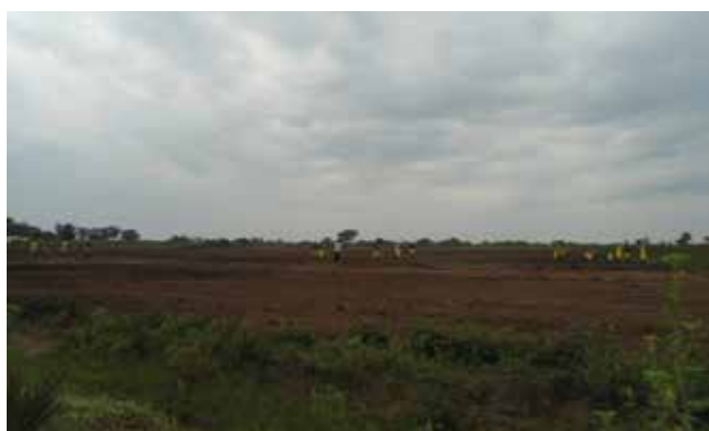
Prisoners planting passparum grass in the temporary ground that had just been levelled at Akii Bua Stadium –Lira District
