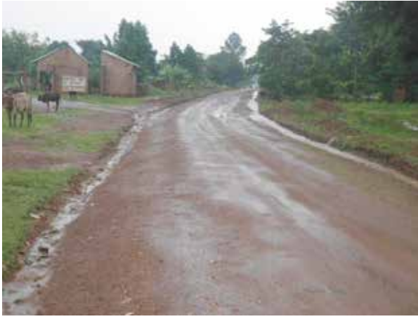
A well gravelled section of Kalamira-Kagulu-Izimba Road at km 0+000
