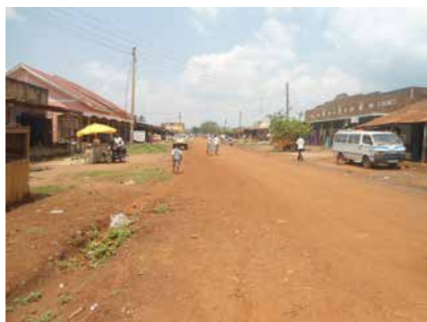
A section of Busoga Avenue that was graded and gravelled
