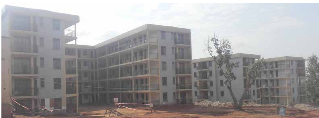
Mulago staff houses at substantial completion
