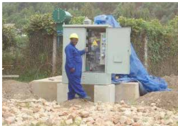
L-R: Boiler and power control panels under installation at Kigezi Highland Tea Factory in Kabale District
