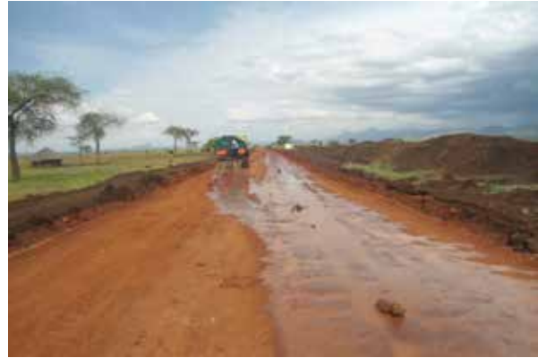
Gravelling works on Chepsikunya-Girik Road
