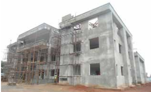
Faculty of Agriculture Block at 76.7% progress by June 2017 – Gulu University
