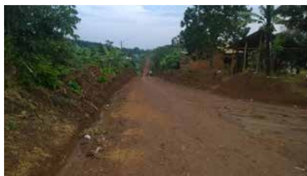
Graded Kudus Road whose works were completed in Quarter one FY2017/18
