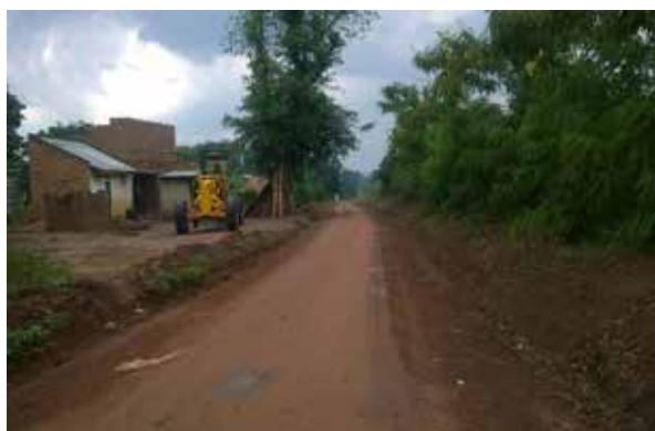
Graded section of Namusaale – Lusanja Road
