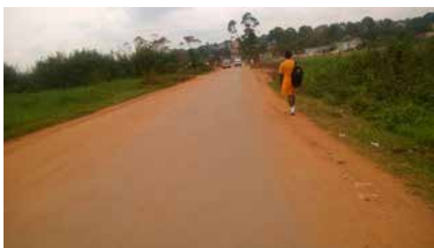
Naluuma Road where second seal surface dressing was applied
