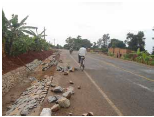
Completed section of Iganga-Kaliro road with stone pitching on works ongoing
