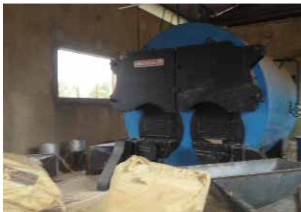
L-R: Boiler and power control panels under installation at Kigezi Highland Tea Factory in Kabale District
