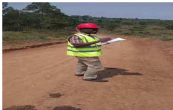
Graded section of Kabandebe–Kyabwamba–Kyebugotoko Road – Sembabule District
