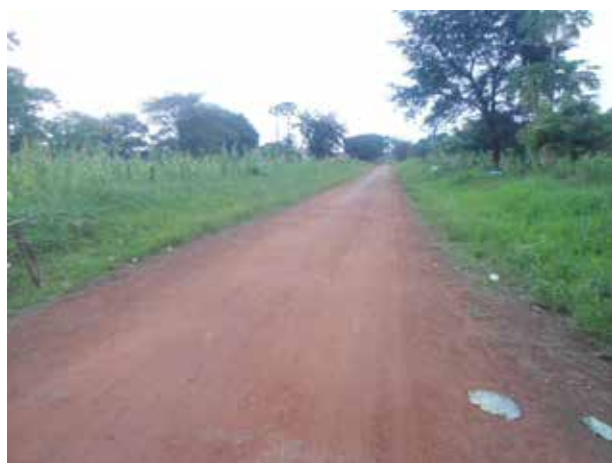
A section of Zambia-Kamdini Road which was in a fair condition
