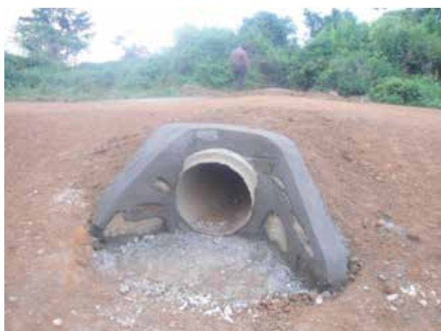
Ochero-Bugoi Road (13.1 km): A culvert installed at km 1+000; A raised swamp section
