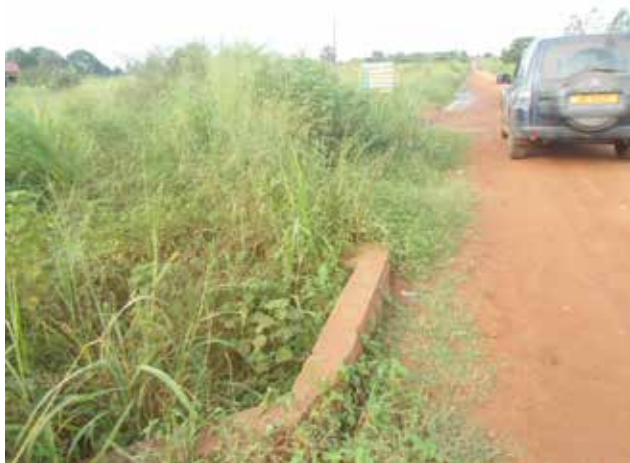
A bushy culvert along Oryang Ojuma Kitgum Matidi Road
