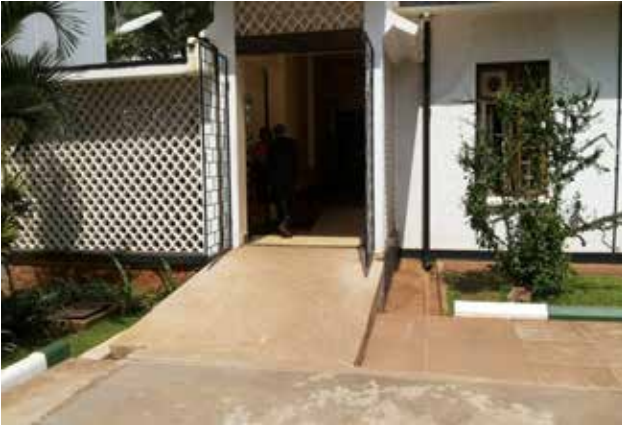
PWD ramp used to access the Lord Mayor's Parlour at KCCA offices in Kampala
