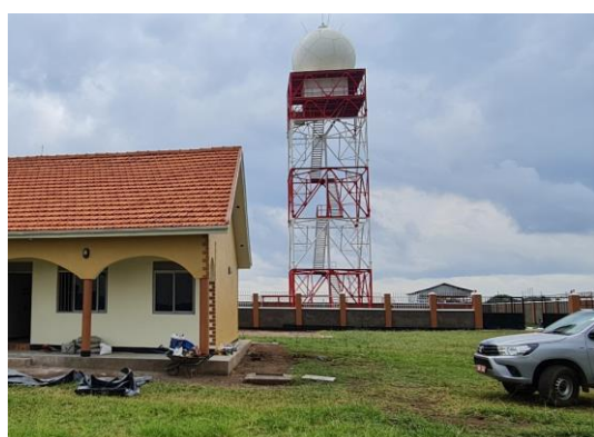
The radar in Lira District
