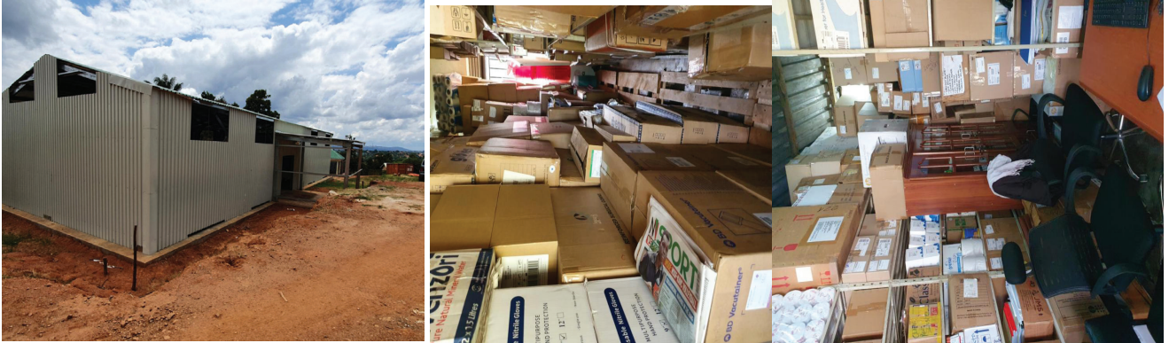
Stores (under construction) Store(headquarter)
