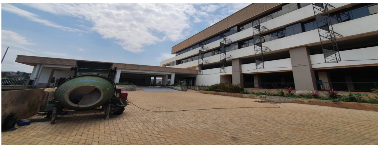
New stores for national medical stores under construction
