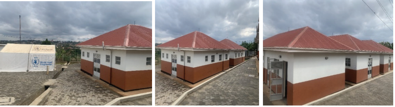
The newly constructed COVID facility:
