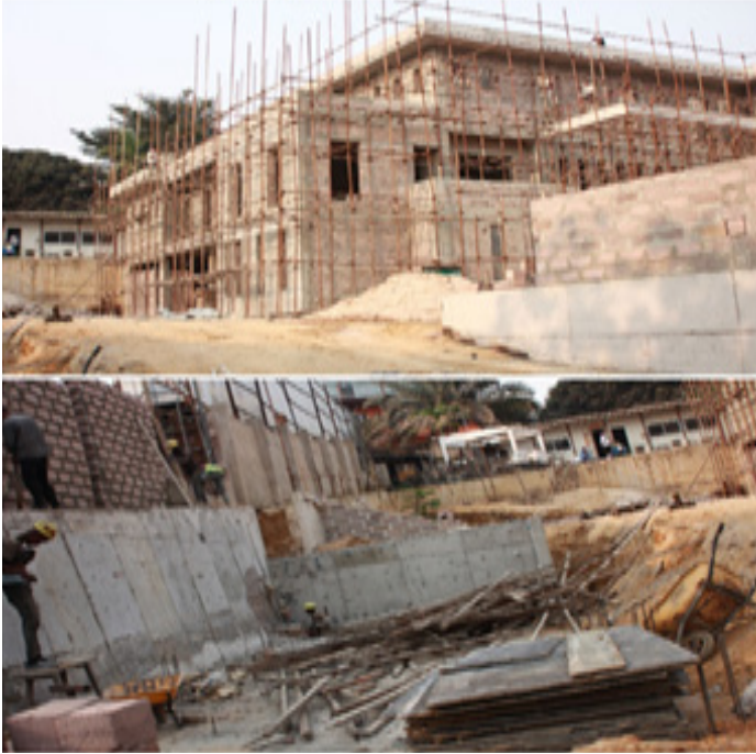
Construction of a new Chancery
