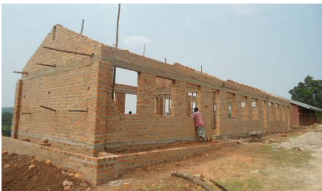
A two classroom block, and a five stance VIP latrine at whole plate at St Kizito P/S Kyengeza in Mityana District
