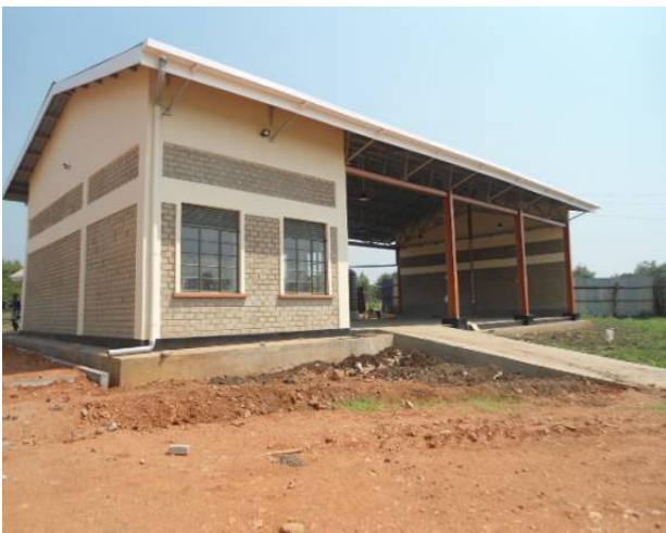
A BCP workshop completed at Kasese Youth Polytechnic
