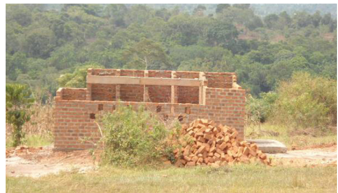
A two classroom block, and a five stance VIP latrine at whole plate at St Kizito P/S Kyengeza in Mityana District
