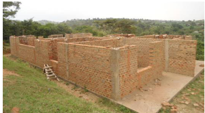
L-R: A 2-unit staff house at finishes level; A 2-unit staff house at ring beam level at Kazo T/I (formally Kiruhura T/I) in Kazo District
