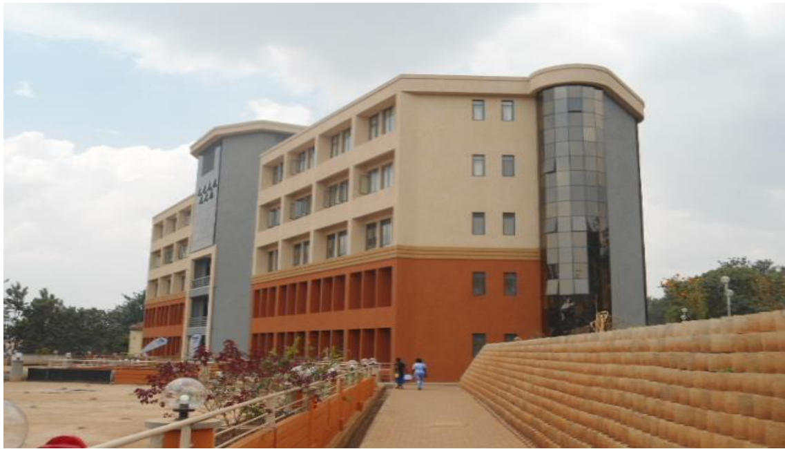
The office/classroom block completed at UMI
