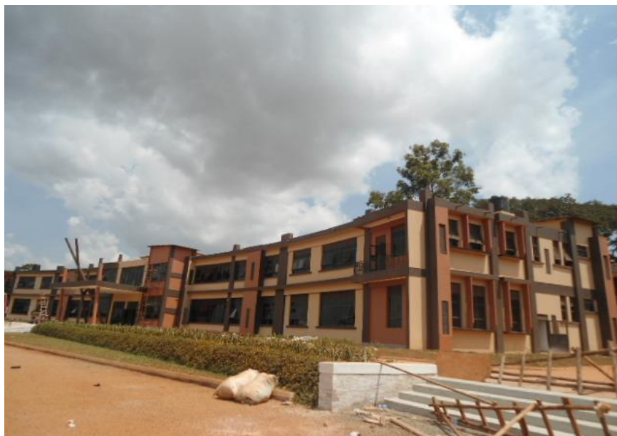
The completed lecture block at Kyambogo University
