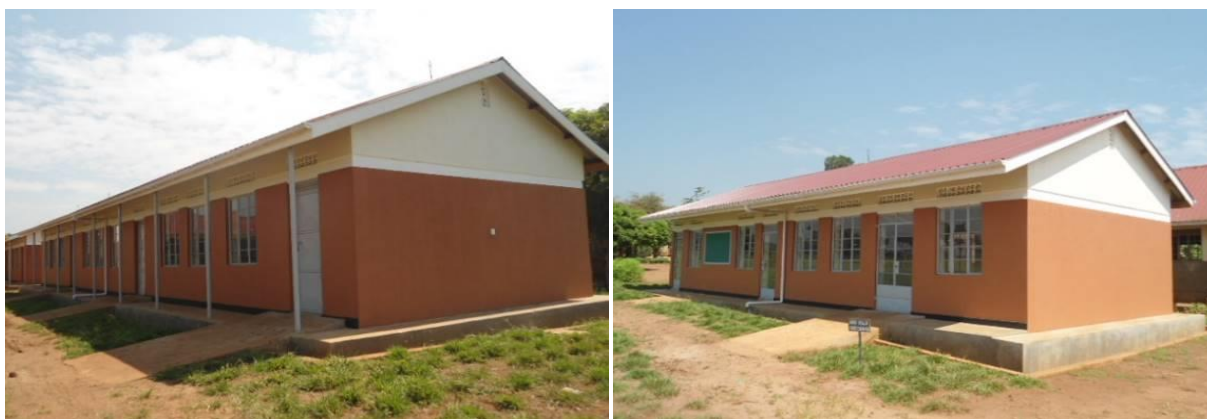
Completed classroom blocks at Bwetyaba UMEA P/S under UTSEP project in Butambala District
