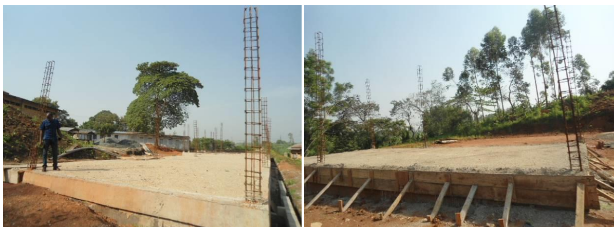
Construction of an MV workshop and a 2 classroom block at St. Joseph Virika VTI at DPL level as at January 2019
