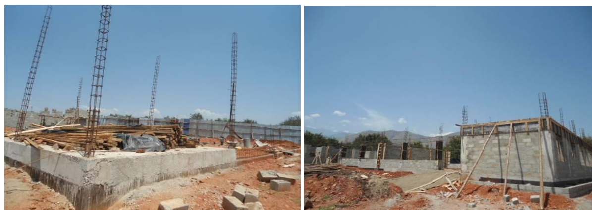
Left: Construction of BCP at sub-structural level and an Electrical Installation and Renewable Energy Workshop at ring-bim at Kasese Youth Polytechnic as at January 2019
