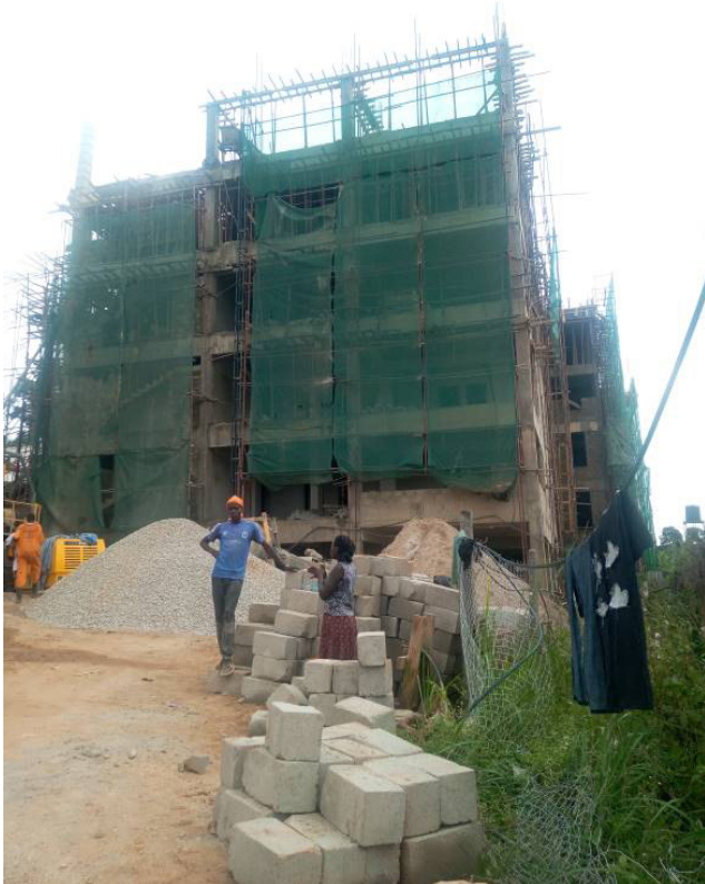
The 6-floor UNEB storage facility at Kyambogo at 85% progress
