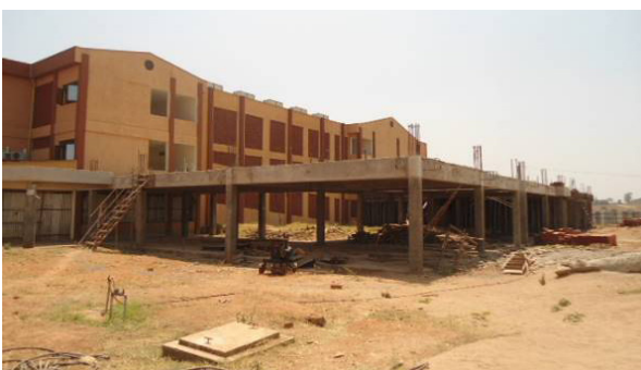
The Health Science laboratory at 35% progress at Muni University
