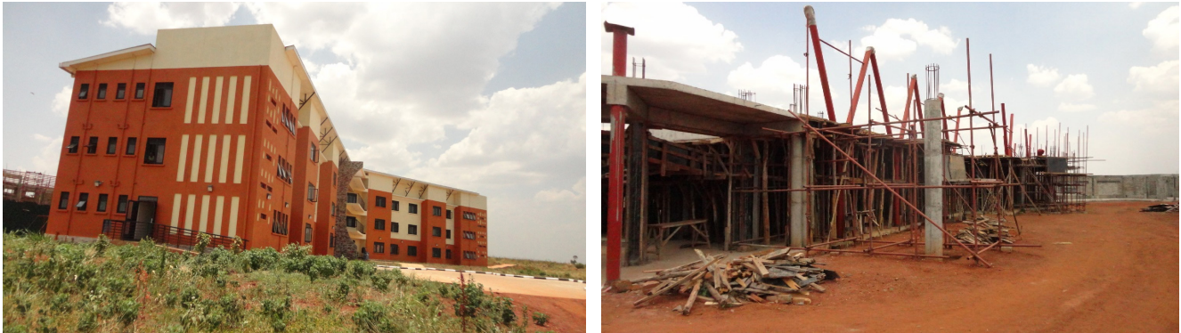
Left-Right; Male Hostel, and the Classroom block (3 floors) under construction
