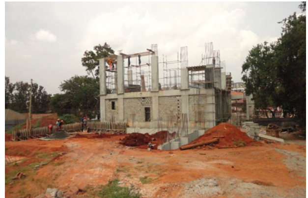
The new School of Public Health building under construction
