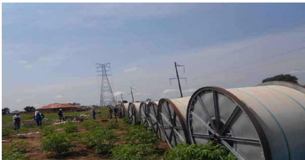
Ongoing tower stringing works on the Tororo-Lira line in Kumi
