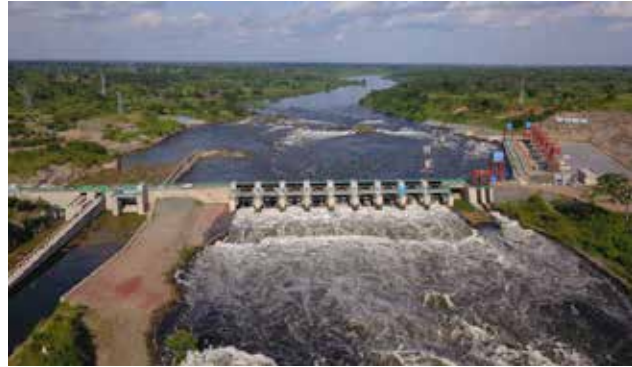
L-R: Substantially completed switchyard at Karuma HPP; Completed spillway, fish ladder and power intake structures at Karuma HPP
