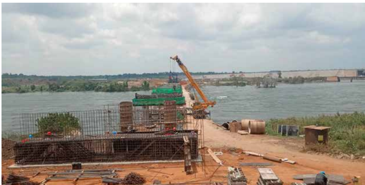
Ongoing civil works on the bridge at Isimba HPP
