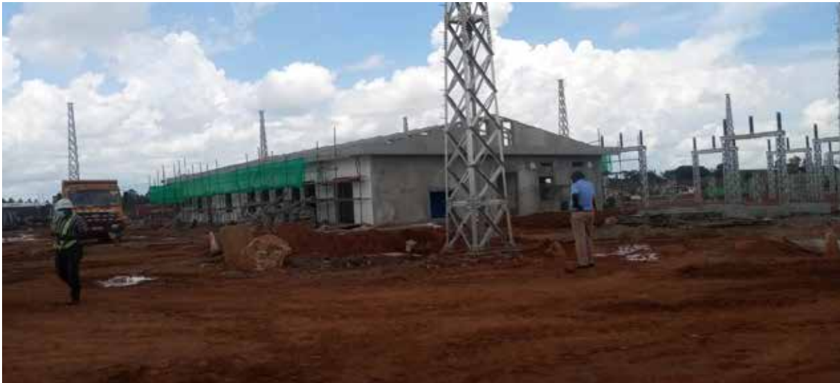
On-going civil and electromechanical works at the 400kV Olwiyo substation
