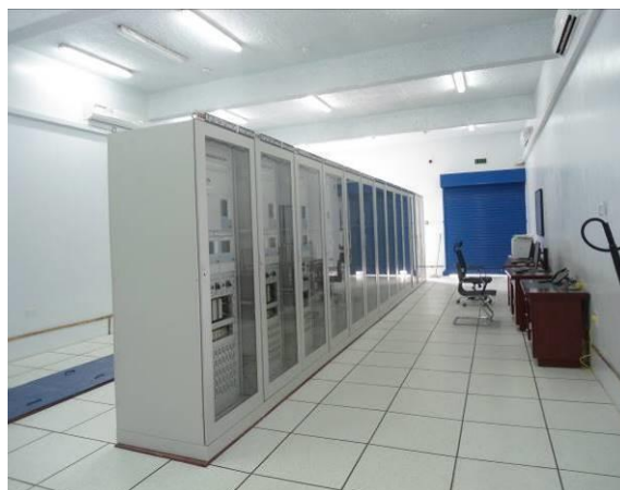
L-R: Completed grid extension schemes in Kaduggala-Kalungu District, Completed Control room at the newly constructed 220 kV Masaka substation
