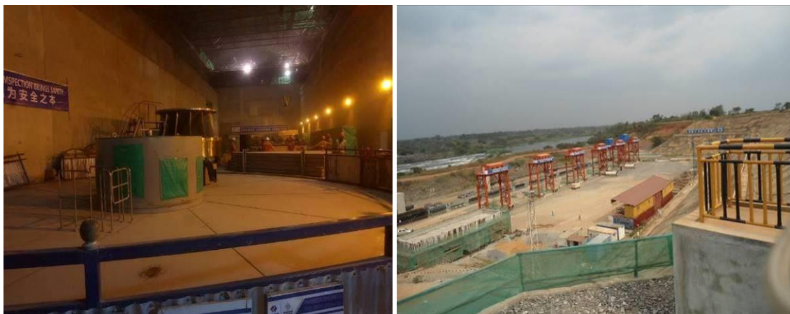
L-R: Electromechanical works in the power house showing a partially completed generator unit, Ongoing works at the power intake
