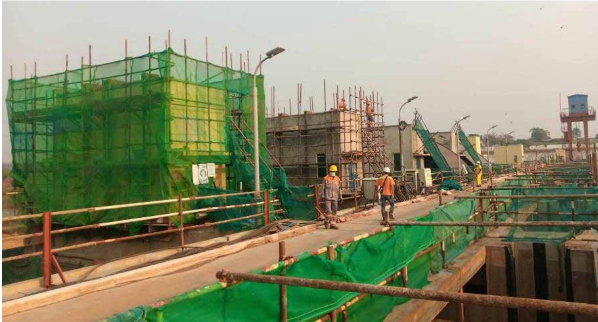
Ongoing finishing works on the hoists at the Karuma HPP
