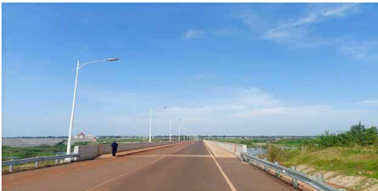
Completed public access road and bridge at Isimba HPP
