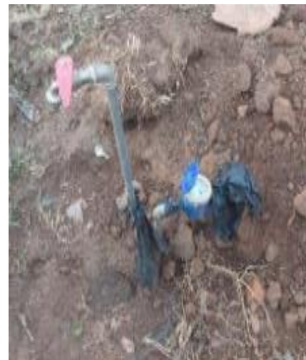
A yard tap of Orom WSS of Acholibur supply area in Pader District
