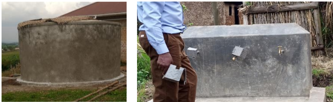
L-R: A 10m 3 Rain Water Harvesting Tank and its connecting Public Stand Post at Kyakahimbi P/S in Mitooma Town Council, Mitooma District
