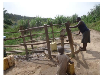
Nyamugusa rehabilitated borehole in Kabasekende Parish, Kibaale District
