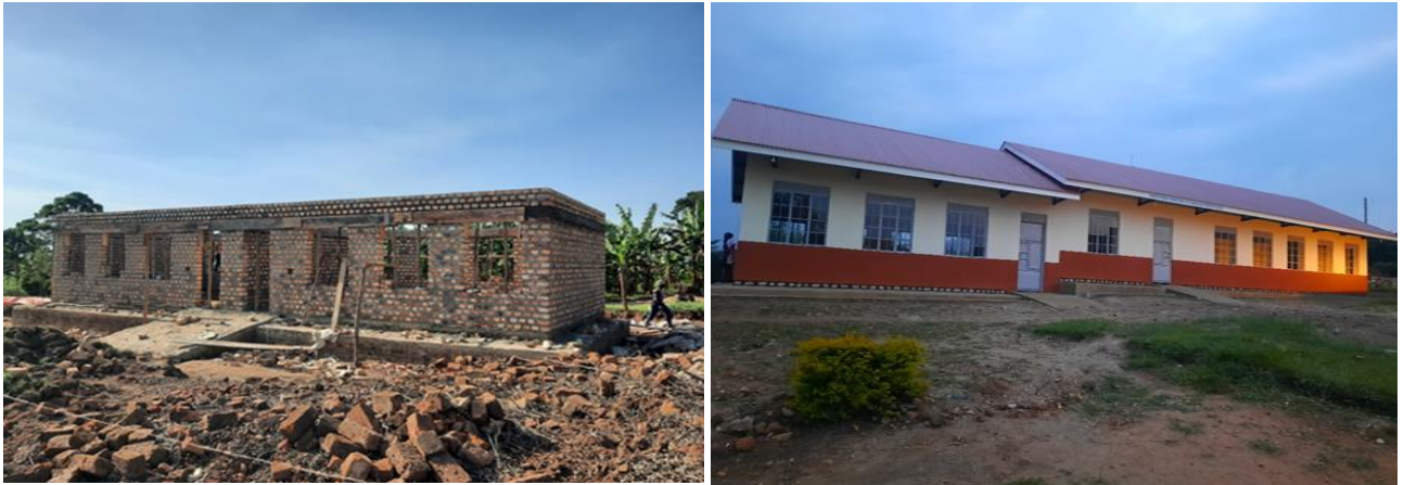
L-R: A two-classroom block constructed at Kitembo Primary School, Kalungu District under the SFG, and a two-classroom block constructed at Kasheshe Primary, Rukungiri District under the Transitional Grant
