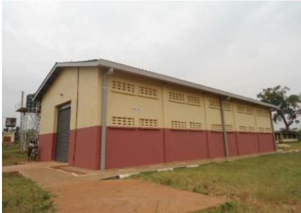
Renovation of the feed mill completed at Bukalasa Agricultural College
