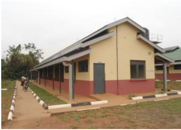
Renovation of a pullet barn completed at Bukalasa Agricultural College
