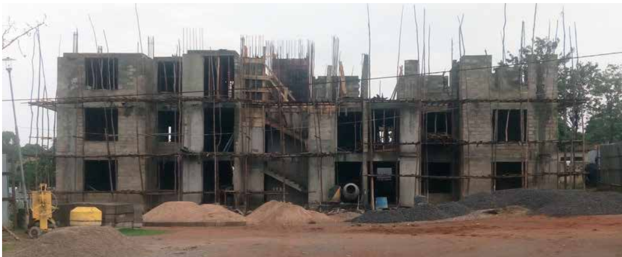
Front View of the Staff house under construction at Arua RRH
