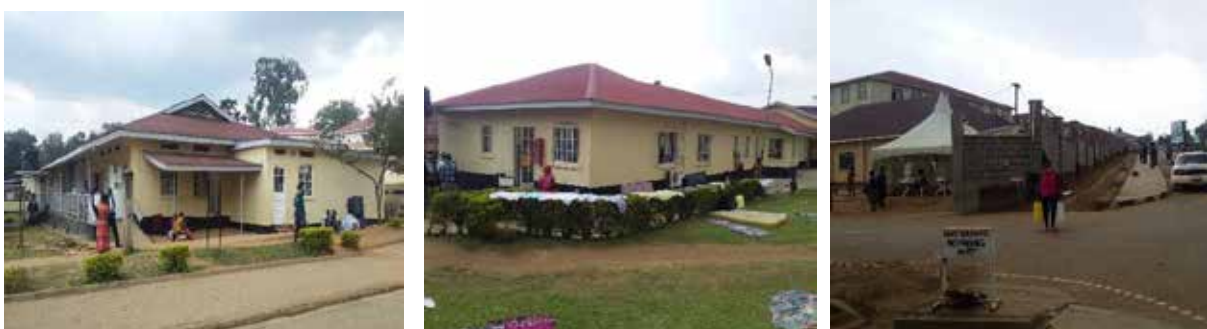
L-R: Rehabilitated OPD, Rehabilitated Medical ward and Perimeter wall at Mbarara RRH
