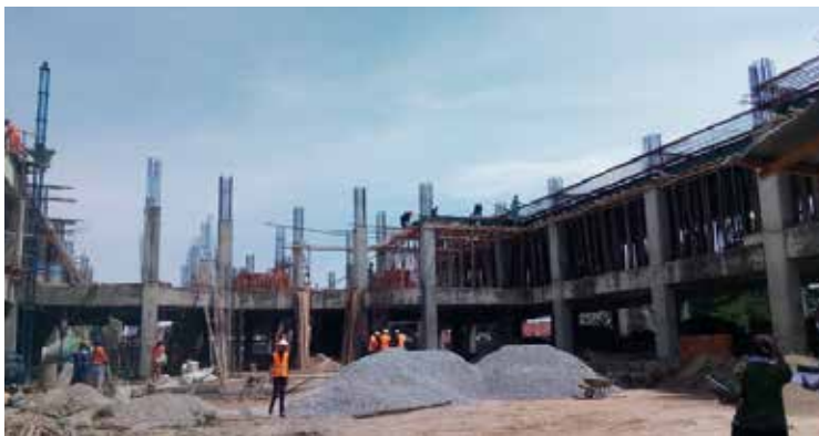
Surgical Complex under construction at Mbale RRH
