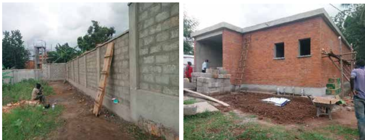
Left: Boundary Wall under construction Right: Substantially completed radiology structure remodeled
