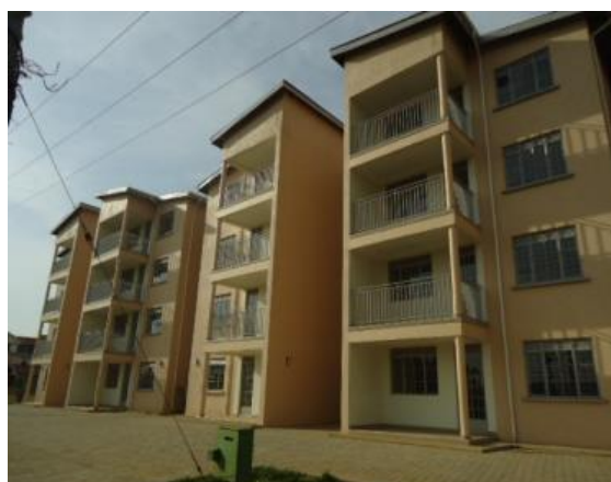
Completed staff house at Mbarara RRH
