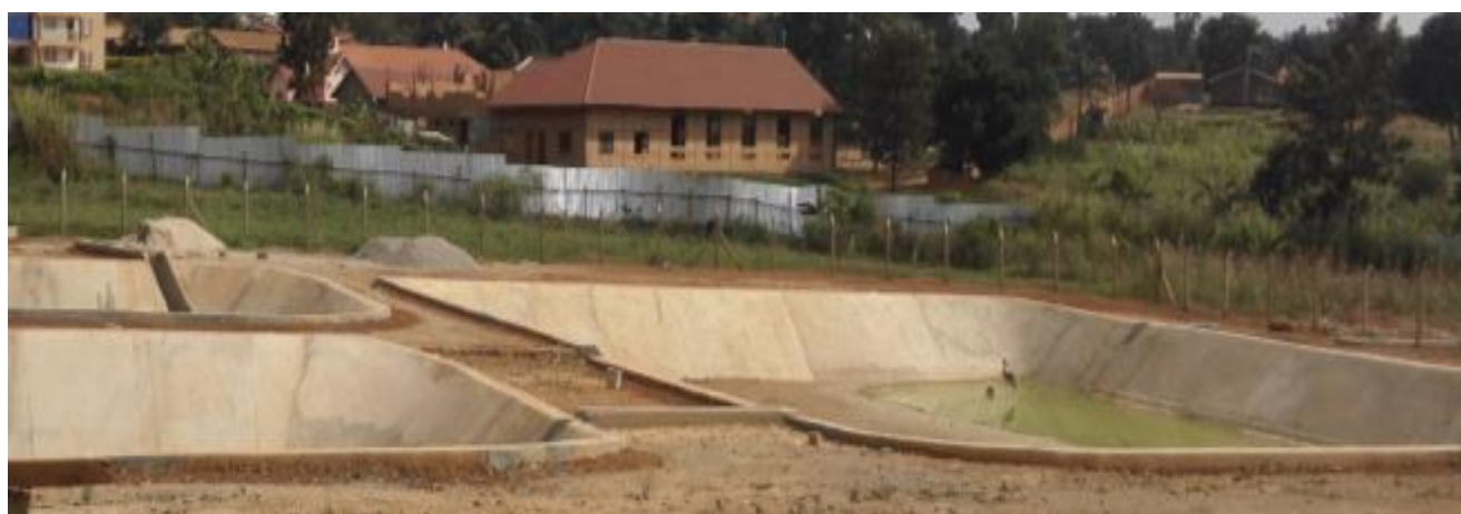
Lagoon at Substantial Completion at Hoima RRH
