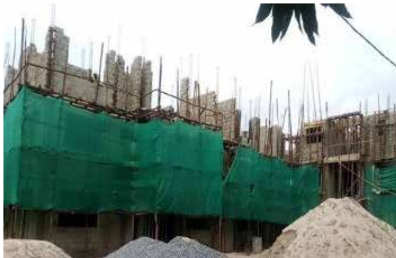
Staff house under construction at Jinja RRH, in December 2019
