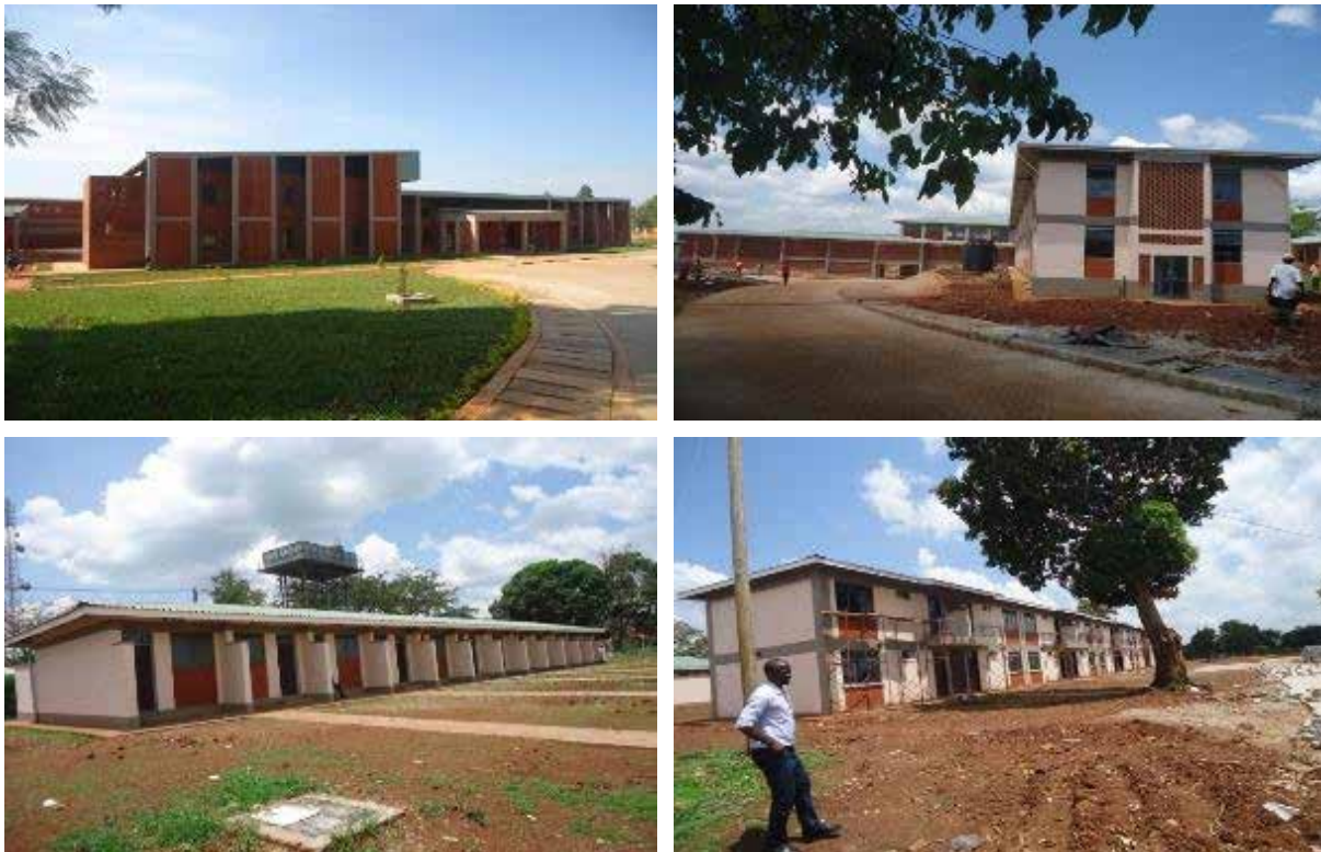
Clockwise: New hospital building; Old wards (T-Block); new staff quarters and rehabilitated old staff quarters at Kayunga Hospital
