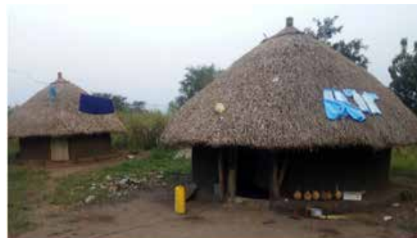
Staff houses constructed by local community at Koch-Lii HCIII in Nwooya District
