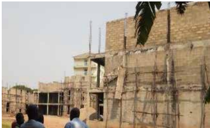
Status of Gulu staff house under construction
