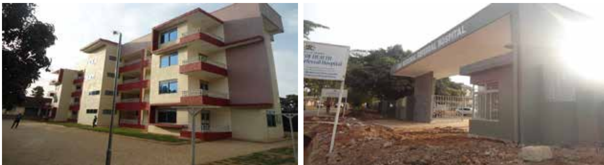
Completed Staff quarters and perimeter wall with a gate at LRRH
