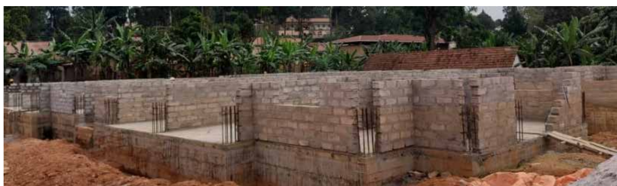
Forty-unit staff house under construction at Masaka RRH
