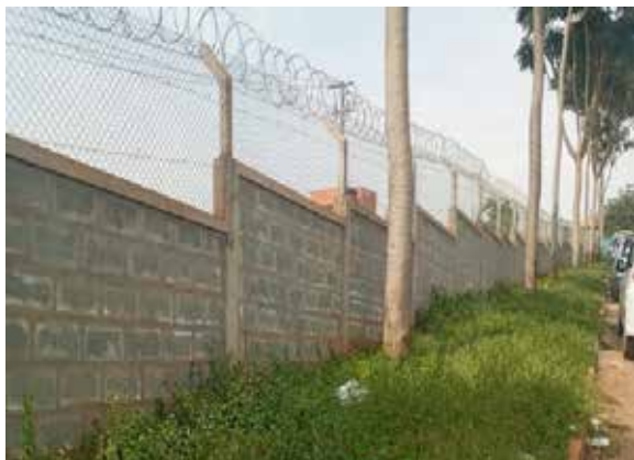
Completed Boundary wall at the Assessment Centre, Mulago NRH
