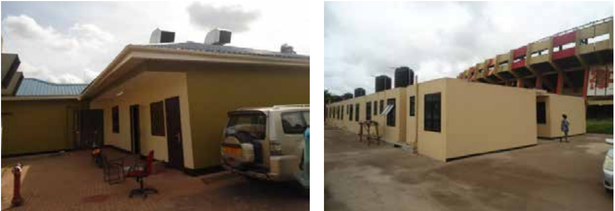
L-R: Oxygen Plant House at Mulago National Hospital and staff house at Namboole National Treatment and Isolation Facility
