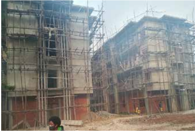
Interns hostel under construction at Kabale RRH
