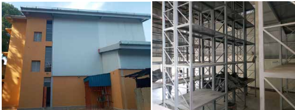
Left: Exterior view Right: Interior of the cold rooms and stores at Nakasero
