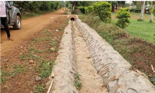
Kamuli District: Stone pitching along Mbulamuti S/C HQ -Railway Station (1.9km)
