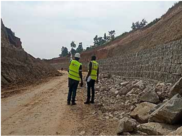
Gabion Embankment protection works on Rukungiri-Kihihi-Ishasha Road
