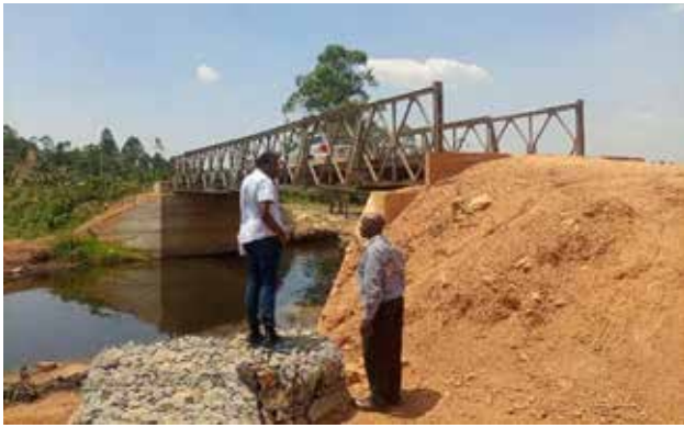
Kibaale District: Muzizi Bailey Bridge in Kayakazire Sub-County
