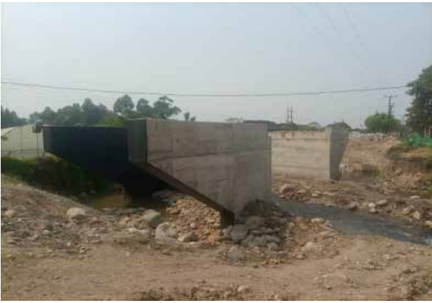
Completed abutments of Rwembyo Bridge in Kasese District
