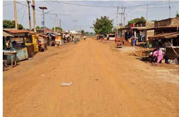
Kamuli District: Butabala-Namisambya-Kitayundwa Road (5.8km) after rehabilitation works
