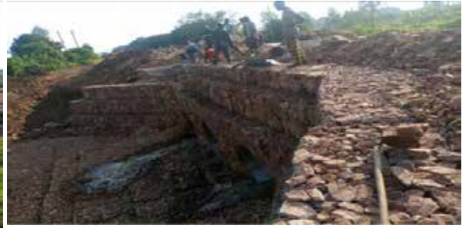
Kabale UNRA Station: Restoration works along Kabale-Muhanga-Ntungamo Road
