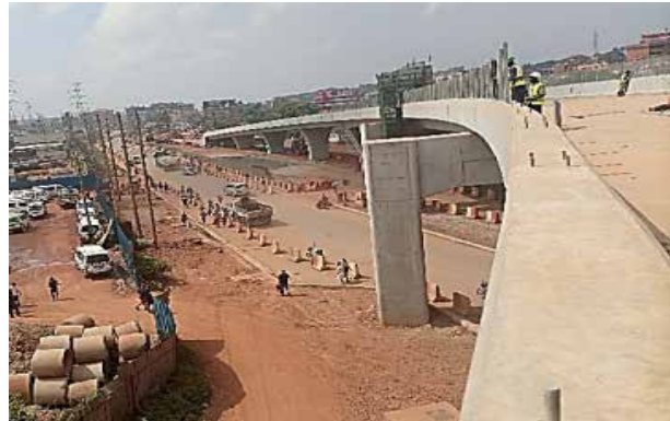
An overpass from clock tower –Nsambya on the Kampala Flyover
