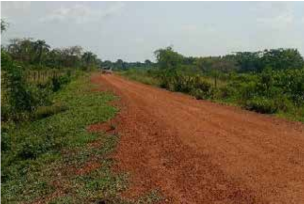
Mukono District: A section at Km 0+900 on Kakooge-Nakasenyi-Mulembya Road (2.0km) after rehabilitation works
