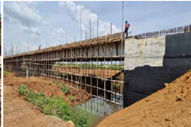
Alleles Bridge under construction in Pallisa District
