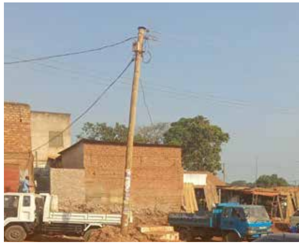
The electric pole within the Right of Way that is pending relocation in the 200m section on the Kitala-Gerenge Project
