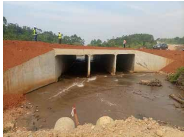
A three-cell box culvert at km 38+700 on Rukungiri-Kihihi-Ishasha Road
