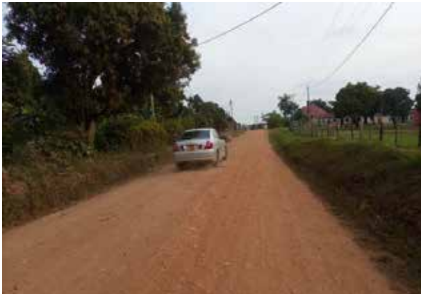
Mukono Municipality: A section of Nyenje Budugala Road at km 1+300 where routine mechanized works were carried out
