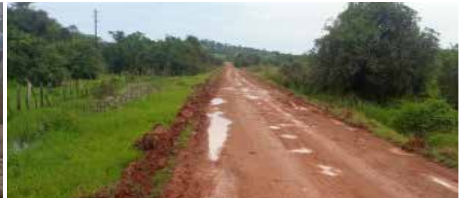
Masaka UNRA Station: A section of Mateete-Kyabakuza Road at km 32+600 in a bad state
