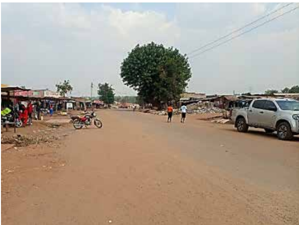
A primed section of Kinali Rise as part of the Kigumba-Bulima Town roads
