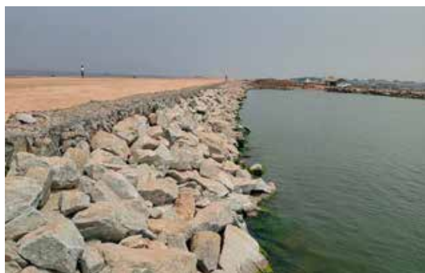
Wanseko Landing site: The access road to the site that was constructed by the Hoima-Wanseko contractor
