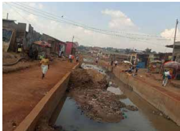
KCCA-KIIDP 2: Nakamiro Channel under construction in Kawempe Division
