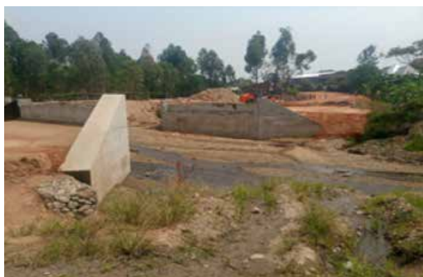
Constructed Abutment walls of the Kajwenge Bridge in Kasese District
