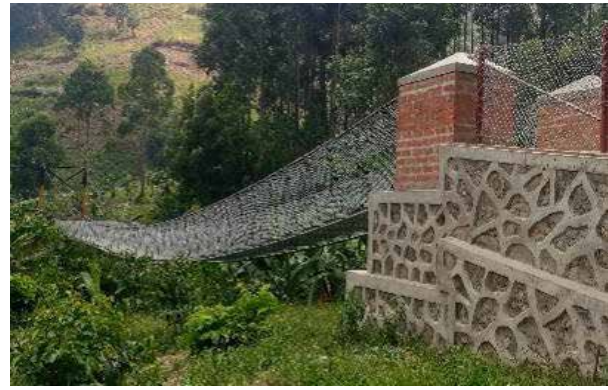
Kasese District: Completed Ruboni Foot Bridge
