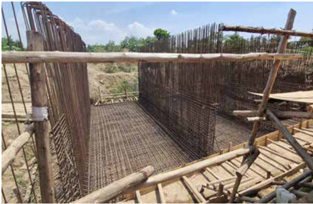
Tororo District: Steelwork for Aderema box culvert
