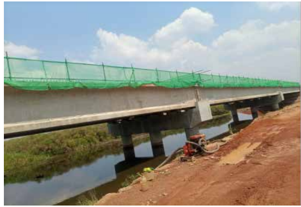
Bridge section at Lugogo Swamp crossing in Nakasongola District
