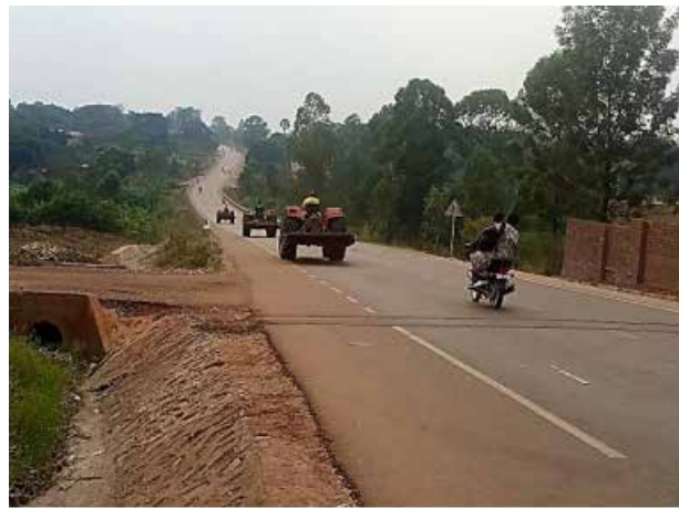
A completed section of Municipal-Hoima Road as part of the Kigumba-Bulima Town roads
