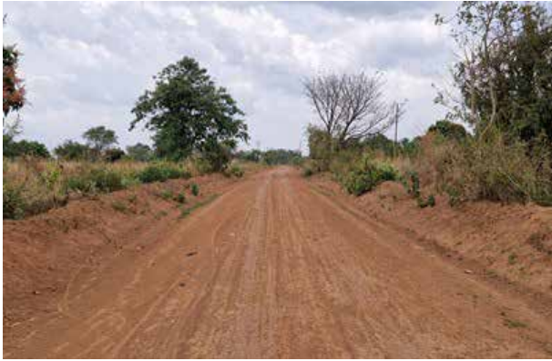
Soroti District: Akaikai-Oduui Road (7.2km) after periodic maintenance in Q2
