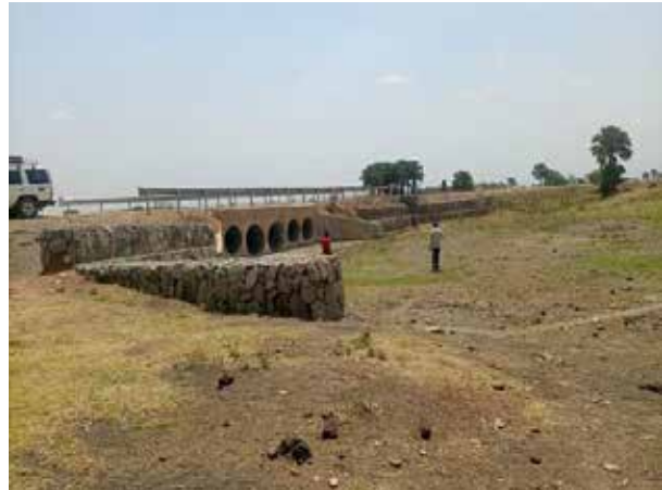
Ntoroko District: Five armco pipe culvert lines installed on Rewbisengo Road
