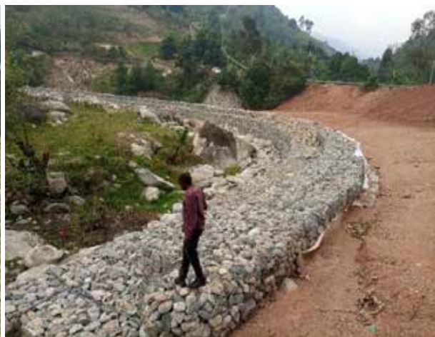
Kasese District: Nyamusangani river protection works
