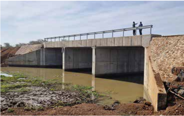
UNRA Bridge: Completed Multi-Cell Box Culvert at Ajeleik
