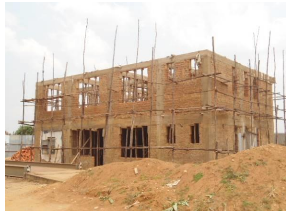
Completed substructure and administration block awaiting roofing at Kayonza Tea Factory
