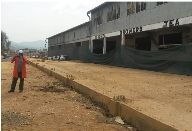
Completed substructure and administration block awaiting roofing at Kayonza Tea Factory
