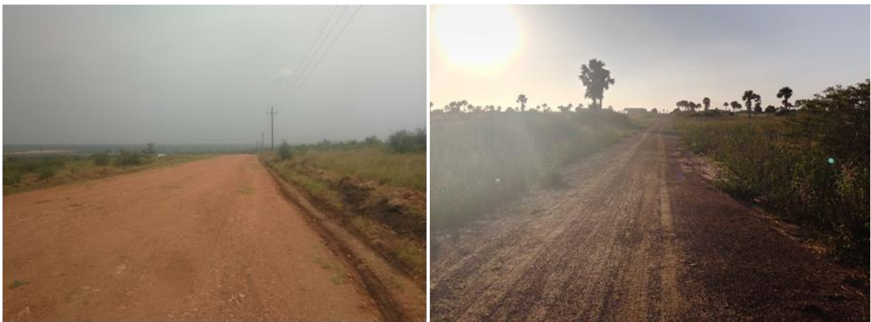
L-R: Maintained gravel road in Kasese IBP; and unmaintained road within Soroti IBP
