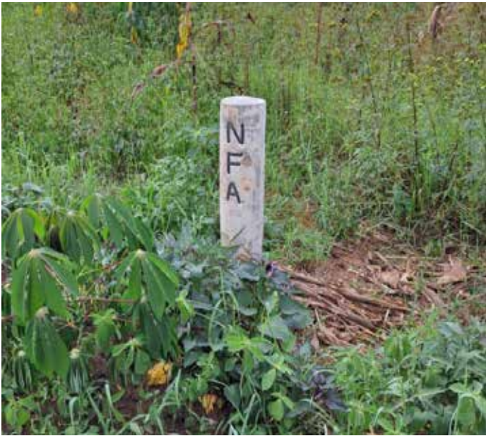
Boundary Marking with a concrete Pillar at L. Wamala in Mityana District
