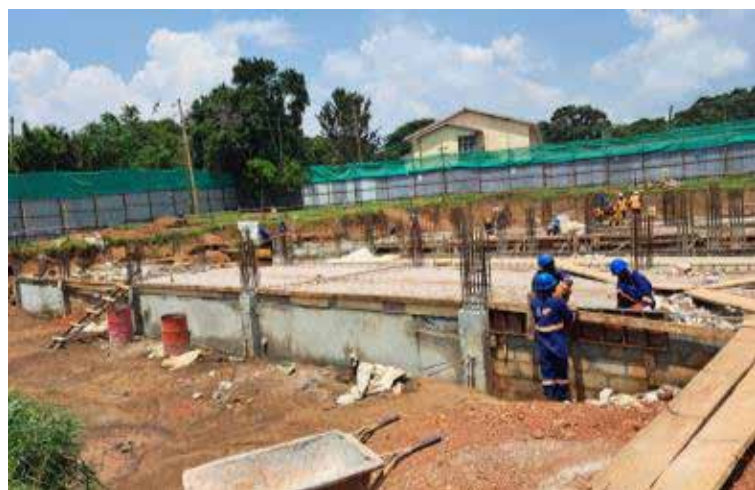
Ongoing construction of the National Water Quality Reference Laboratory in Entebbe
