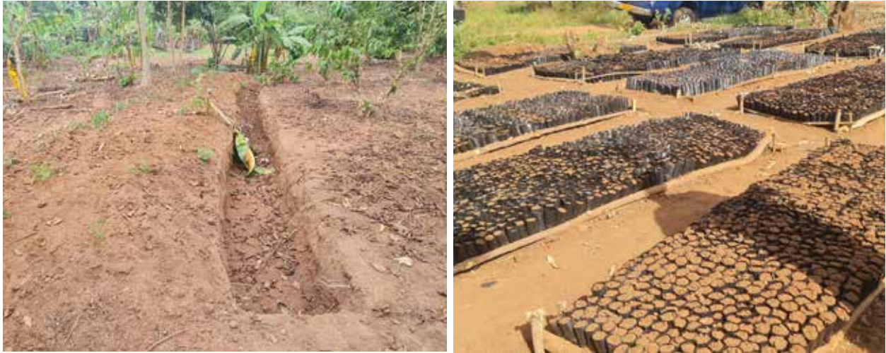
Left: Soil and flood control structure on demonstration farm land in Bulumba town council Kaliro District
