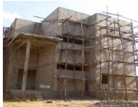
Incomplete support to Teso Regional Office in Soroti Municipality
