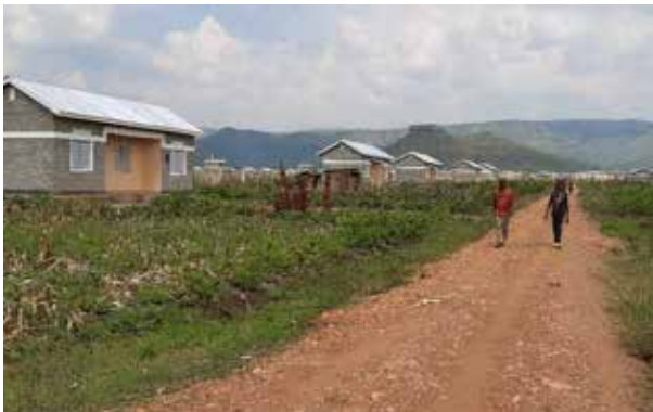
Constructed access roads in resettled communities under Phase II in Bunambutye Town Council, Bulambuli District
