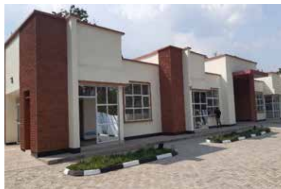
Newly constructed Kasese Service Centre, Kasese Municipality
