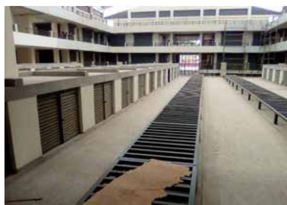
Completed lockup shops in the Soroti Market
