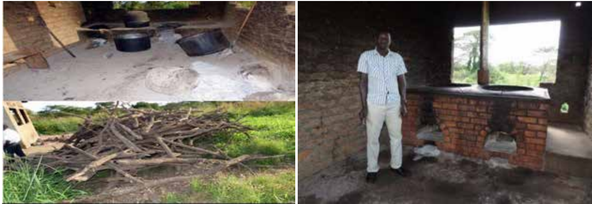
L-R: Traditional stove used before; improved twin energy cook stove at Paicho Senior Secondary School, Gulu District
