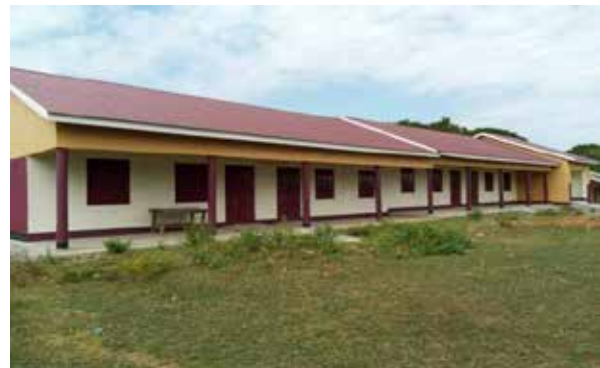
Completed classroom block and toilet at Kaler Primary School in Ngora District
