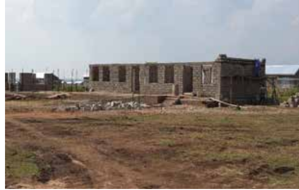
Ongoing civil works on new classroom blocks
