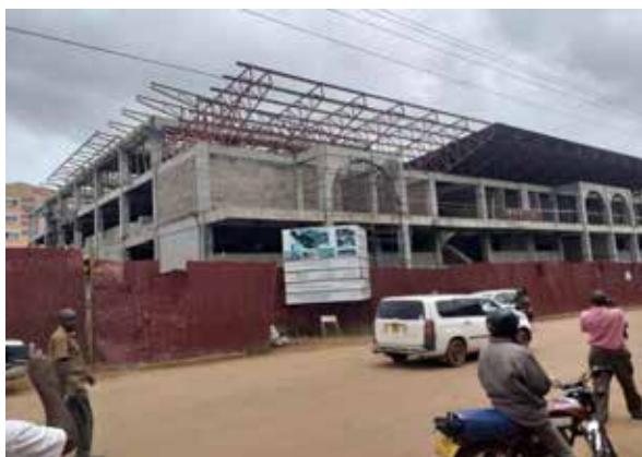
Roofing and plastering ongoing at Masaka Central Market
