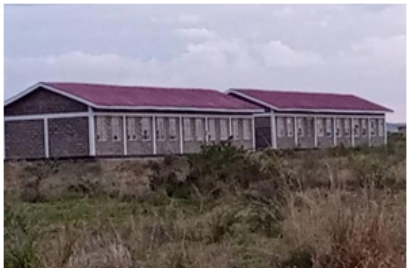
Completed two classroom blocks at Bunambutye Primary School, Bulambuli in March 2020
