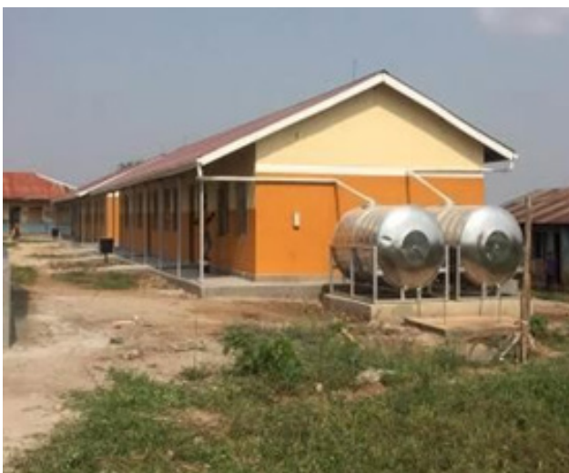
Completed 2 three in one classroom blocks at Nyamasoga primary school in Hoima District
