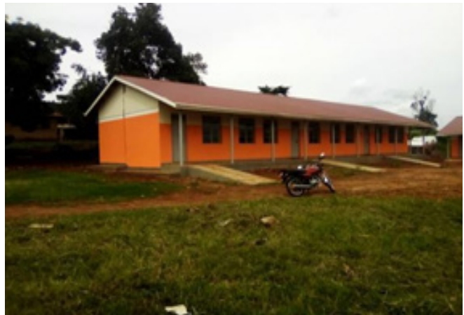
Complete classroom blocks at Kabwoya Primary School Kikuube District
