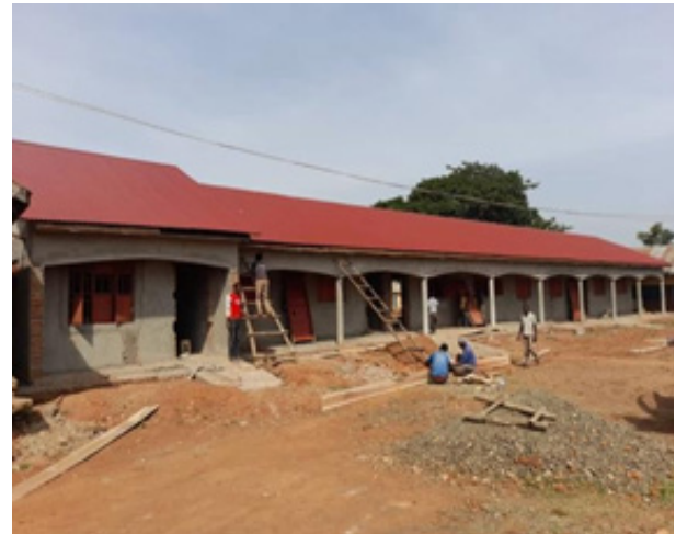
Ongoing construction works at Kachumbala Primary School in Bukedea District
