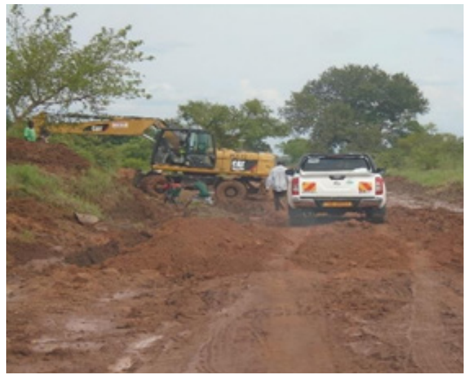
L-R: Compacting 95% BS heavy; Repair of eroded section along Atiak-Gulu Road
