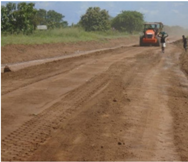
L-R: Compacting 95% BS heavy; Repair of eroded section along Atiak-Gulu Road
