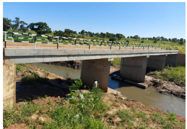
Newly constructed bridge on the Cetkana-Palyec (5.7km) CAR, in Gulu District
