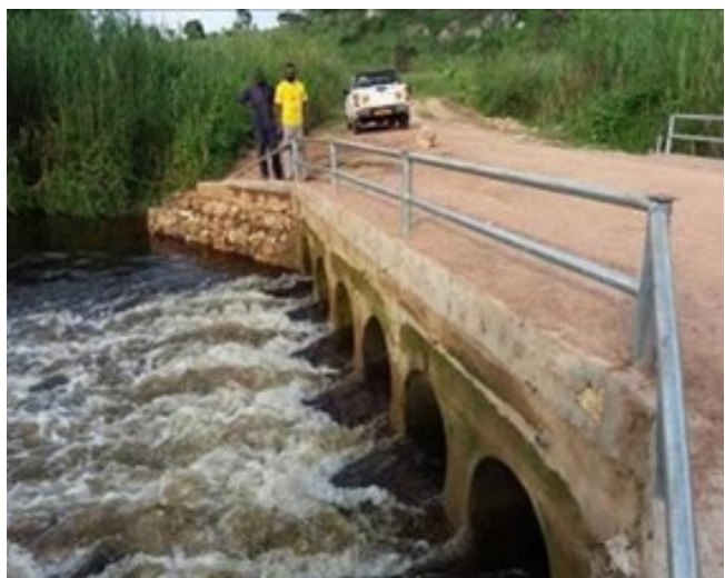
Full rehabilitated Kyegegwa-Nkomangani- Kasenene Hamwogo - Buraro, 27kms in Kyegegwa District
