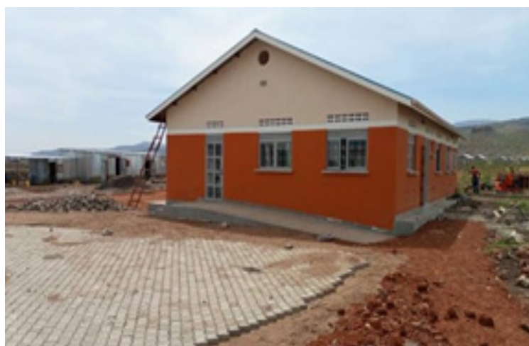
Ongoing works at Bulambuli HC III in Bunambutye sub-county
