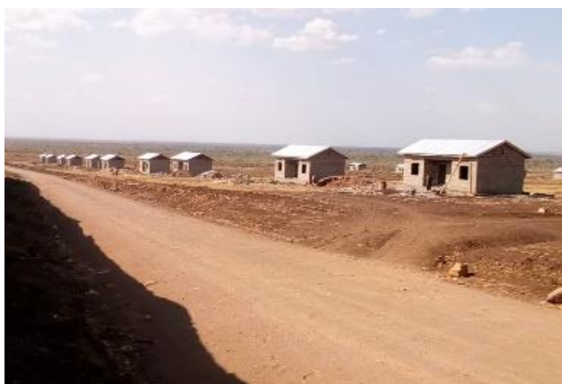
Superstructure of resettlement housing units constructed by Uganda Police in Bulambuli district as at January 2019
