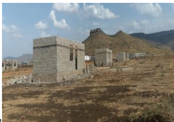
Housing units at wall plate constructed by UPDF as at January 2019
