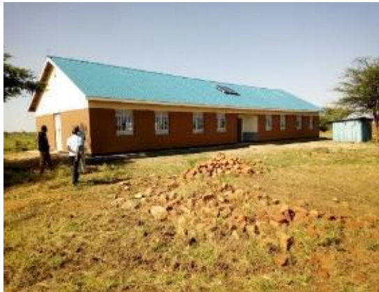
Completed Dormitory at Nadunget Primary School in Nadunget Sub-County, Moroto District as at January 2019
