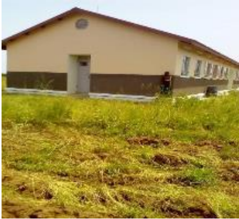
Completed Girls' dormitory at Lolachat Primary School in Nakapiripirit district as at January 2019
