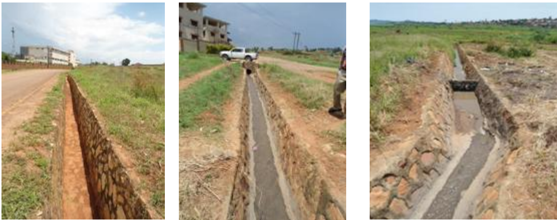
Left: De-silted drains in Luzira Right: Untreated waste water released to the park side drains
