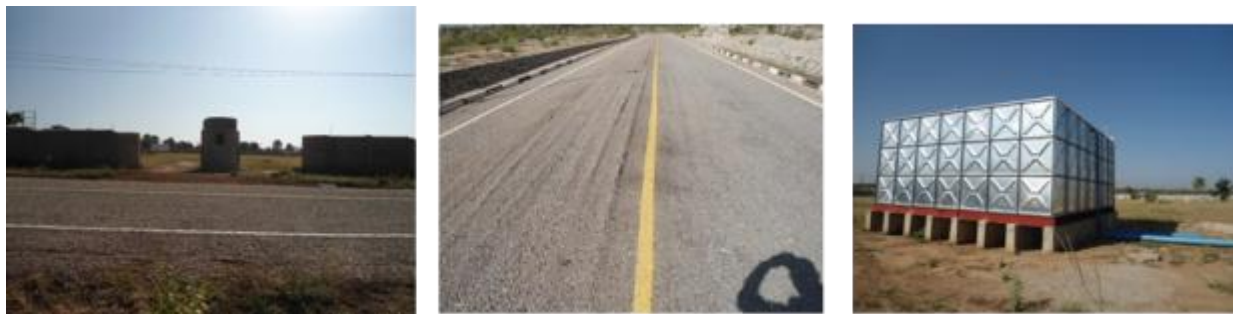
Left: Incomplete section of the perimeter wall Centre: Failing section of the road Right: Installed water reservoir
