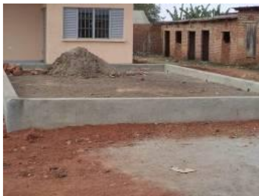
Uncompleted drying slab in Mbale district
