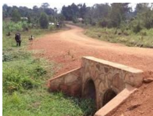
Installed culverts and swamp raised section of the road in Jinja district
