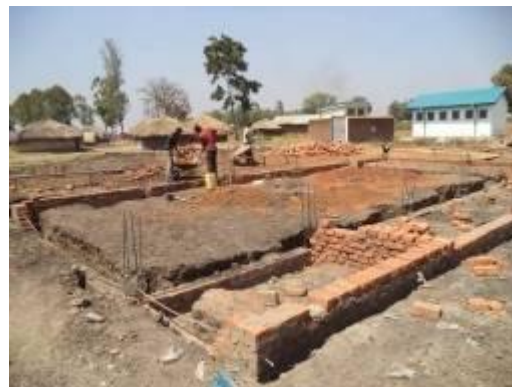
Ongoing construction works at t maize mill facility and excavated pit latrine in Gulu district
