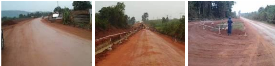
Left: completed subgrade section; Centre: ongoing earthworks; Right: Swamp section on km 12+600 awaiting rock fill
