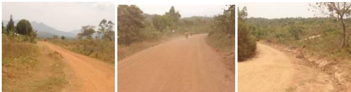
Sironko District: Left: A slashed section on Bukiyi-Kibembe road; Centre: A graded section on Bumundu-Namanyonyi road; Right: A graded section on Nampanga-Buwalasi road
