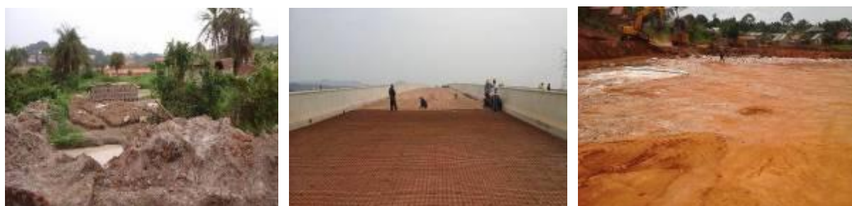
L-R: Obstruction of works at km 9+100 by fish ponds; Fixing of reinforcement at Busega Bridge; Earthworks ongoing at km24+500
