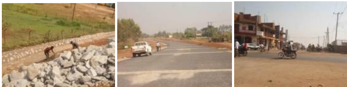
Left: Stone pitching works at Km 69+000; Centre: A section where the 1 st seal had been done; Right: One of the building in Arua town junction which has obstructed round about construction
