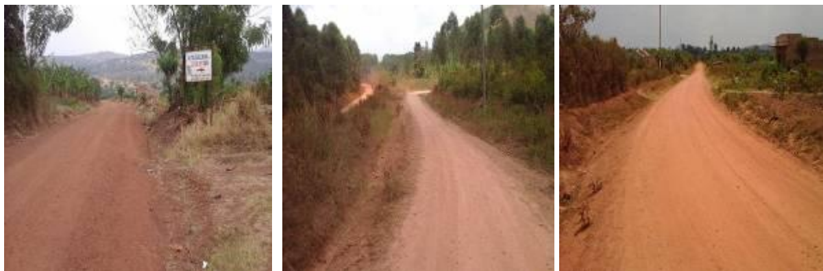
Lyantonde District: Left: A Graveled section at km 11+300 along Kasambya – Kitazigolokwa road; Centre: Graded section at km 7+300 along Kiyinda – Kitesa - Twafanda road; Right: A graded section along Karagala-Kitovu road
