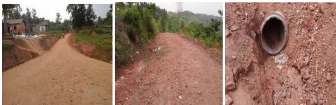
Mityana District: Left Gravelled section along Naama – Buswabulongo road; Centre: Loose gravel at km 3+000 along Mpiringwa - Kasenyi road; Right: incomplete culvert end structure at km 2+800 along Mpiringwa - Kasenyi road
