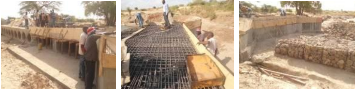
Moroto UNRA Station: Left: The existing drift with culverts and the new construction box culvert works with scaffolding; Centre: Reinforcement for the decking; Right: Gabion protection works at Naoi Bridge on Kokeris-Lopei road
