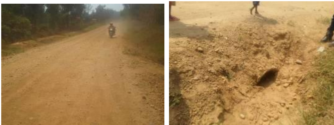
Kabale UNRA Station: Left: Graded section at km 14+700; Right: Culvert needs to be opened at km 7+000 on Katojo Kihhihi road
