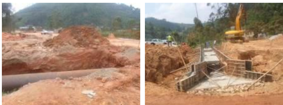
Left: Armco culverts yet to be constructed at km 155+628; Right: A box culvert under construction at 1.4km from Katuna
