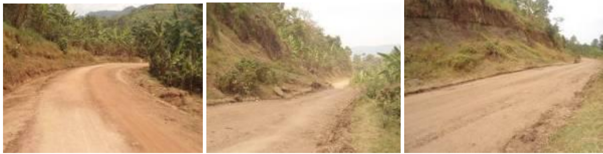
Sironko District: Bweri-Bumunulo road; Left: A graded section of the first 4kms; Centre and Right: A section at Km 5+200 which was affected by landslides
