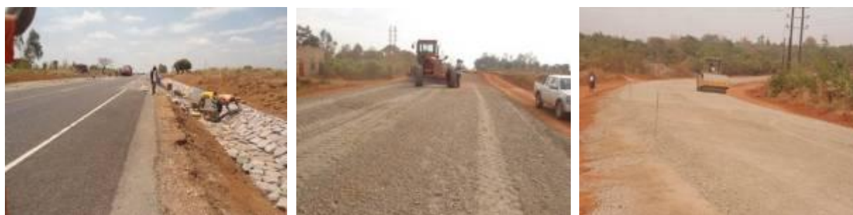
Left; Stone pitching works at km 35+580; Centre: spreading of road base material at km 1+200; Right: compacting of road base at km 1+100
