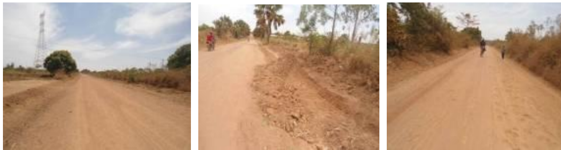
Soroti District: Left: A graded and shaped section of Aponyi-Obito Road (6km); Centre: An offshoot at Km 14+100 on Soroti-Lalle road; Right: A defective section with dust on Asuret-Amagoro road at Km 8+500
