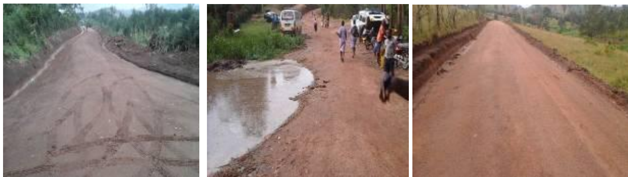
L-R: Graded section of Rukanga Primary School road ready to receive gravel; very well graded section of Nyakatojo – Kabumba section; Unworked on swampy section at 0+200 along Kikonje – Rwashamire road, works have not yet started because of lack of culverts.
