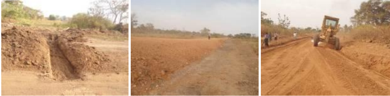
Serere district, Kasilo County, Olwa-Obangin-Otoba road: Left: Excavated trench for pipe culvert installation at Km 4+200; Center: Swamp raising at Km 6+600; Right: Grading and shaping of the road at Otoba
