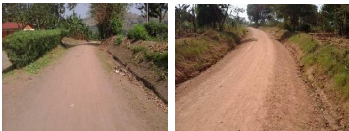
Ibanda District: Left: Graded section of Birongo – Kinagamukono – Kyekanga road at km 5+600; Right: Gravelled section of Kashasha – Nyakahama road at km 4+000
