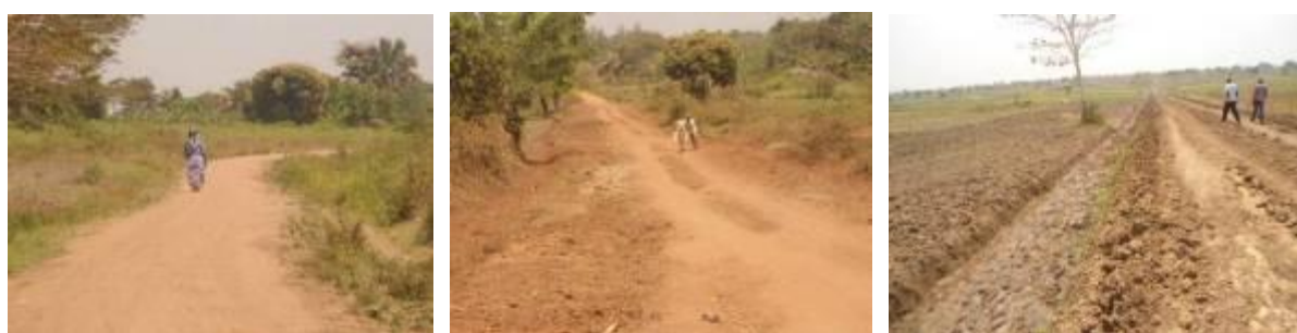
Budaka District: Left: A section of Kabuna-Nansana-Kebula road; Centre: A graded section of Nalera-Kiryolo road; Right: The swamp raising done using manual labour on Nalera-Kiryola road
