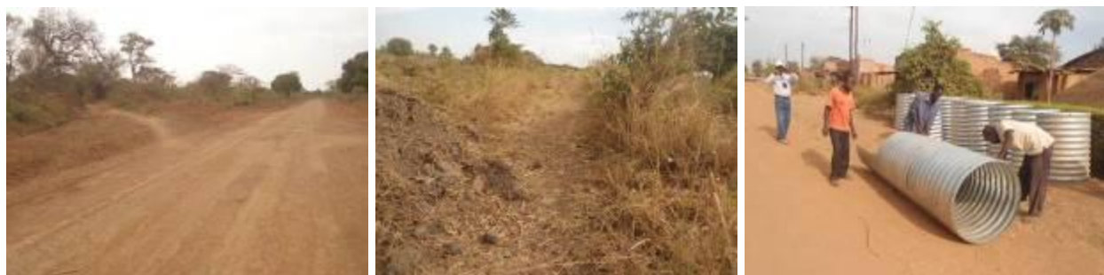
Serere District, Kasilo County: Adwenyi-Toror-Kilembe road: Left: The straightened re-aligned section at km 2+200 with the old section of the road (path) on the left; Center: A section of the old road that was avoided at Km 1+600; Right: Assembling of the Armco culvert pipe culverts at Apapa Police Post
