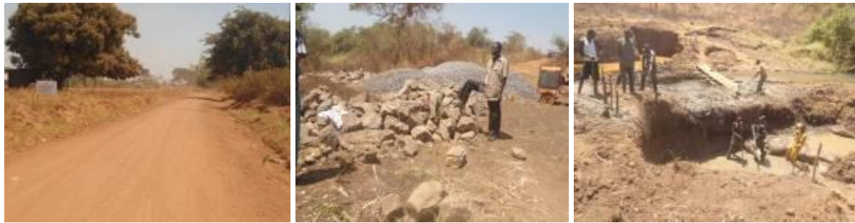
Gulu District: Left: Opit-Awoo road - A graded section at Km 11+100; Centre and Right: Odek Bridge – Construction materials on site and Excavation for the abutments
