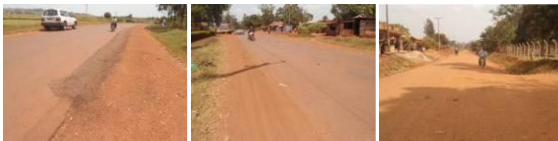
Jinja UNRA Station: Left; Patch works along access to Kimaka Military Academy road: Centre; A recharged shoulder along Access to Kimaka Military Academy road: Right; A section of Iganga-Nawangisa road
