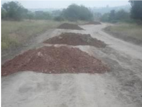
Isingiro District: Left: Dumped gravel at km 7+300 along Kyanyanda-Kihanda-Rwenshekye; Right: Grading works along Ngarama-Kakamba-Omukatogo road
