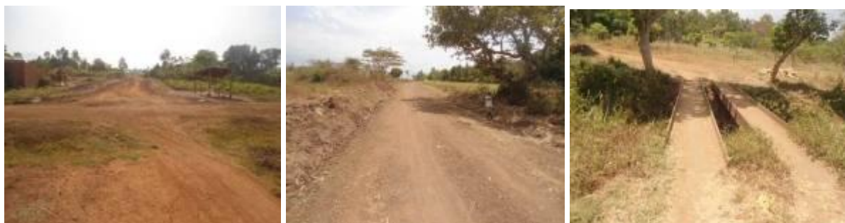
Sironko District: Left and Centre: Graded and shaped sections of Sironko Town Council – Kumira – Kilembe road; Right: I-sections used for the temporary crossing at the Soloni bridge crossing
