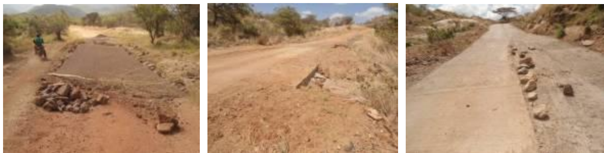
Moroto UNRA Station: Moroto-Rupa-Nakiloro-Nakabat road (28km): Left: Drift at Km 16+300; Centre: Drift at Km 20+100; Right: The 120m by 60m concrete pavement at the escarpment at Km 21+400
