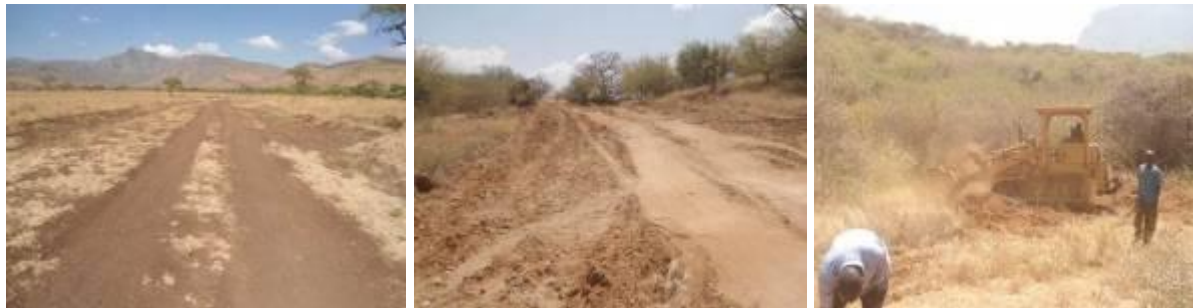
Moroto District: Left: A bush cleared section of Kodonyo-Lorengedwat road at Km 2+300; Centre: A Bush cleared section of Nakabaat-Narengenyia road; Right: A bulldozer clearing the bush on Nakabaat-Narengenyia road
