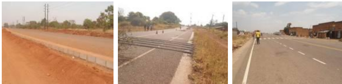
Left; Concrete lining along the road edge at km 0+800; (Centre): Rumble strips;(Right):A completed section at km 35+174
