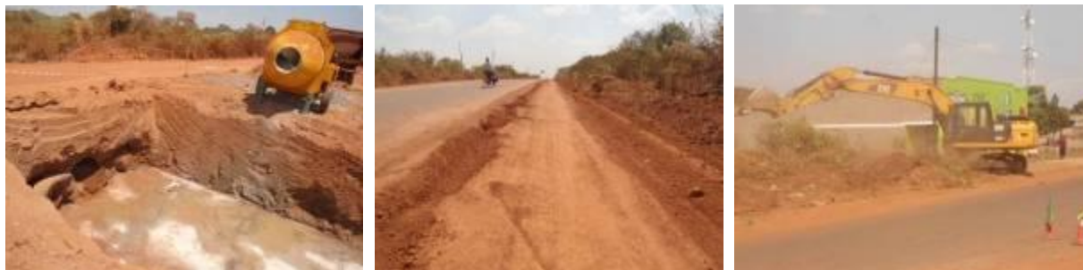
Left; excavation works for a culvert at km 2+370; Centre: rehabilitation of road shoulders at km 40+419; Right: Bush clearing with an excavator at km 59+000
