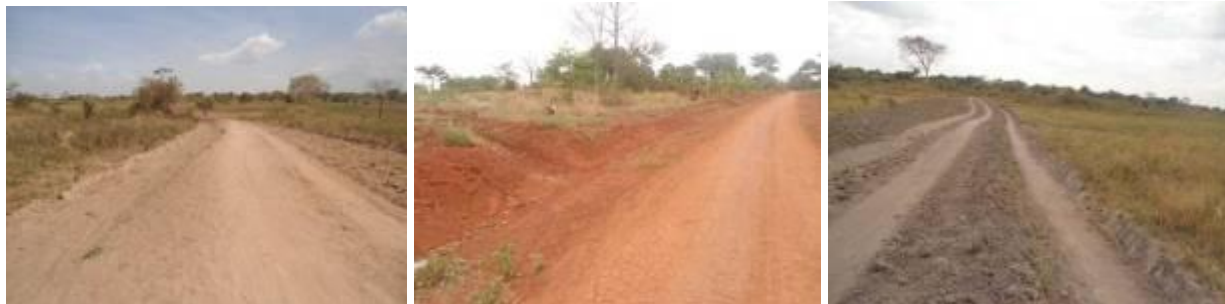
Left: A swamp section at Km 6.0 along Nsomba P/s-Igalaza road which need to be gravelled; Center: A bush cleared and shaped road section with an offshoot at Km 1.4 on Irapa-Kigwesi road; Right: A swampy section along Irapa-Kigwesi road between Km 5.4 and Km 7.1 where culverts were to be installed.
