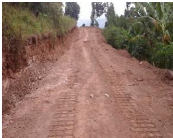
Section along Kikombe Trading centre-Lyashisha-Kyambura river crossing-Mukatojo road which requires deep cuts; Incomplete section along Kikombe Trading centre-Lyashisha-Kyambura river crossing-Mukatojo which has been graded
