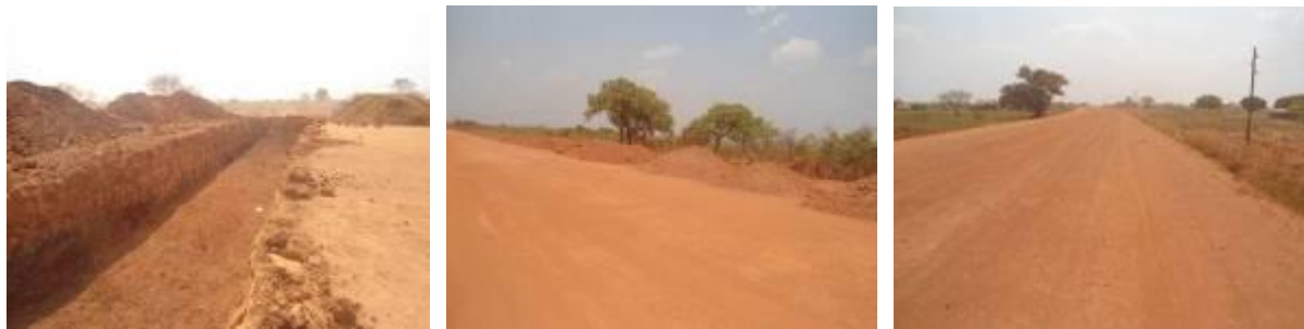
Left: excavation for pipe culvert at Km 96+430; Centre: Dumping of sub base at km 82+300 ; Right: milled section at Km 70+000
