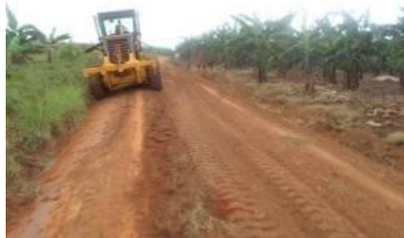
Isingiro District: Left: Dumped gravel at km 7+300 along Kyanyanda-Kihanda-Rwenshekye; Right: Grading works along Ngarama-Kakamba-Omukatogo road
