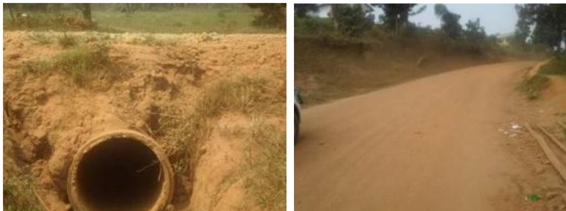
Kabale UNRA Station: Left: Incomplete culvert at km 20+600; Right: Completed section of the road for Kanungu-Kihihi-Ishasha road
