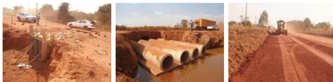
Left: culvert under construction at km 1+518; Centre: four lines of culvert at km 2+944; Right: A milled section at Km 19+545
