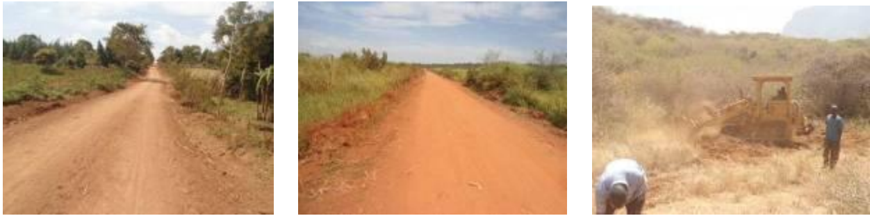
Mayuge District: Left: A graded and shaped section of Kaluuba-Luuba road; Centre: A regravelled section in a swamp at Km 2+900 on Kaluuba-Luuba road; Right: A graded section at Km 2+400 on Bugade-Bukoba road
