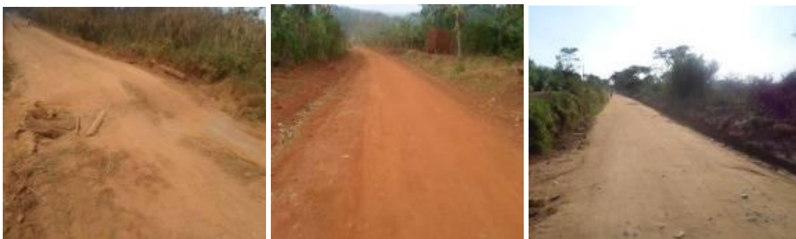
Mubende District: Left: Section at km 13+700 in need of replacement of drainage structures; Centre: Graded section of Kitovu – Lwabusana at km 2+100; Right: Graded section of Musozi – Kalamba road at km 9+600
