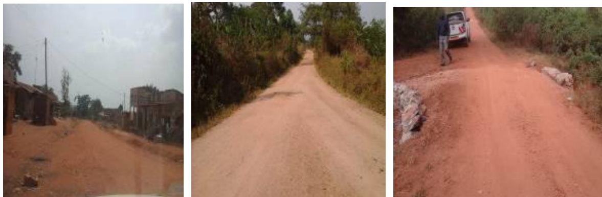
Luwero District: Left: Graded section of Buzibwera-Makangonyigo road; Centre: Gravelled section along Bukembya-Nakusubyaki road; Right: Culvert structure without wing walls at km 5+00 along Bukembya-Nakusubyaki road
