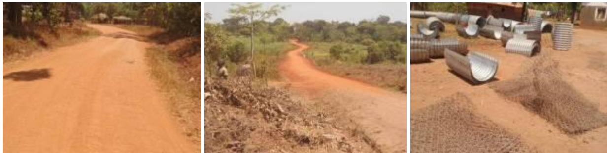
Kamuli district: Left: A completed section on Musunu-Bulukaire-Nakabala road; Center: A swamp raised and gravelled section on Bukyonza-Bukozi road; Right: Armco culvert material and gabion meshes supplied by MoWT one of the project sites
