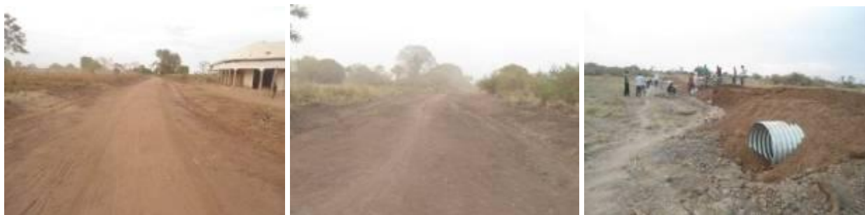
Serere County, Serere: Left: A dusty graded section of Sapir-Ojara-Amakio road in Olio sub county; Center: A bush cleared section at Km 2+200 on Kampala-Kachinga road in Kyere sub county; Right: Swamp raising after culvert installation with gravel at Km 3+400 on Angole-Omagoro-Kachinga road in Kyere sub county
