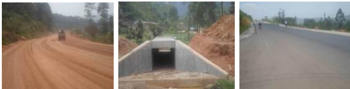
Left: A completed improved sub-base at km 152+312; Centre: A completed box culvert at 4km from Katuna; Right: A completed section of the road at km 100+300
