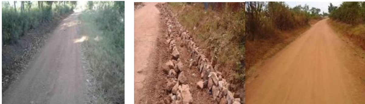
Masaka UNRA Station: Left: Completed section Ndegeya -PTC Access road; Center: Incomplete stone pitching works at km 26+300 along Lukaya-Miwula-Kagorogoro road in Mivula trading centre; Right: Graveled section at km 1+700 along Lukaya-Miwula-Kagorogoro road
