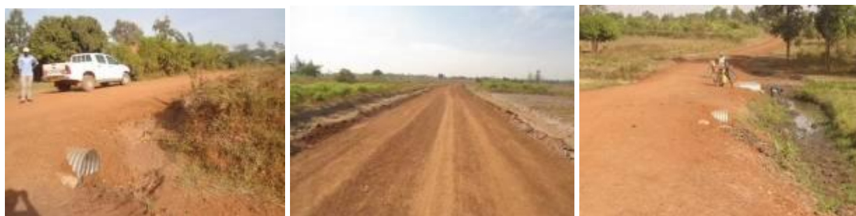
Left: An access culvert and a gravelled section on Mudimbu- Highland road in Mazimasa sub county; Center: A 300m raised swamp section with side drains of 2m width at Km 1+200 on Mazimasa B - Guli road; Right: A raised swampy section along Kachonga-Bufujja road at Km 1+400 in Kachonga sub county
