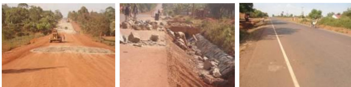
Left: A section still under construction at Km 9+000; Centre: Stone pitching works at km 6+186; Right: A trial marked section at km 24+990
