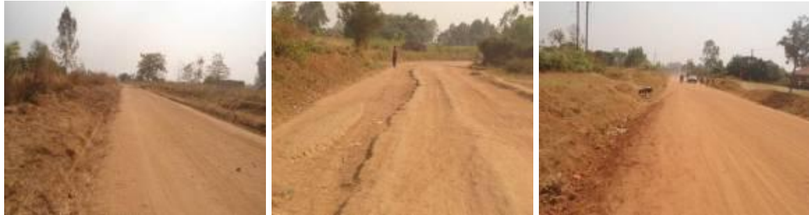
Arua UNRA Station: Left; Graded section at Km 4+400 along Arua-Biliaffe-Otrevu road: Centre; A damaged section at km 7+600 along arua-Girigiri-Ovision road: Right; Graveled section at Km 0+000 along Manibe-Wandi road
