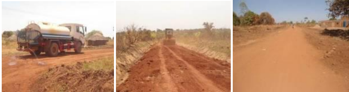
Gulu District: Left and Centre, Lalogi – Bario road - Gravelling activities of watering and spreading; Right: Laroo-Pageya road- Bush cleared section
