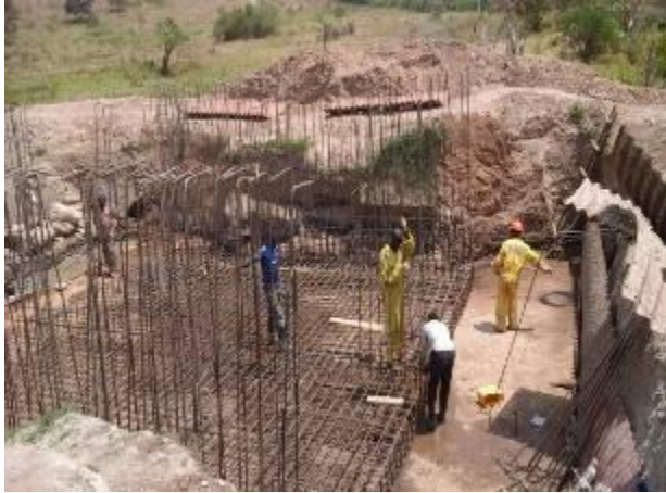
Left: Fixing of reinforcement bars for the bridge and Right: Construction material on site
