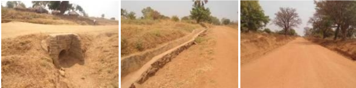
Arua UNRA Station: Left; A concrete culvert installed at km 2+500: Centre; A stone pitched side drain at km27+500: Right; A Front view of the road at km 38+000
