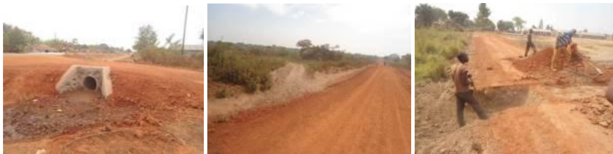
Left: A 600mm diameter access culvert with a head wall at the beginning of the road; Center: A gravelled section with a mitre drain; Right: Excavating for a culvert line along the project road
