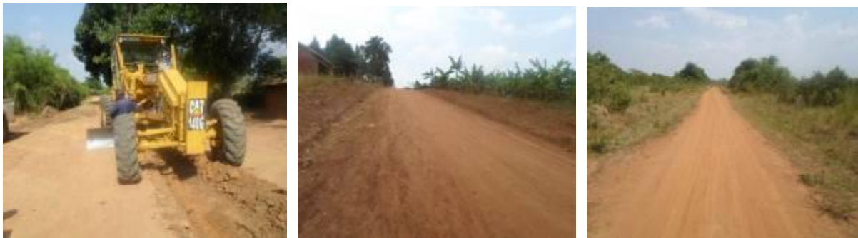
Kiboga District: Left: Grading using a hired grade along Bulyankuyege - Kibisi – Kigwanya road; Centre: Graded section awaiting graveling along Jokero - Nakasozi – Kibulala road; Right: Completed section of Kajjere - Nakasagazi – Mulagi road
