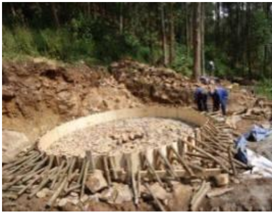
L-R: Foundation works of 40m 3 concrete reservoir; Retention wall at intake on Rushoroza Hill
