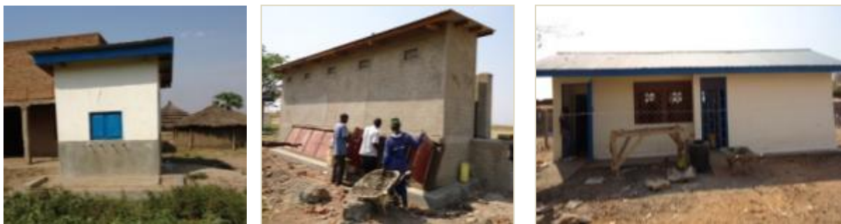
L-R: Public water kiosk in Patongo TC; Ecosan toilet in Moo Dege P/S; public water borne toilet in Patongo Taxi Park
