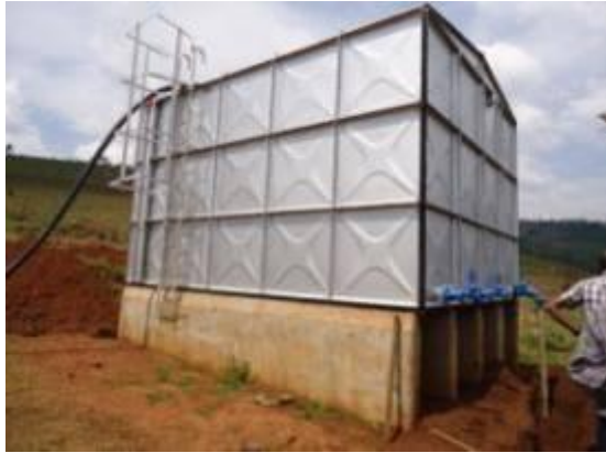
L-R: 5m 3 institutional reservoir tank and 50m 3 main reservoir tank on Rushoroza Hill
