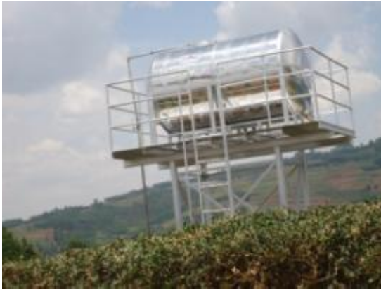
L-R: 5m 3 institutional reservoir tank and 50m 3 main reservoir tank on Rushoroza Hill
