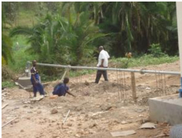
L-R: Anchoring of pumping main; 120m 3 twin reservoir tank both in Kijongo sub-county
