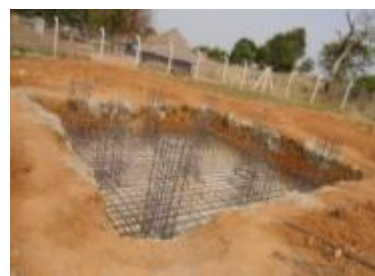
L-R: Water office; pump house & generator house; foundation steel works for reservoir tank all in Patongo Town Council
