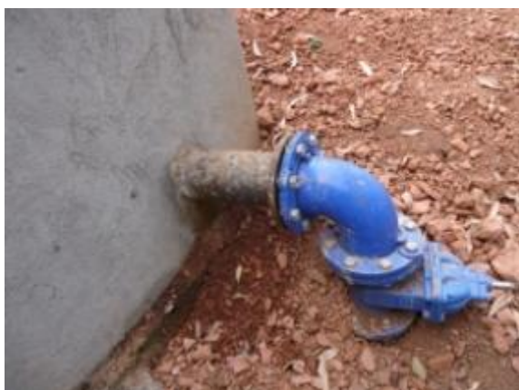
L-R: Leakage on 8m 3 BPT; 250m 3 reservoir tank in Lyantonde Town Council
