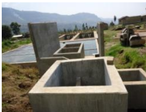
Left: Completed retention weir in Bupoto sub-county; Right: Inlet chamber, alum dosing unit, coagulation and flocculation chambers, and sedimentation tank in Bukokho sub-county
