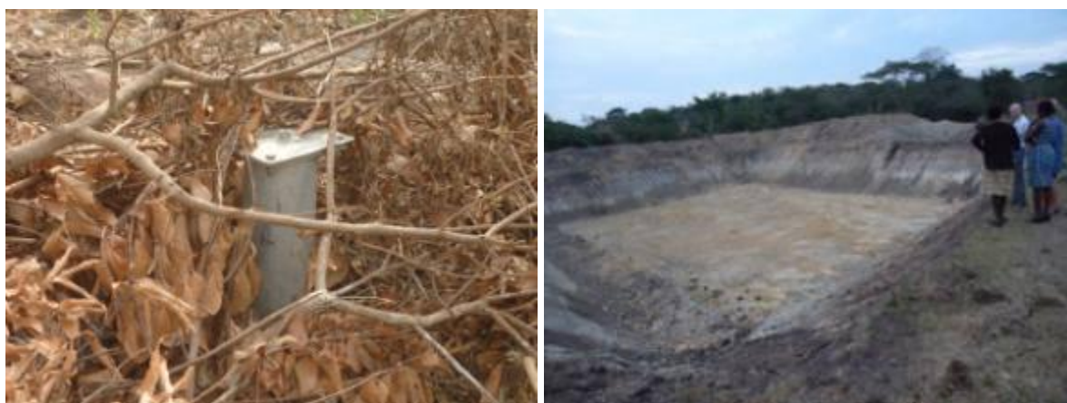
L-R: Drilled borehole at Ntungamo village, Ntungamo parish Kabaringa sub-county; Rwemutongole village, Kawawa parish; 10,000m 3 valley tank in Manyogaseka (sub-county Mubende district)
