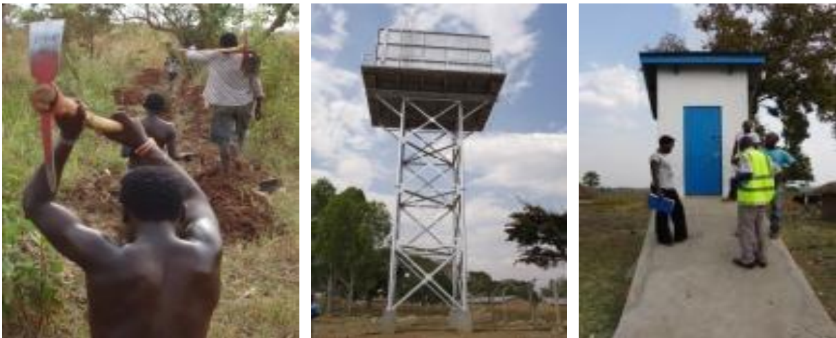
L-R: Trenching transmission mains; 100m 3 reservoir tank; Household ecosan toilet all in Lakwana sub-county
