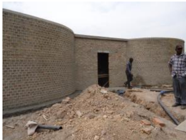
L-R: Anchoring of pumping main; 120m 3 twin reservoir tank both in Kijongo sub-county
