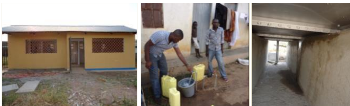
Left: Water borne public toilet in Ocheri town; Centre: Functional household private tap in Ocheri town; Right: Leakage underneath the reservoir tank on Ocheri hill
