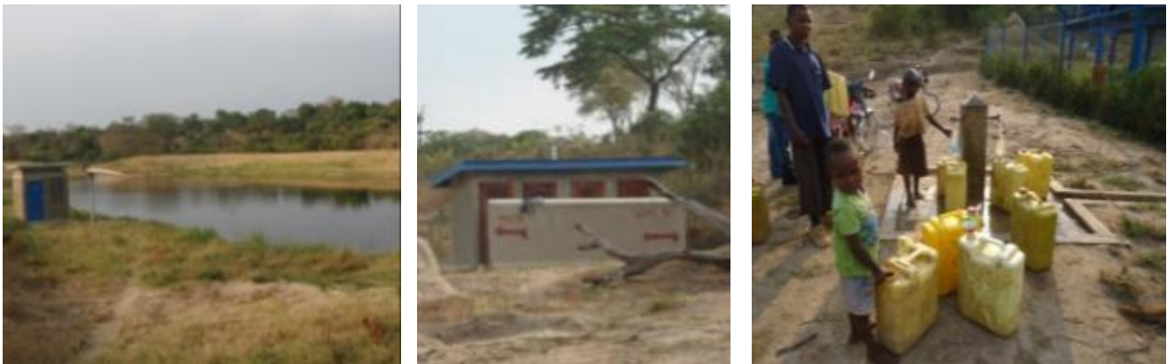
L-R: Pump house & Valley Tank; Public VIP latrine; Public water stand post in Ruyonza sub-county
