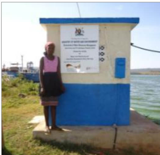
Completed protective house
