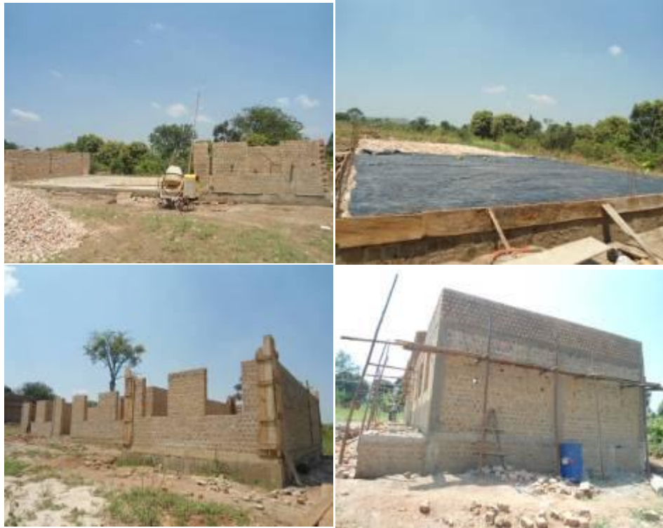
From Top L-R: The BCP workshop at walling level, the Capentry workshop at ground slab level, the administration block at ring bim level, and the two classroom block at roofing level at Bamunanika Technical Institute
