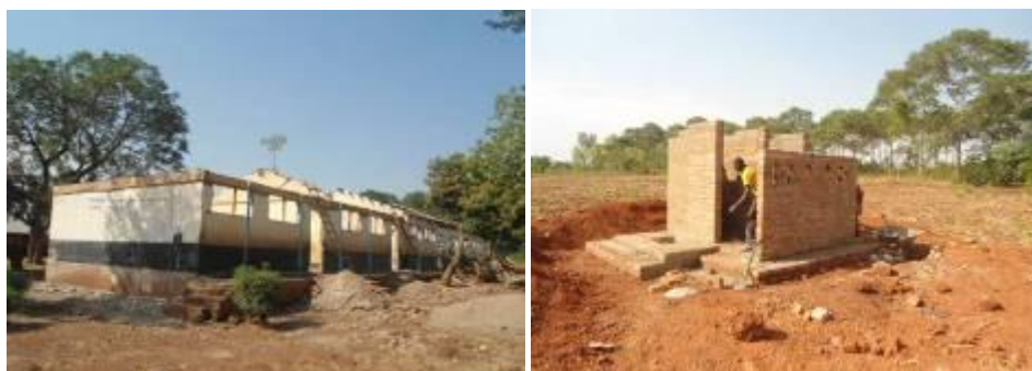
L-R: Rehabilitation of a four classroom block with an office and construction of a two stance lined VIP latrine at Waluwerere P/S
