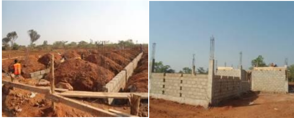
L-R: A boys' dormitory at plinth wall level and a girls' dormitory at walling on one side and first floor slab on the other at Lira UTC.
