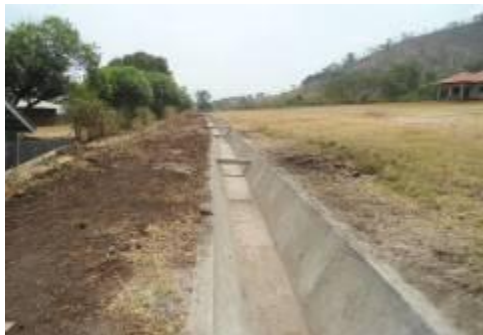
The water channel diverting water from Kasese hills from entering the school and the two unit science laboratory completed at Kasese S.S.
