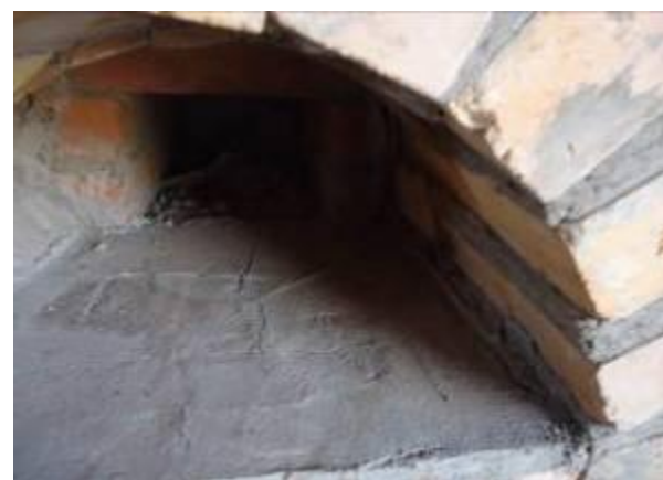
Cracks on the newly constructed institutional stove at Lango College
