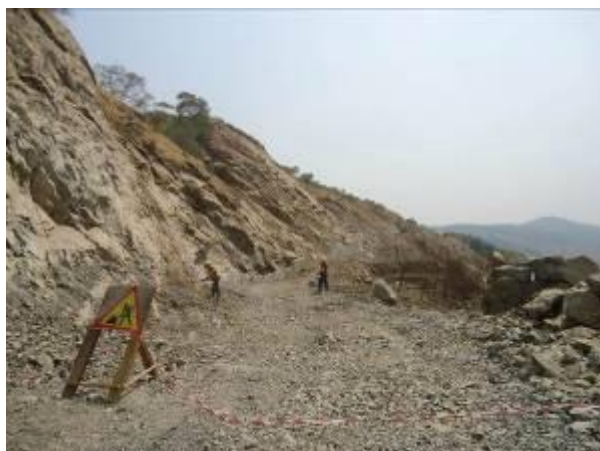
Left -Right: Preparation for blasting of the rock to create access road; Road network to Field Development Area being developed
