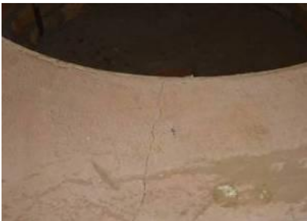
Cracks on the newly constructed institutional stove at Lango College
