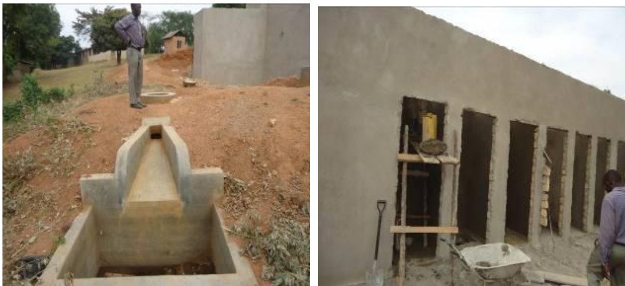
Left: Component of the Bio latrine. Right: plastering works on the bio latrine at Kitagobwa SS, Ngando sub county, Butambala district
