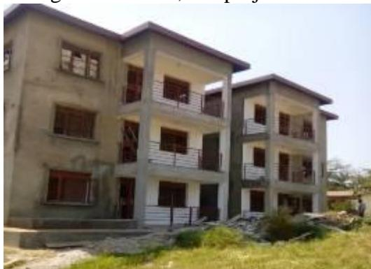
The facility was roofed and plastered, outstanding works included painting, floor works, electrical, plumbing and external works (landscaping). The hospital noted that the contractor was willing to continue and have works completed upon availability of the balance. There is fear that the hospital will not have enough money to clear any more certificates
