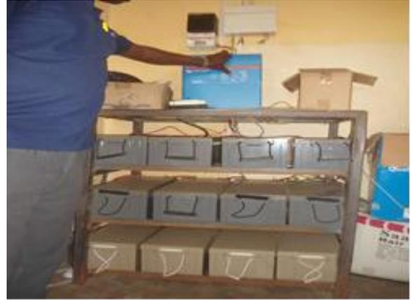
**Left: Solar Panels installed and right: Staff showing the weak batteries and burnt charger control at Yumbe Hospital**
