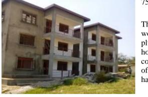
The facility was roofed and plastered, outstanding works included painting, floor works, electrical, plumbing and external works (landscaping). The hospital noted that the contractor was willing to continue and have works completed upon availability of the balance. There is fear that the hospital will not have enough money to clear any more certificates
