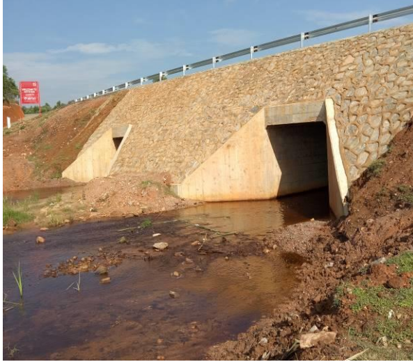
A box culvert at 1+500 on Kashenyi–Mitooma (11.53Km)
