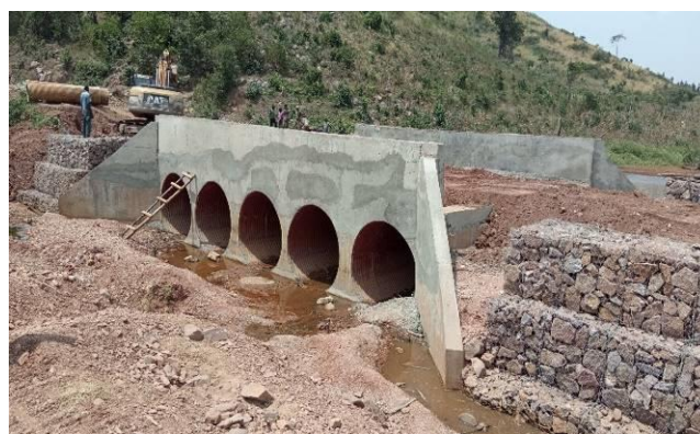
Bambala bridge: Construction of a five cell of 2.1m diameter ARMCO culvert crossing in Kyankwanzi District
