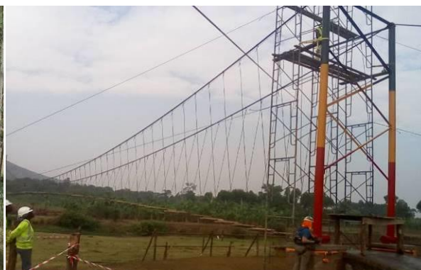
Erection of cables at the Tongole cable bridge site in Manafwa District in progress
