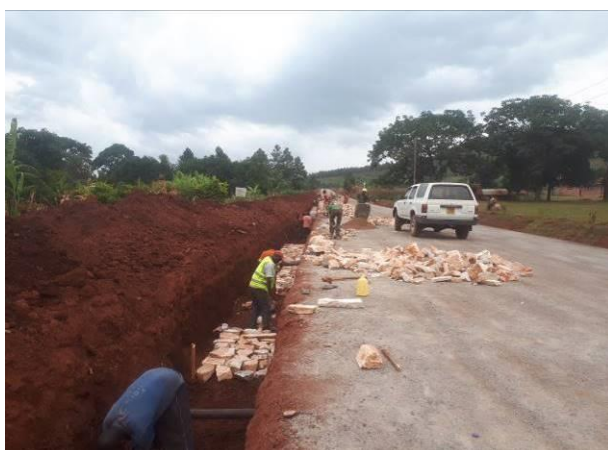
Stone pitching works along the access road to Busoga College Mwiri in Jinja in progress
