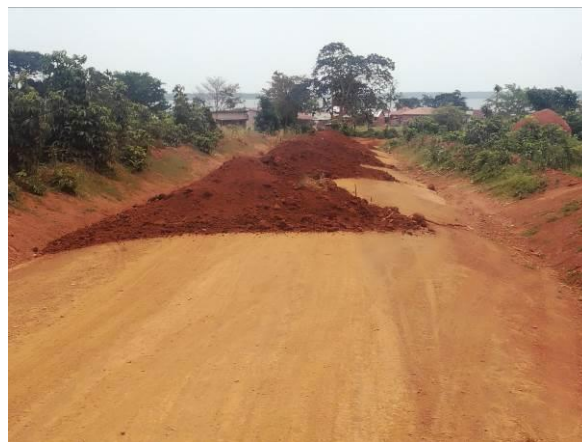
Graving of Kikonge – Katuba road (9km) road in Buwoya Sub County Left: Km 0+300; Right: Km 5+000
