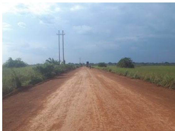
A swamp section Amii - Kidilan - Atura-Aber-Atapara road that was raised and widened during mechanized maintenance under the term maintenance contract in Q2 FY2018/19
