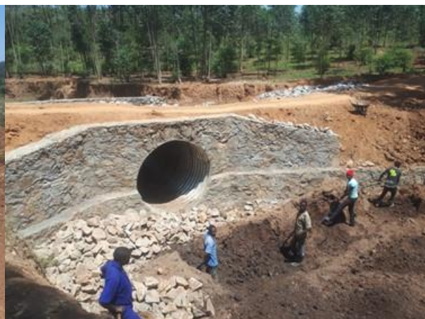
Installation of a 1.2m diameter armco culvert crossing on Mulatsi-Bukiende Road (7.1km) under periodic maintenance
