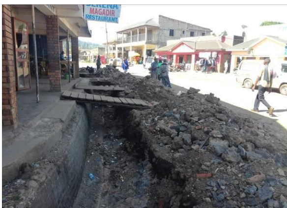
Excavation for the side drain on Bishop Kivengere road (0.3km) at Km 0+000
