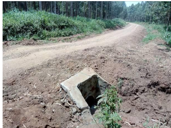
A culvert installed at 9+900 along Butambuka-Guwe-Kitwala Road
