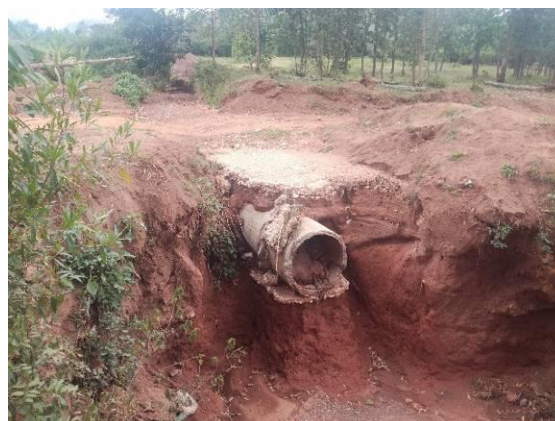
Omungyenye-Nyanga-Ruyonza road (10.3km): A damaged drift at Km1+300 at a point with a seasonal stream
