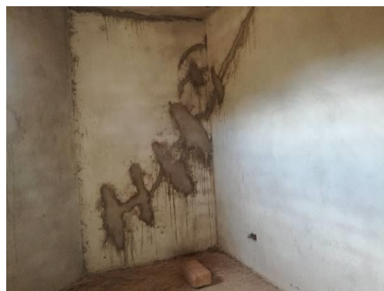
Repair work on the cracks in the walls caused by settlement at the Katuna OSBP
