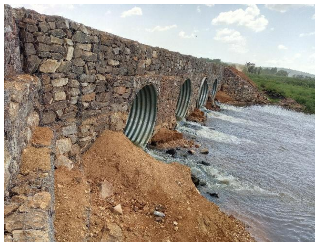
Emergency works of swamp raising along Mawale-Danza-Kakiri Road at 13+800 from Mawale
