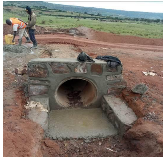
Culvert installation works at 15+500 along Isingiro-Rugaga road
