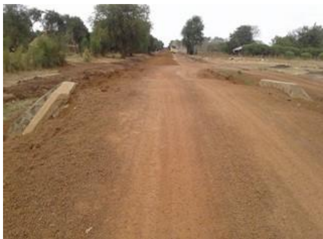
Ongoing gravelling works along Nabilatuk – Angatun Road (25.6km)
