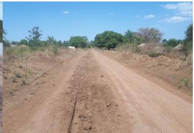
A section of Adwoki-Bata Road (10km) that had deteriorated because it was not compacted during RMeM in Q2
