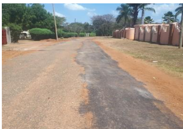
Kyoga Avenue (1.3 km) was undergoing patching works under periodic maintenance
