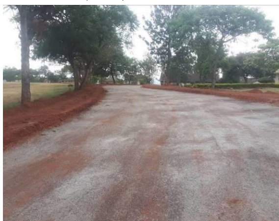
Primed section along the access road to Busoga College Mwiri in Jinja
