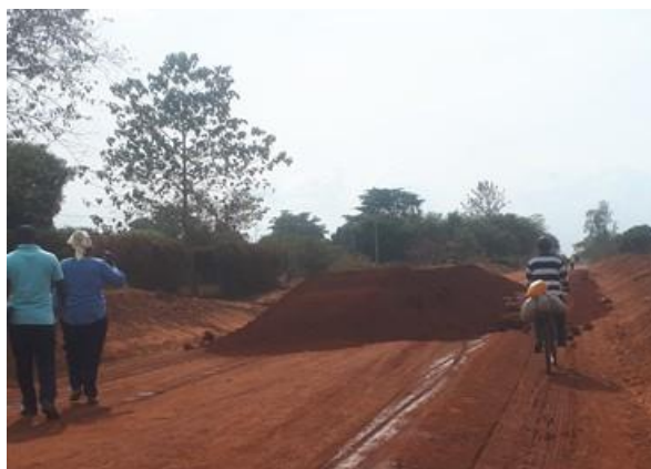
Ongoing gravelling works on Lira-Aduku-Apac road that was under mechanized maintenance using term maintenance contract
