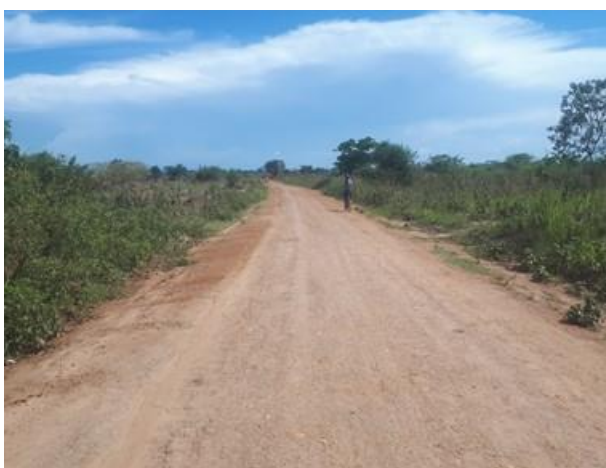
A section of Amolator-Acamulum Road (4.4km) after RMeM in Q2. The road lacks proper drainage structures
