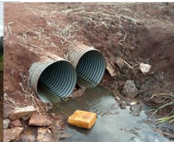
Armco culverts installed at Kinabi-Karim swamp
