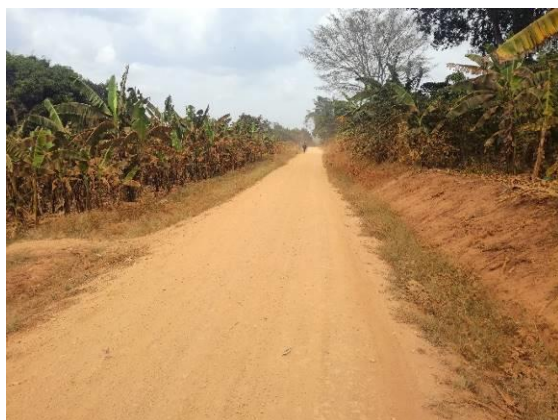
Nabutongwa-Kalungu road (3.5km): A well graded road section with over grown grass in the side drains at Km 2+800
