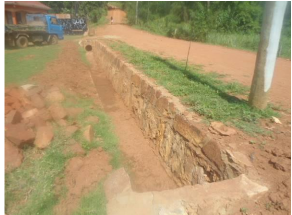
A stone pitched drain on Suula Ebikomo swamp
