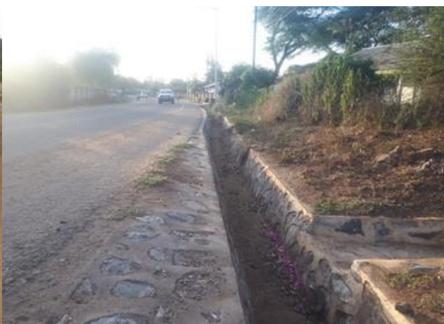
Stone pitching works on Moroto Municipal roads under RMeM in Q1
