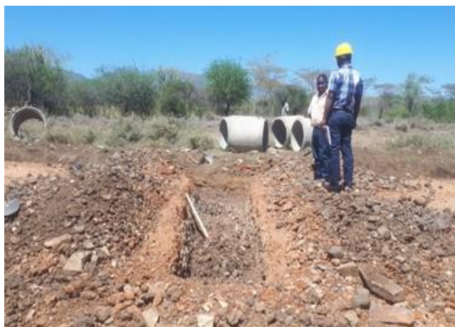
Culvert installation was ongoing along Moroto-Lokitanyala Road during the of 5 th cycle of term maintenance
