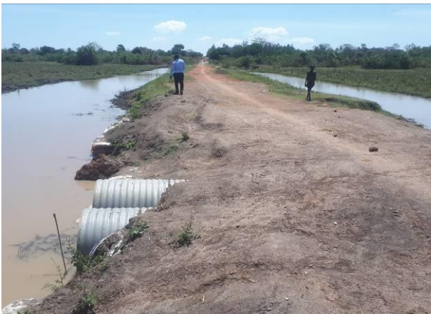
A 1.2km swamp section of Apenyoweo-Regprego road that was raised and installed Armco culverts in Q2
