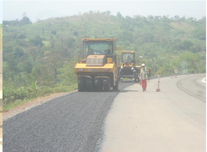
Laying of first seal at km 63+045 on Kyenjojo-Kabwoya Road
