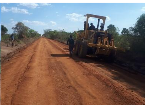
Gravelling works at km 8+400 along Bar junction-Corner Amach Road
