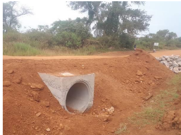
Soroti-Serere Road (27km)-900mm diameter encased culvert installed at km 22+450 in Q2 FY 2018/19; pending construction of end structures
