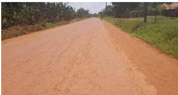
Stabilised base awaiting the first seal along Kayunga–Nabuganyi Road
