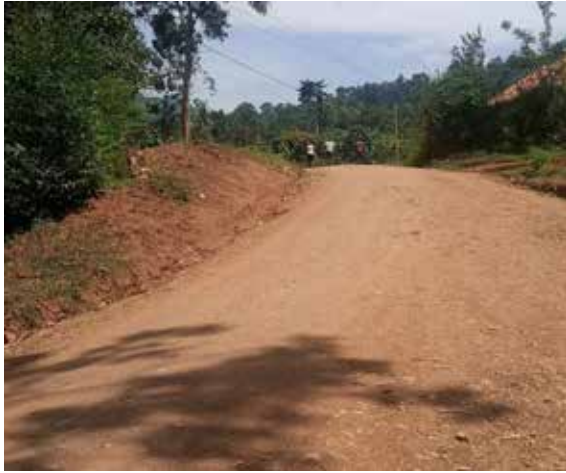
A well graveled section of Buwangani-Butooto Road at Km 0+400
