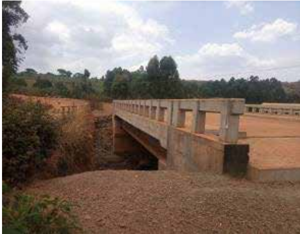
A completed bridge across Atari River at 2+370 on Kapchorwa –Suam Road
