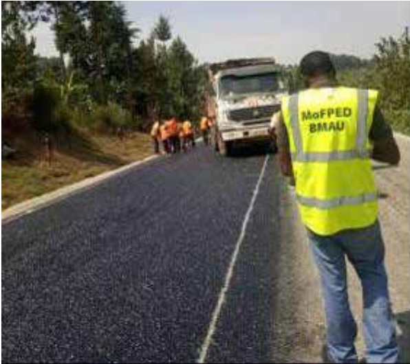
Laying of asphalt on Namunsi Sironko Road at 54+495
