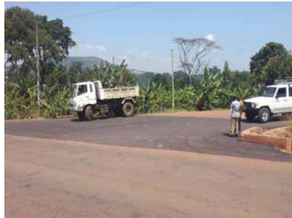
The asphalt surfacing at the Jinja –Iganga Highway
