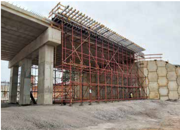
Kisaasi interchange on the Kampala Northern Bypass
