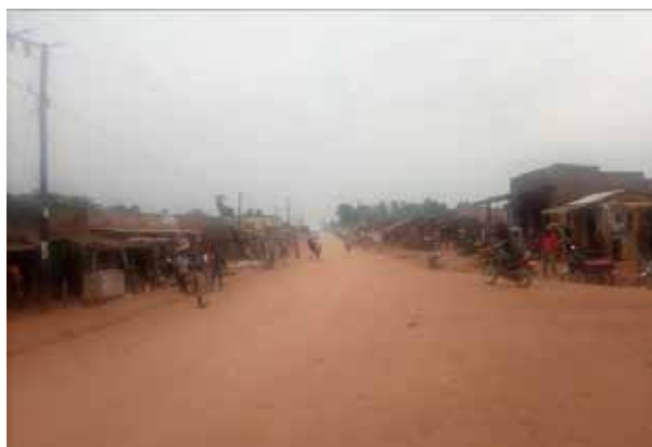
A section of Paidha-Anyavu Road at 9+100 at Nyapea
