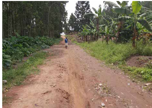
Nyakabare-kaberebere-Kitwe Road (8km) after routine mechanised maintenance in Q1
