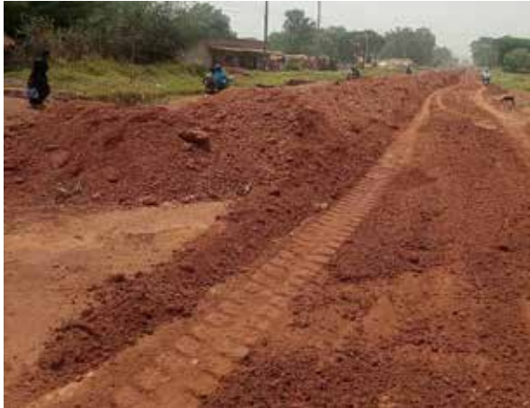
Dumping and spreading of gravel on Tororo-Nagongera Road
