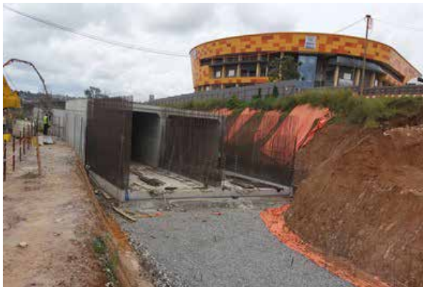
Nsambya Underpass (part of Kampala Flyover) works in progress
