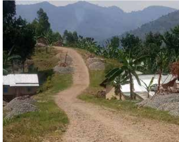
A rocky section of Buwangani-Sikunge Road at Km 2+300
