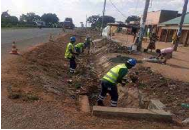
Cleaning of side drains at 2+000 on Soroti-Dokolo-Lira-Kamdini (189.4km)- Lot 2
