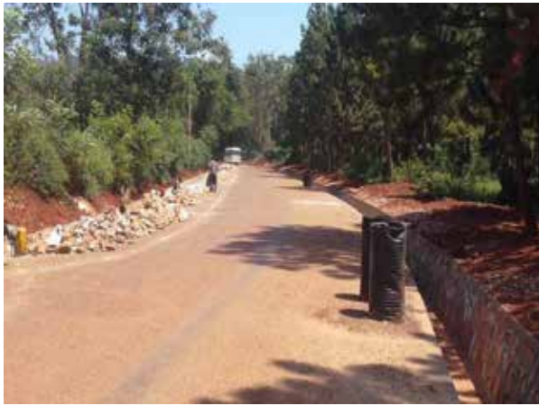
Stone pitching works at km 0+300
