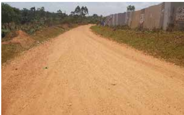
Gravelled section along Kisuule–Nakaseke–Kapeeka Road
