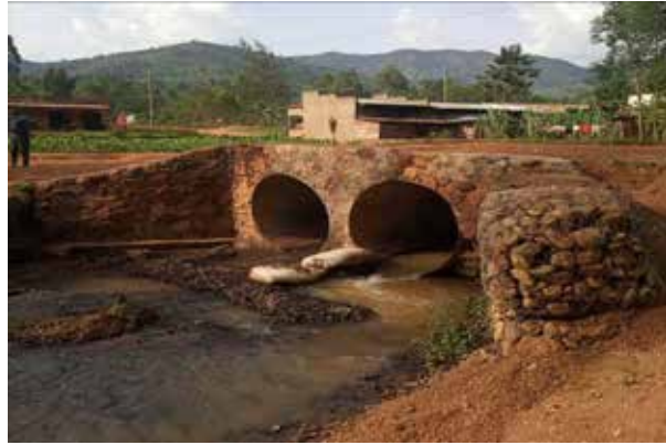
Installed Armco culverts of 1.8m diameter at km 3+300 on Mabale-Wakamala Road
