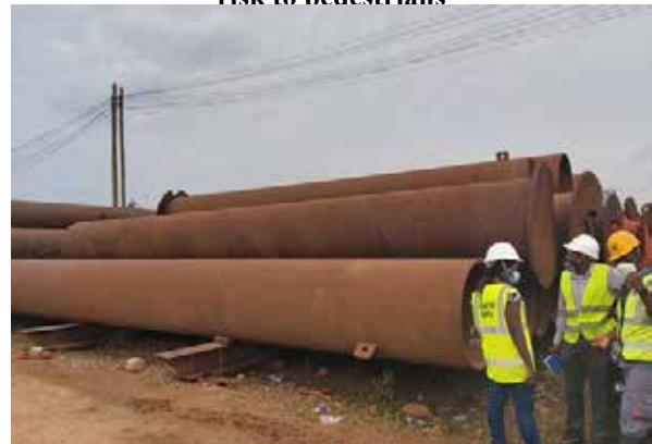
Mobilised piles for the Kampala Flyover Project
