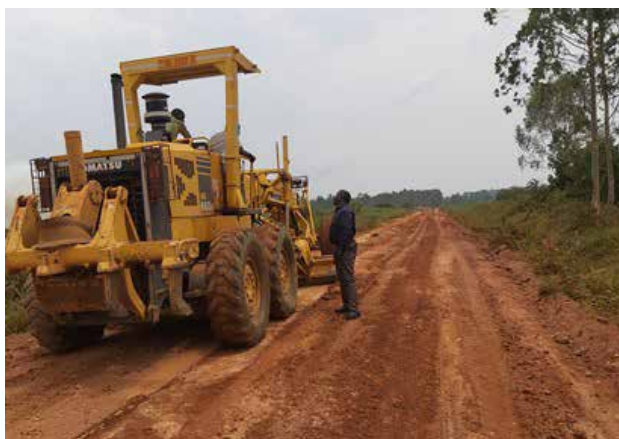
Gravelling works of Kinyika swamp at km 4+800 along Kayabwe-Bukasa-Muyanga Road
