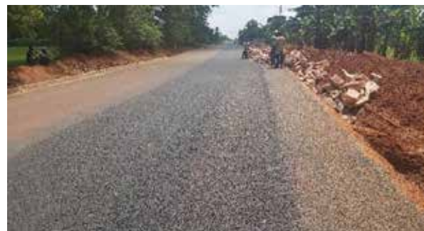
Finished road with side drain construction ongoing along Kayunga–Nabuganyi Road
