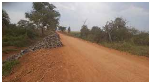
Gravelled section of Ihunga–Bulyamusenyu Road with mobilised materials for gabion works
