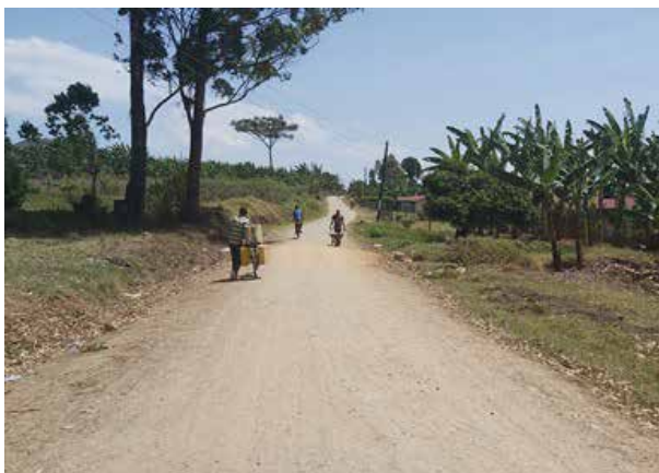
Rwenkumba–Mukonomura-Buhara Road (5.7 km) after the rehabilitation works
