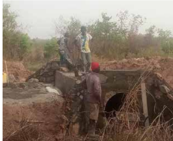
Ongoing culvert headwall construction works at 6+000 on Inde-Okollo Road
