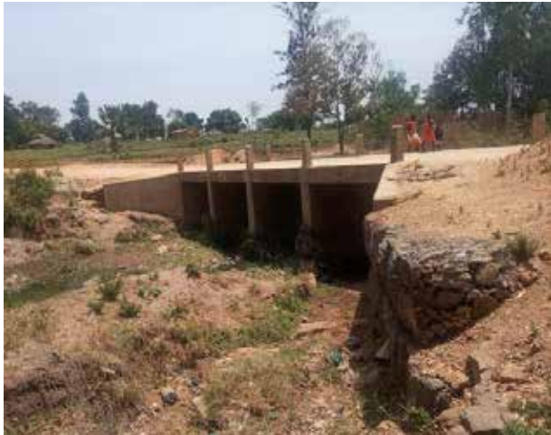
Osu Box Culvert Bridge on Ochiba–Ombakyi Road
