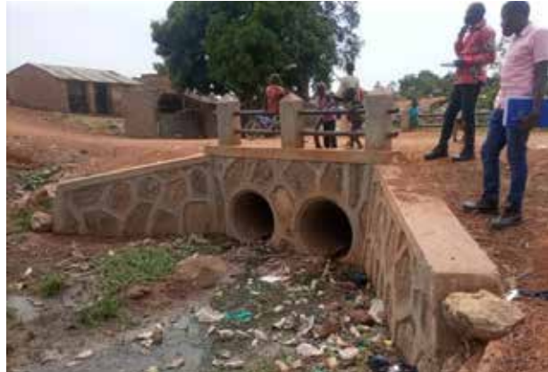
A two lines bridge culvert, 900m, on Amin Road
