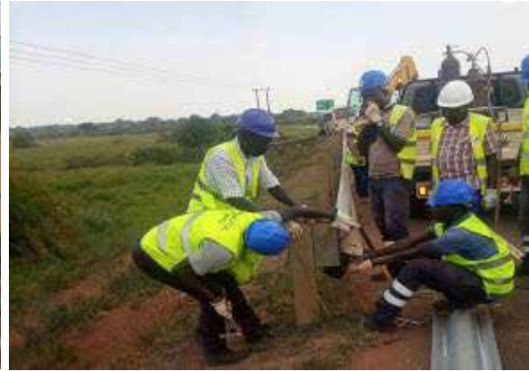
Replacing of a guard rail at 19+000 on Soroti-Dokolo-Lira-Kamdini (189.4km)-Lot 2
