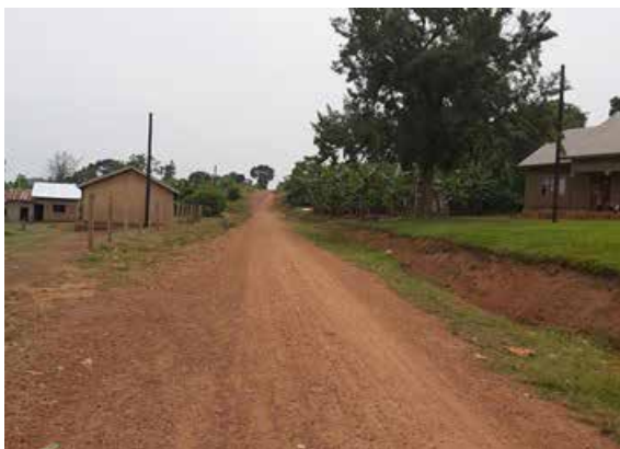
A graveled section of Masagala-Bunyenyne Loop Road (4.3km), works done under the rehabilitation contract
