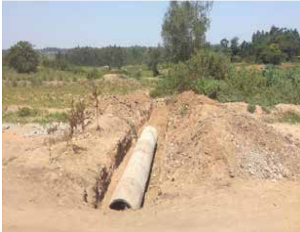
Ongoing culvert installation at Km 2+600 along Soko Market–Pei Road
