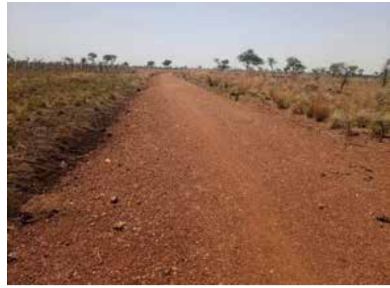
A well graded and gravelled section of Okoboi-Akulony-Acinga Road
