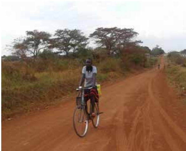
A section of Kitgum-Lukung Road at 18+000
