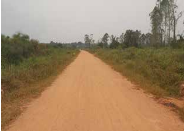
Timuna-Lugogo Road (8.0km) after the rehabilitation works
