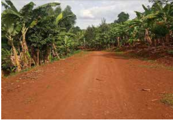
A well opened and formed ungravelled section at 1+800 on Mabale-Wakamala Road
