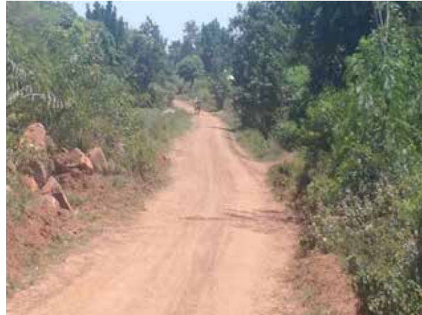
Well graded section of Abweli-Corner Bar-Nagongera NTC at Km 1+000
