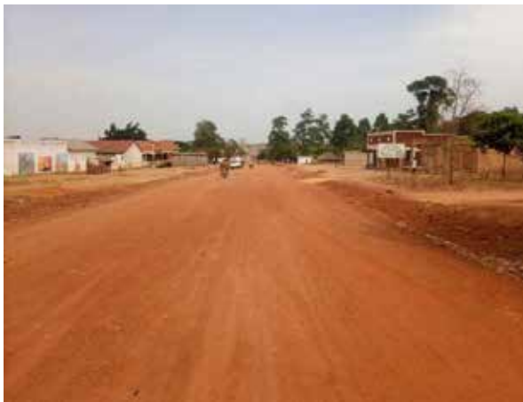
A section of Appa road at 0+500
