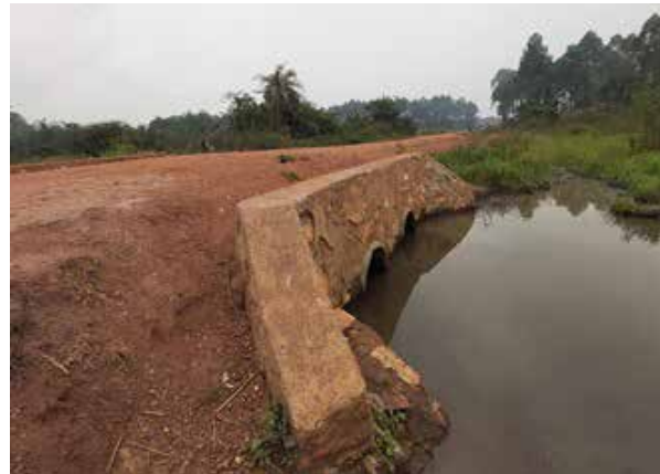
One of the 600mm diameter concrete culverts installed on Kyampisi–Sombwe–Kyambogo Road
