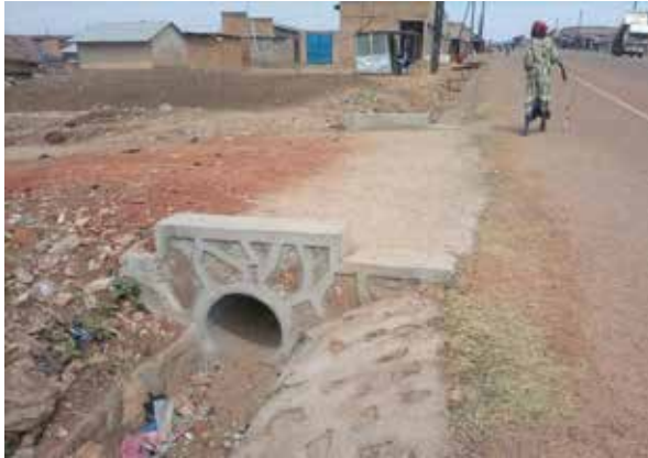
An access culvert on Amin-Ali-Kenyi Road
