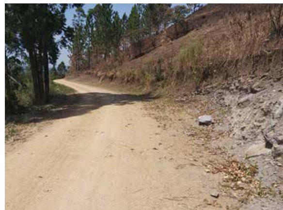
Mukonomura-Kasindikwa (2.0km) Road was rehabilitated under the contract
