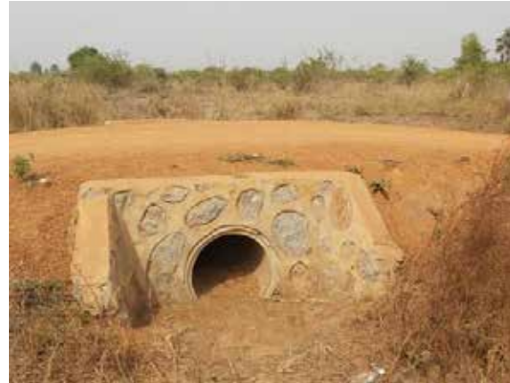
600mm diameter concrete culvert with end structures installed on Nakitoma-Nabiswera Road
