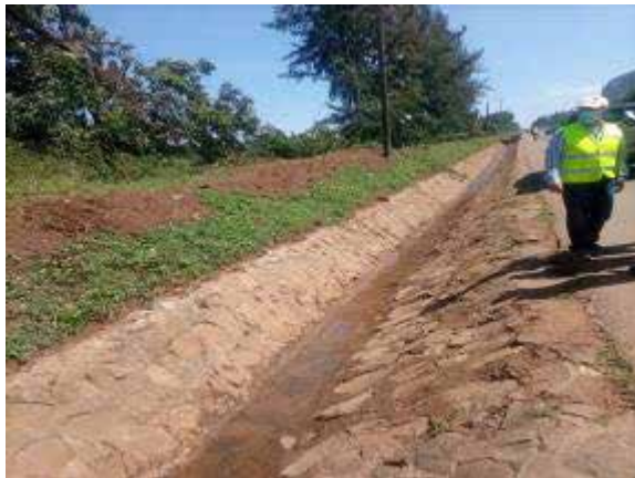
A cleaned side drain at 0+600 on Tororo-Mbale-Soroti Road (150.8km) – Lot 1
