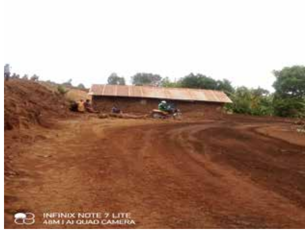
A PAP awaiting compensation at 41+000 on Kapchorwa-Suam Road
