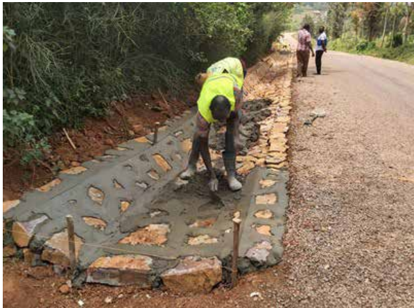
Construction of side drains using stone pitched masonry along Kijjukizo Road
