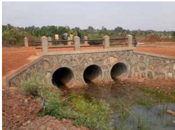
Three lines of 1200mm culvert Bridge on Harizona Road
