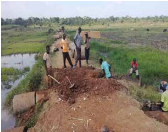
Excavation for culvert installation at the swamp crossing along Busembatita-Lumbuye Road
