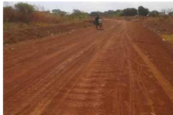
A section of Pajule-Pader-Konkwich Road at 14+100
