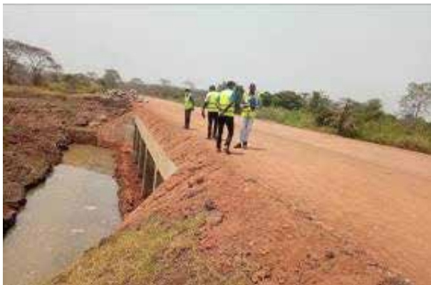
Awa Bridge on Pakwach - Inde -Ocoko Road
