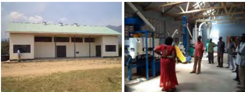
Completed but non-functional coffee huller facility in Kichwamba sub-county, Kabarole district; top right: Installed machinery for maize mill in Myene sub-county, Oyam district
