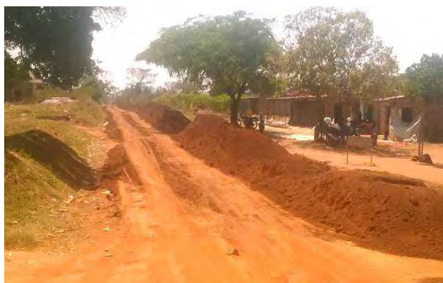
Gravelling works on going along Ikooba- Ntoma Road
