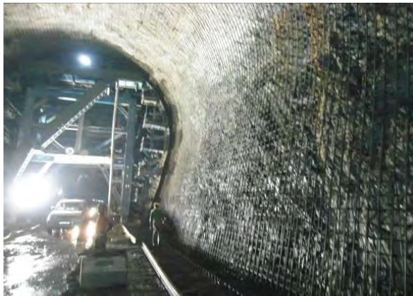
L-R: Completed excavations and ongoing steel works in preparation for concreting in the Tail Race Tunnel (TRT) at Karuma HPP in Nwoya/Kiryandongo district
