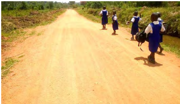
Graded section along Kalule-Bowa-Nakaseke – Kiwoko Road
