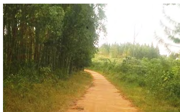
Kyakatwanga-Kakwaku-Kisenge road under routine manual maintenance
