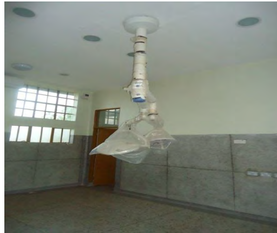
Left: Poor quality terrazzo and misfitted cabinet doors in the theatre at Nakaseke GH; Right: Poorly fitted theatre light at Atiak HC IV, Amuru District
