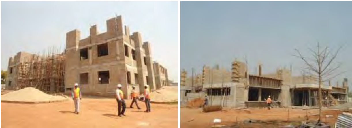
L-R: The agricultural block at 45% and multi-functional laboratory block at 29% progress at Gulu University
