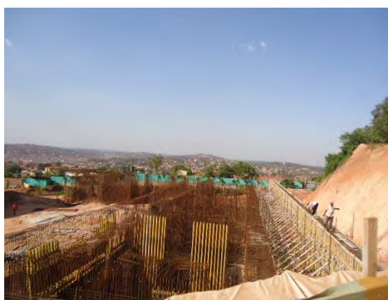
On-going construction works for the bunker at Uganda Cancer Institute
