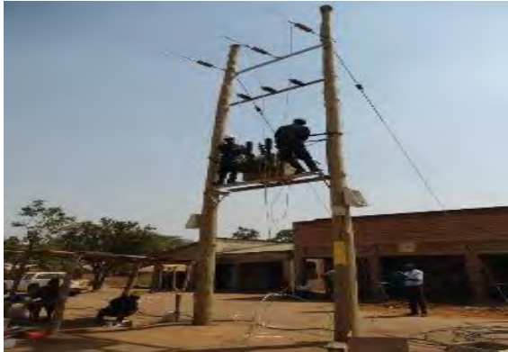
L-R: Workers of C&G Installing a transformer at Acuta Trading Center (Oyam District), Completed work on the Aduku-Inomo 33kV distribution line in Anac District
