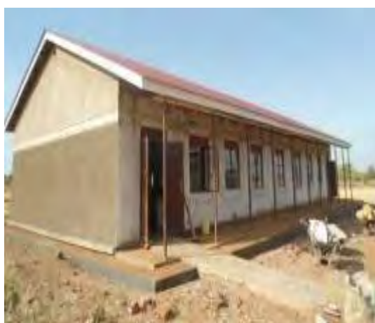
A science block completed at Patong S.S in Agago district
