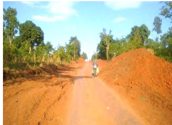
Bush clearing along Bukulula–Kalungu Road – a pilot project for full gravelling
