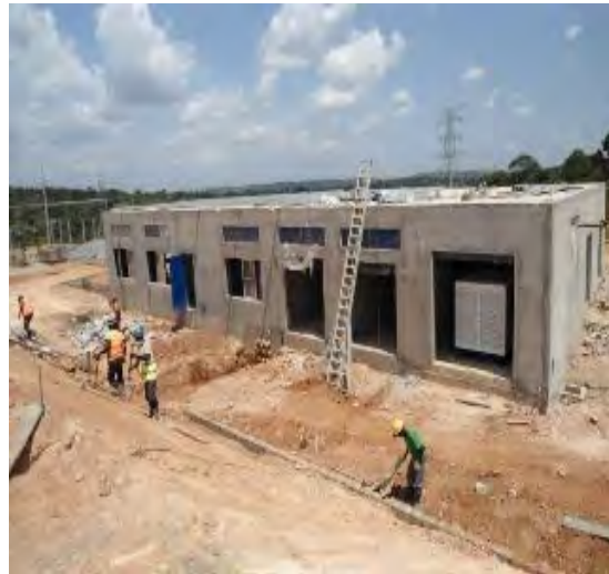
L-R: Ongoing stone pitching works for slope protection; Civil works on the 220kV plant house in Masaka substation
