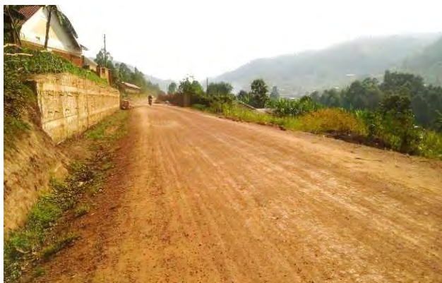
Stabilised gravel base for Bukinda-Highland tarmac road awaiting surfacing
