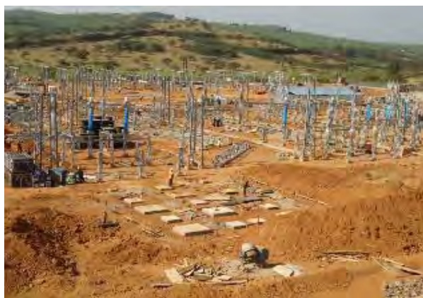
L-R: On-going equipment erection at the 132/220kV New Mbararara substation; On-going civil and electro-mechanical works at Mirama Hills substation
