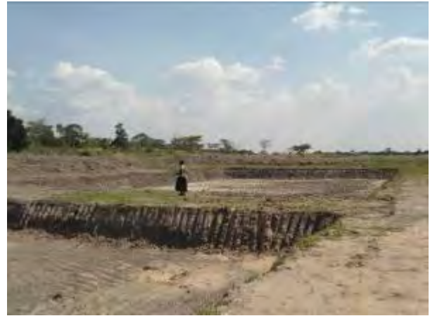
Two of the 10 fish ponds that were excavated on Ms. Nakaggo's farm in Kagalama village, Luwero district
