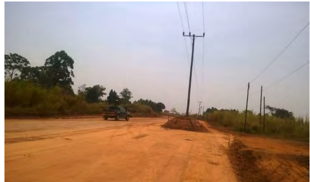
Power lines within the road prism yet to be relocated along the Kabwoya-Kyenjojo road
