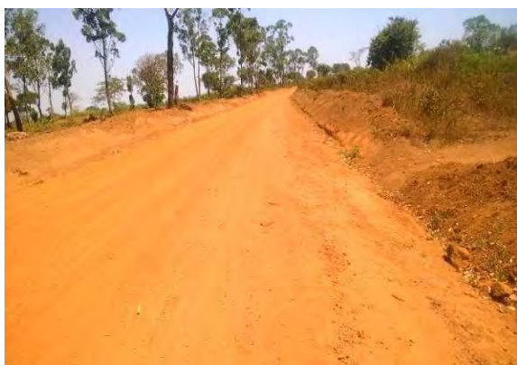
A gravelled section of Ihungu-Bulyamusenyu Road (42km)
