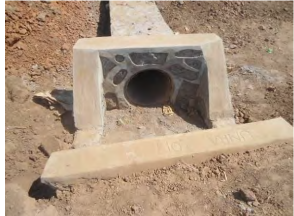
Installed culvert pending backfilling along Aduku-Nambieso Road
