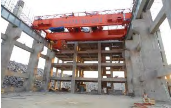
L-R: Newly installed Over Head Electric Crane in the machine assembly room; Repaired crack on part of the dam tailrace structure at Isimba HPP
