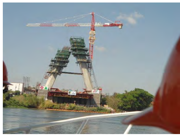
Construction of Pylon 2 of the New Nile Bridge in Njeru town
