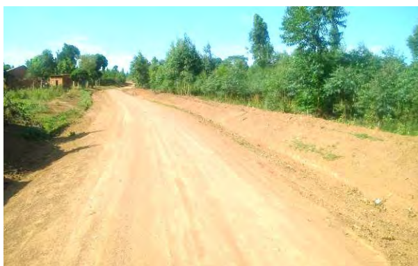
A well graded Degeya-Nuo Kabale Town Board Road
