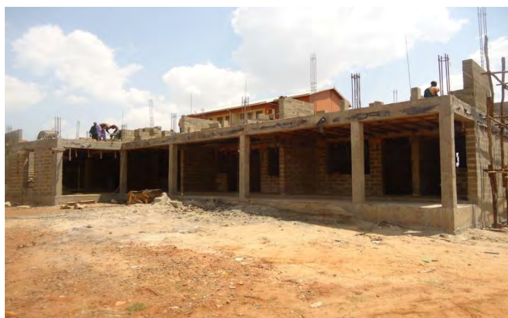
On-going construction works for staff houses at Gulu RRH
