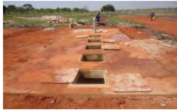
L-R: Excavation for the Sludge Drying Bed; Anaerobic Baffled Reactor tank of Kayunga Faecal sludge in Kavunga district
