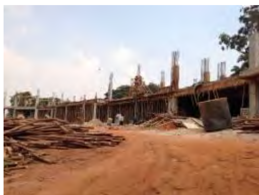
Construction works for Central Lecture Block at Kyambogo University
