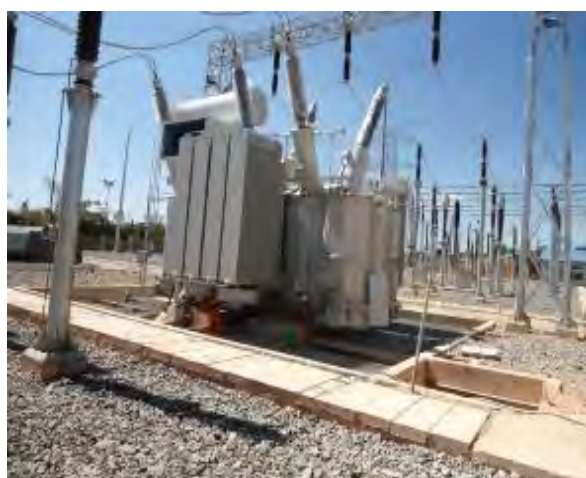
L-R: Installed 250MVA transformer at the 220kV section; Ongoing external works on the partially completed 220kV plant house at Kawanda sub-station
