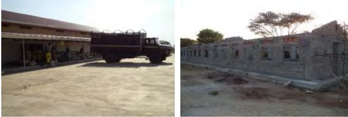
Left: Workers loading sacks of sunflower seeds from the store onto a prison truck in Namalu Prison: Right: Girls' dormitory under construction at Moroto High School. Moroto District
