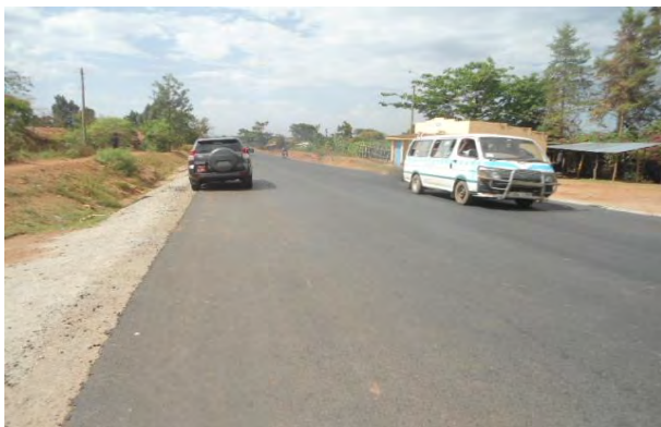
A trial asphalt section along Namunsi-Kapchorwa Road
