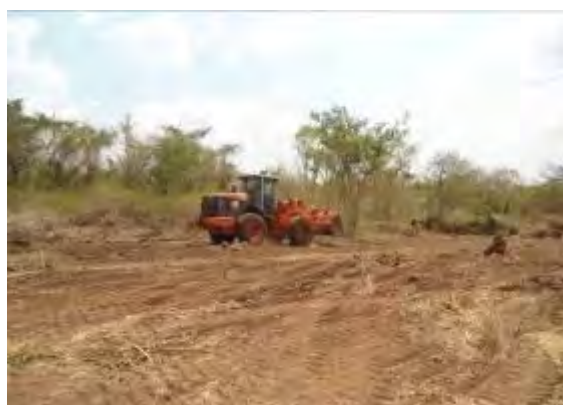
Bush clearing was ongoing at AMFRI FARM in Nakaseke district
