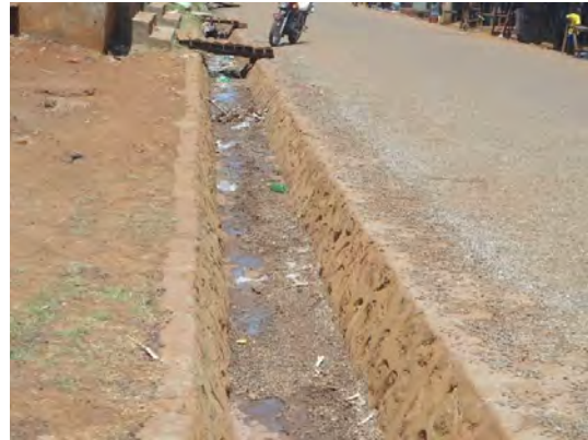
Stone pitched lined drain of Moi Road in Kapchorwa Town Council
