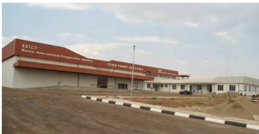
Completed civil works at the Soroti Fruit Factory in Arapai, Soroti district
