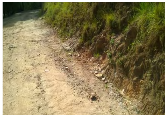
Rocky section requiring a bulldozer along Bukinda-Kahindo-Masiba Road
