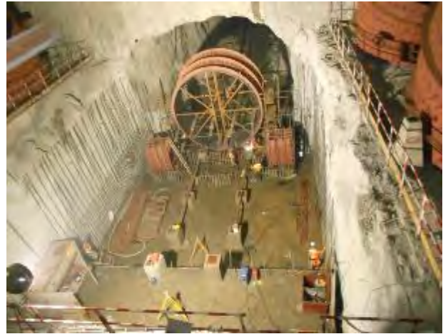
L-R: Civil works at the dam structure; Civil and electromechanical works in one of the turbine pits at Karuma HPP in Nwoya/Kiryandongo district
