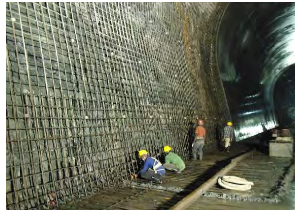
L-R: Completed excavations and ongoing steel works in preparation for concreting in the Tail Race Tunnel (TRT) at Karuma HPP in Nwoya/Kiryandongo district
