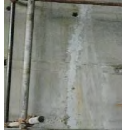
L-R: Newly installed Over Head Electric Crane in the machine assembly room; Repaired crack on part of the dam tailrace structure at Isimba HPP
