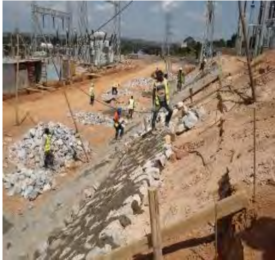
L-R: Ongoing stone pitching works for slope protection; Civil works on the 220kV plant house in Masaka substation
