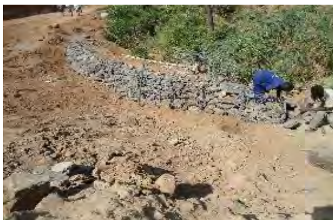
L-R: Laying of gabions on the power house access road; Part of the contractors camp at Nyagak III in Zombo district
