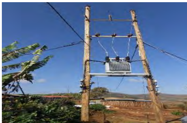
L-R: Installed transformer on the completed 33kV Kapchorwa-Bukwo-Suam line, Poles erected on the Ociba Community share scheme in Arua district
