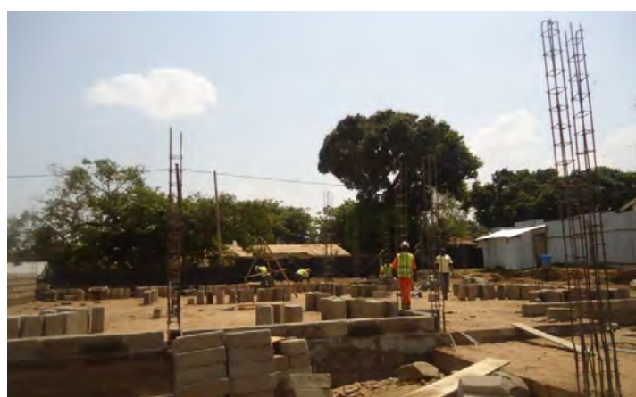
On-going construction works for the drug store at Arua RRH
