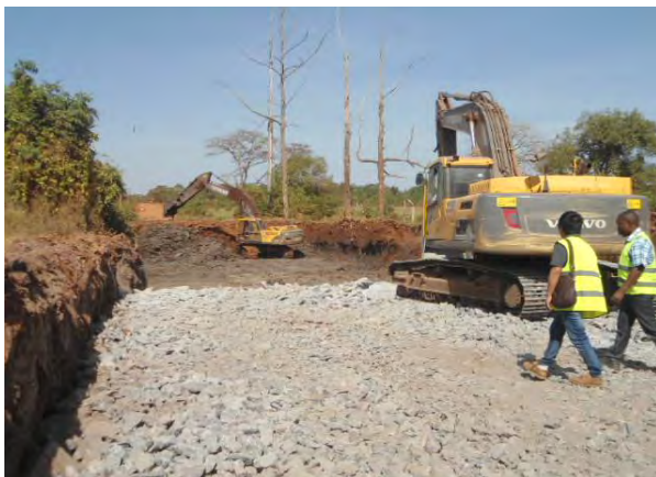
Swamp filling on one of the Kamuli town roads
