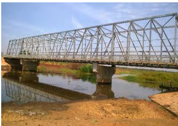
Finished deck for Kabaale bridge, Kyankwanzi district
