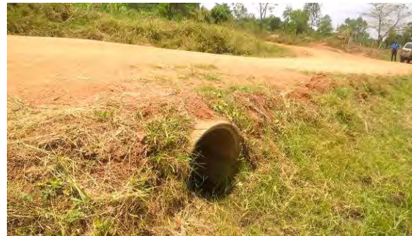
An old culvert installed in the previous years but without head walls
