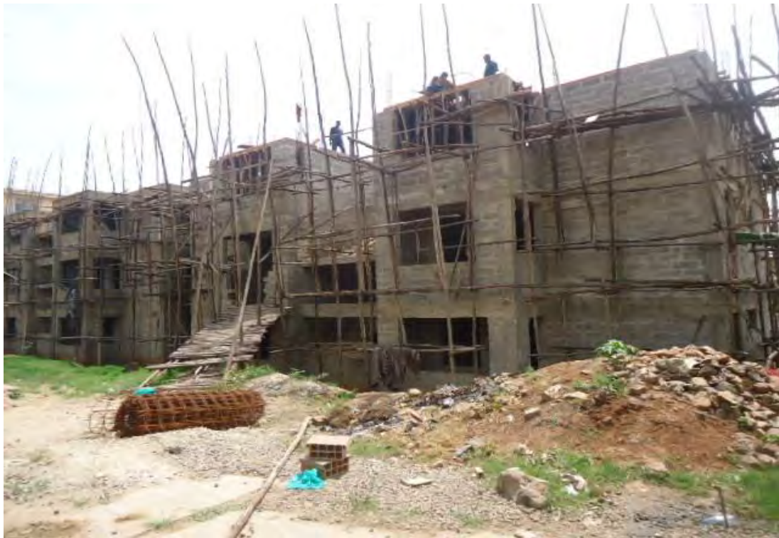
On-going construction works for staff houses at Mbarara RRH
