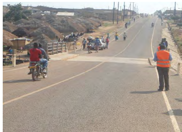
A completed section of Ali-Keny Road in Koboko town
