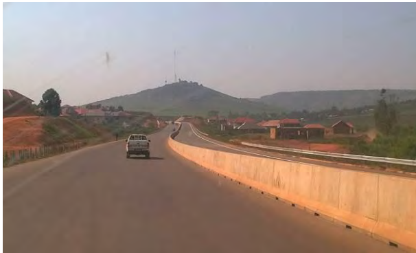
A completed section of the Kampala – Entebbe Expressway awaiting road marking
