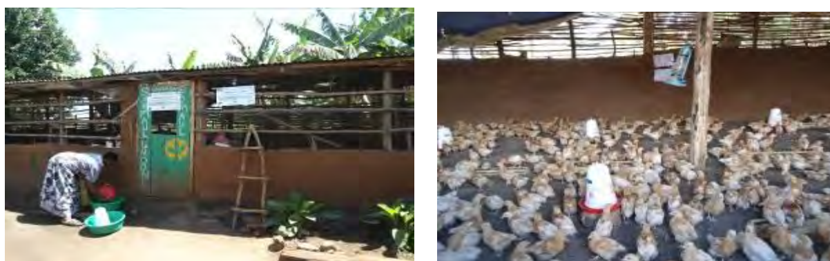
Poultry house constructed and stocked with chicks using the Saemaul Undong Korean model in Kiwumu A village, Kamengo sub-county, Mpigi district
