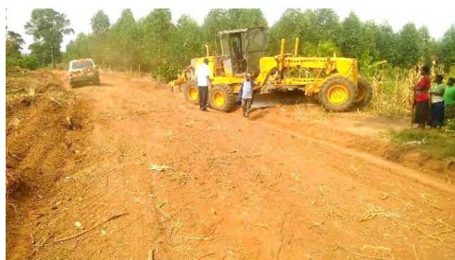
Grading works ongoing along RusandaraRwensambya-Muntabu-Kitoma
