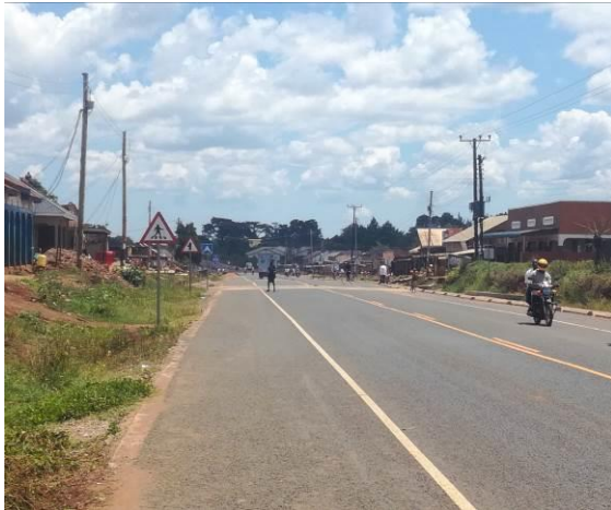
A completed section along the Musita-Lumino/Busia-Majanji Road
