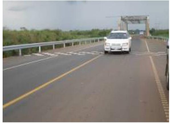
Completed road at Sezibwa river along Mukono-Kayunga Road
