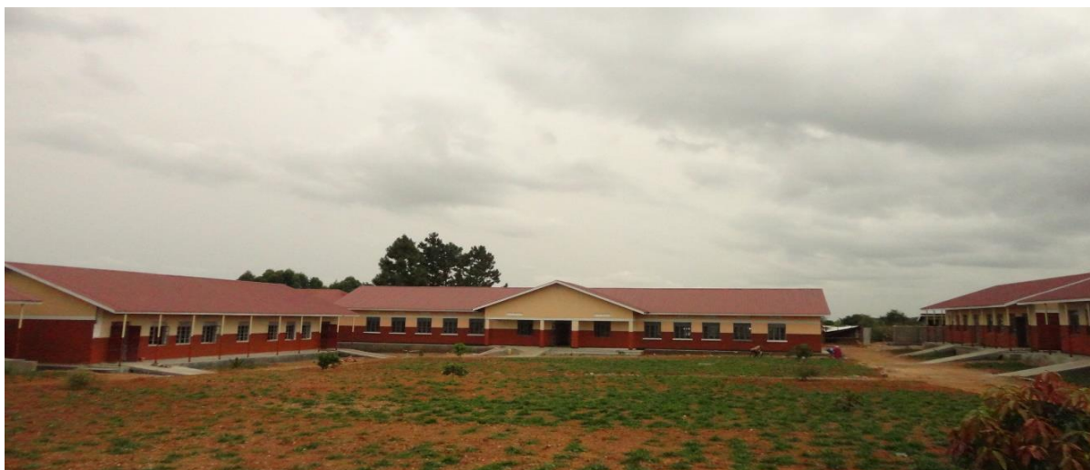
Completed construction of Lukaya Seed School under UgIFT in Lukaya Town Council, Kalungu District
