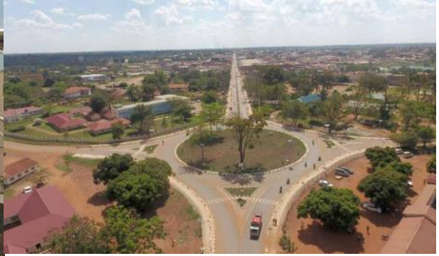
Completed road works on Obote Avenue in Lira City
