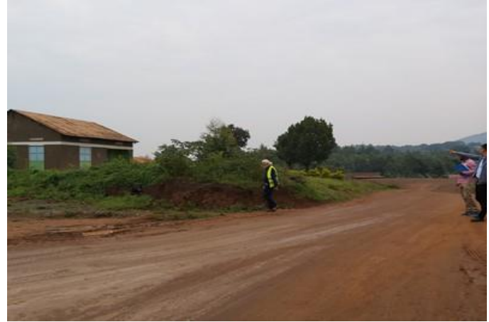
A section (at km16+00) of Bumbobi–Lwakhakha Road skipped due to compensation issues
