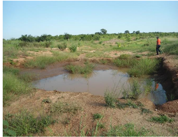
Non-operational Lojudongu community dam (left) and silted small dam in Lojudongu Village, Nebbi District
