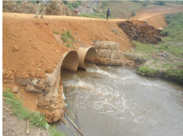
A raised swamp with culverts installed along the graveled Nyakibobo-Buhanama-Rwentojo (12km) Road in Ntungamo District
