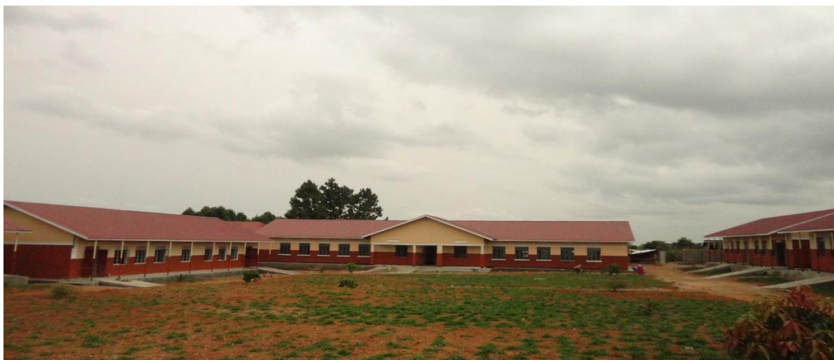
Completed construction of Lukaya Seed School under UgIFT in Lukaya Town Council, Kalungu District
