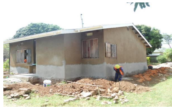
Replacement of asbestos sheets on the principal's house completed (left), and renovation and replacement of asbestos sheets on one of the tutors' house at Bukedi PTC (right)
