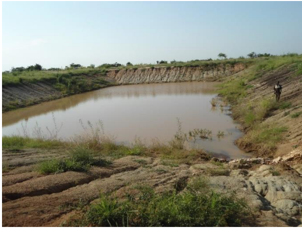
Non-operational Lojudongu community dam (left) and silted small dam in Lojudongu Village, Nebbi District
