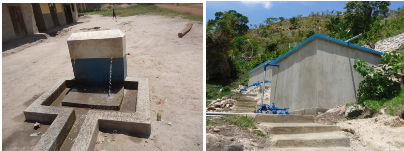
L-R: A tap stand; collection tank and clear water tank in Ngugo Multipurpose Scheme in Ntungamo district
