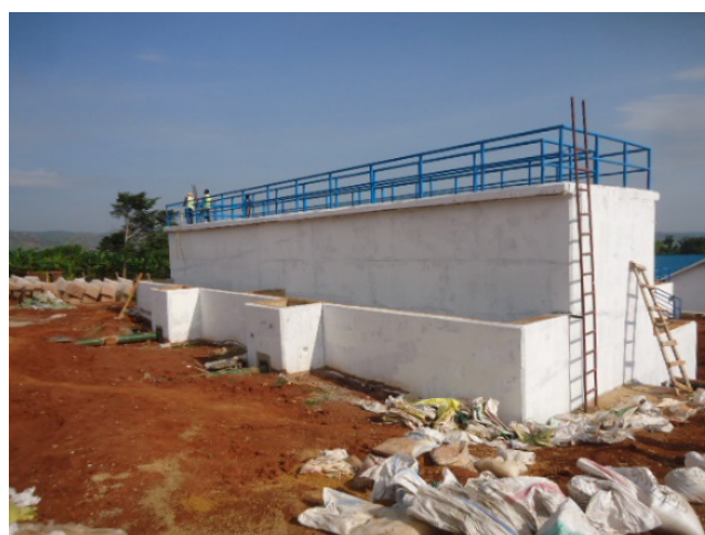
L-R: Sedimentation tank; Filtration tank of the Kapeeka WSS, Kapeeka Sub-county Nakaseke District
