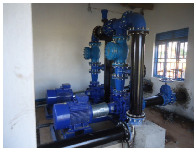
L-R: Weir/low head dam at R. Mayanja; Raw Water Pumps for the Kapeeka WSS, Kapeeka Sub-county, Nakaseke District
