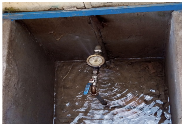
Leakage at the meter
