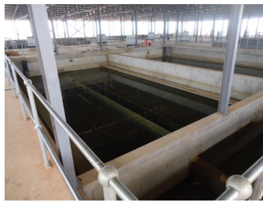
L-R: Sedimentation tanks; Filtration tanks of the Katosi Water Treatment Plant in Mukono District
