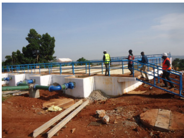
L-R: Sedimentation tank; Filtration tank of the Kapeeka WSS, Kapeeka Sub-county Nakaseke District
