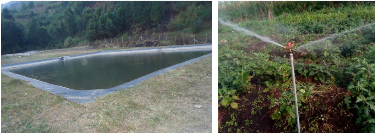
L-R: The 700m 3 reservoir tank in Kazingo Village, Rwengaju Irrigation Scheme and an egg plants' garden in Bukuku Sub-county, Kabarole District
