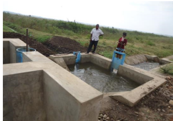
L-R: Ongoing sheltering of the gate valves in Tochi Irrigation Scheme, Oyam District and a Division Box and Gate Valves for both Secondary and Tertiary Canals at Mubuku Irrigation Scheme in Kasese District
