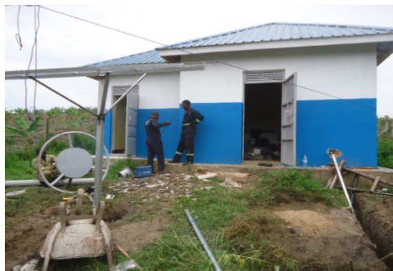
Electro mechanical installation at the pump house
