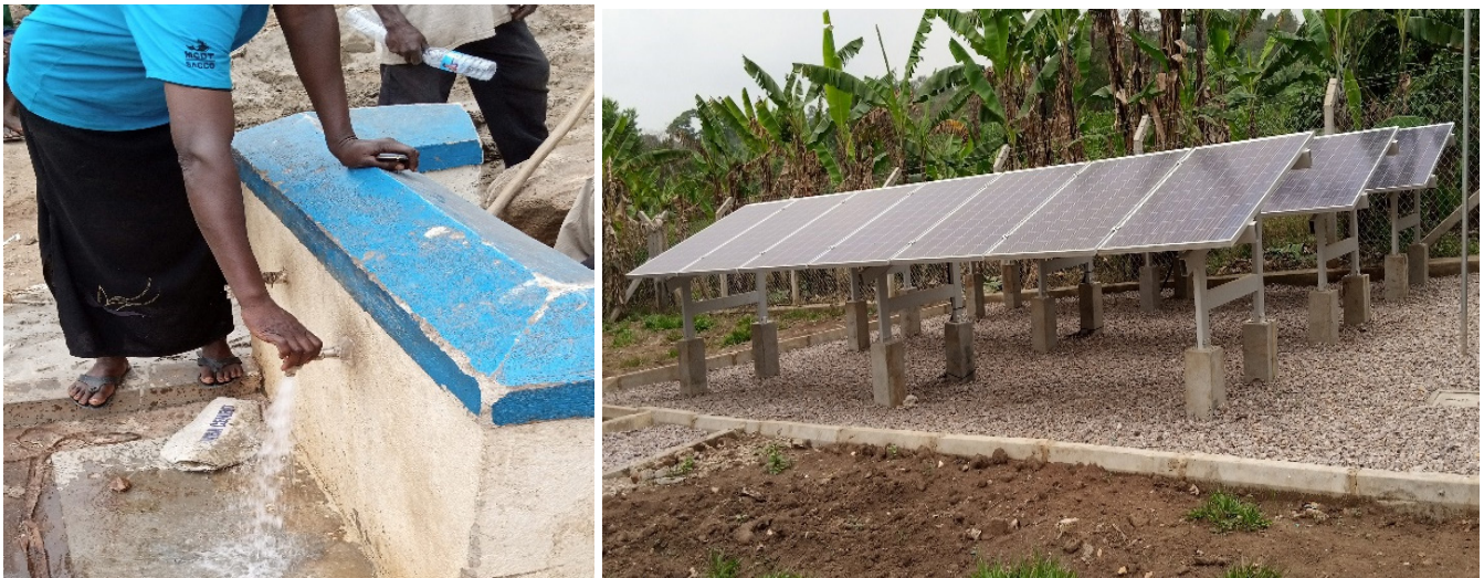
L-R: PSP and solar panels for Sembwa Solar Mini Piped System in Nakaseke Sub-county, Nakaseke District
