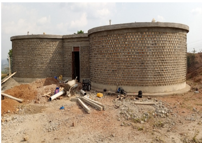
L-R: 100m 3 Twin waters tanks and water pumps in Lwemiyaga RGC Piped Water Supply and Sanitation Scheme Lwemiyaga Sub-county, Lwemiyaga District
