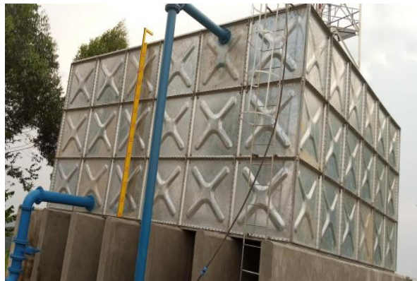
L-R: A six stance Toilet at the market and a steel tank of 200m 3 on dwarf walls in Kigishu village, Kasambya Town Council
