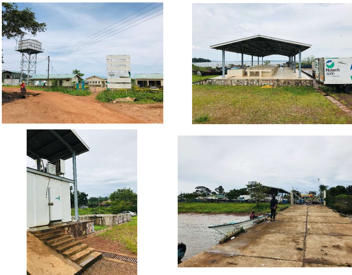
Figure 9: pictures of the facilities at Mwena landing site. Top left: Site entrance showing the water tower, office and security blocks. Top right: processing area. Bottom left: ice machine and ice storage. Bottom right: jetty and access gate to the site.
