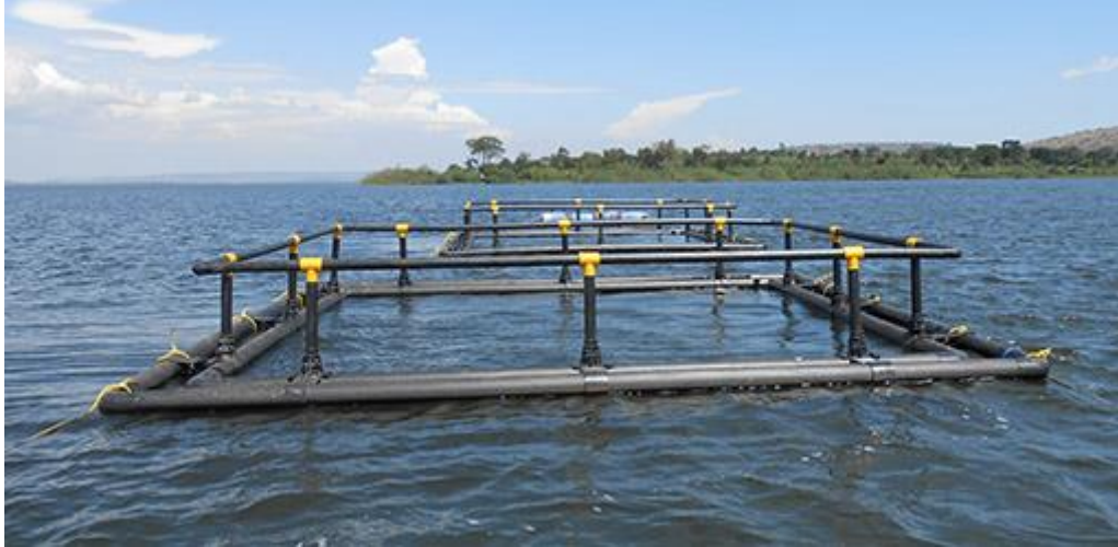
Figure 6; Square HDPE cages which can be operated in the open waters with depth higher than 6 to 8m
